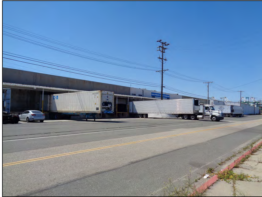
Figure 19: Cannery Block, east elevation with loading dock, showing center of elevation, camera facing northwest. ICF, 2019.
