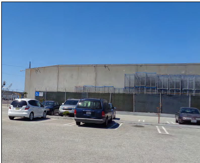
Figure 22: Cannery Block, south elevation, showing western corner of elevation, camera facing north. ICF, 2019.
