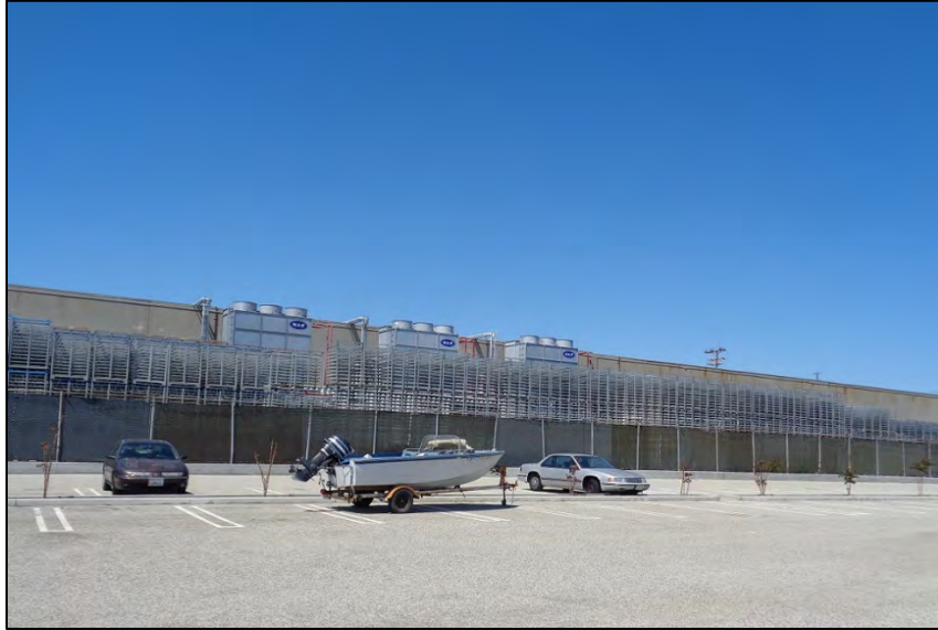
Figure 23: Cannery Block, south elevation, center of elevation obscured by storage, camera facing north. ICF, 2019.
