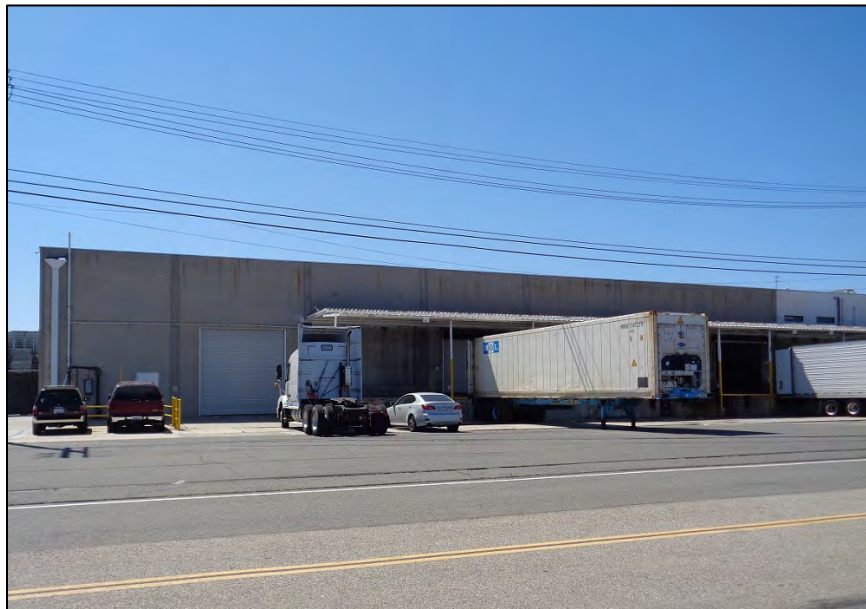
Figure 18: Cannery Block, east elevation with loading dock, showing southern corner of elevation, camera facing west. ICF, 2019.
