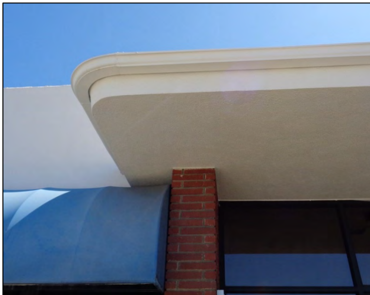
Figure 16: Cannery Block, north elevation, detail showing office building with curved cantilevered porch hood, camera facing west. ICF, 2019.
