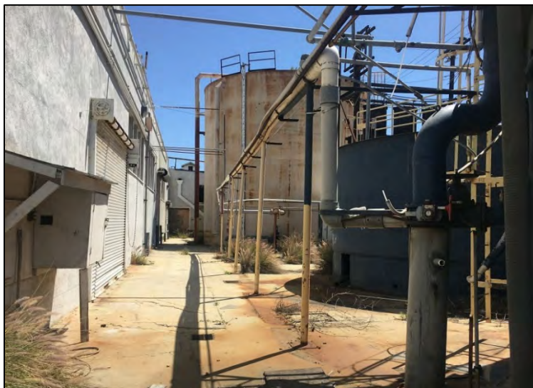
Figure 2: Cannery Block, pipes, tanks, and infrastructure elements, located at the northwest portion of block between a fence at Ways Street and a warehouse (shown on left), camera facing south. ICF, 2019.
