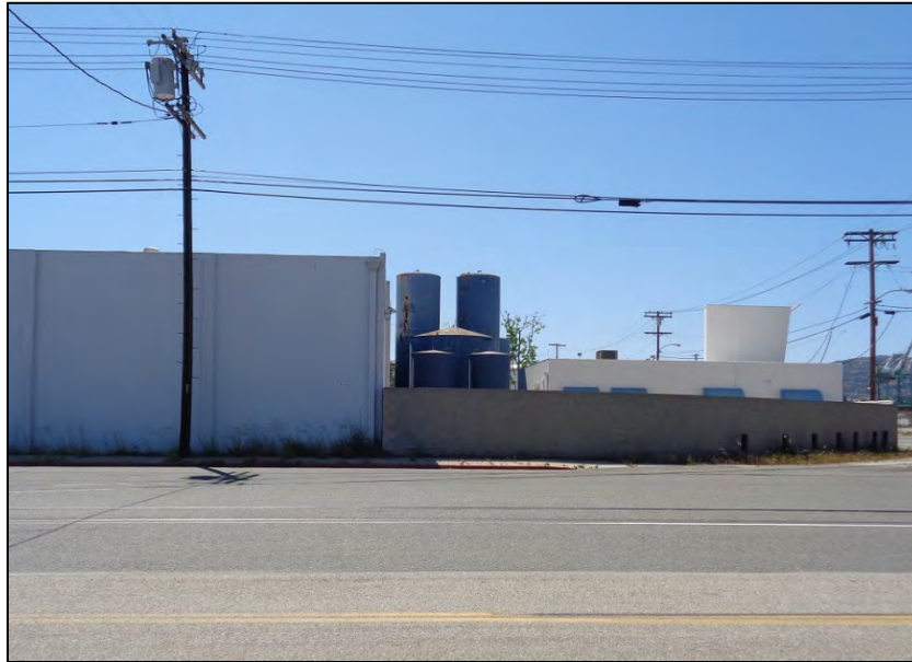
Figure 21: Cannery Block, east elevation with loading dock, showing northern corner, camera facing west. ICF, 2019.
