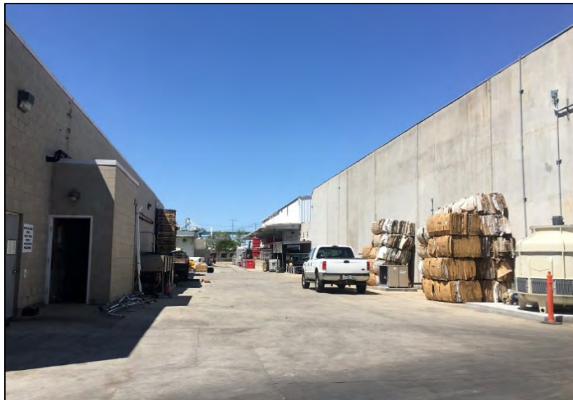
Figure 6: Cannery Block, driveway at an east-west axis, located in the southern portion of the block, camera facing west. ICF, 2019.
