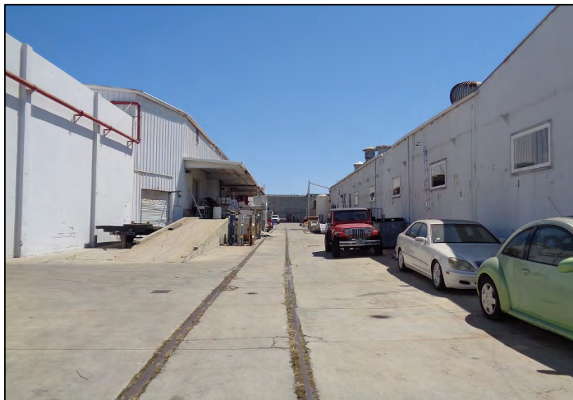
Figure 5: Cannery Block, driveway at a north-south axis, running south from open courtyard between two sets of warehouse buildings, camera facing south. ICF, 2019.
