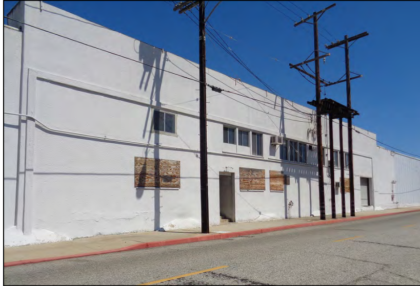
Figure 9: Cannery Block, west elevation, detail showing a middle portion of the elevation with Moderne-esque features, camera facing southeast. ICF, 2019.
