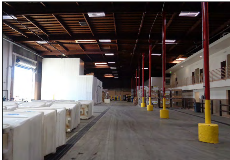
Figure 30: Cannery Block, 1972 warehouse interior, southeast portion of Cannery Block, camera facing north. ICF, 2019.
