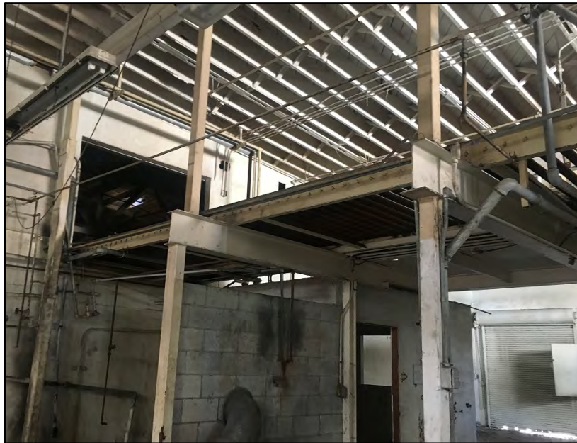
Figure 26: Cannery Block, 1951 warehouse interior, centered between Cannery Street and Sardine Street, just east of Ways Street, camera facing southwest. ICF, 2019.
