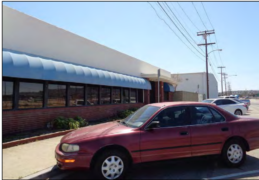
Figure 14: Cannery Block, north elevation, detail showing office building in foreground and warehouse in the background, camera facing west. ICF, 2019.
