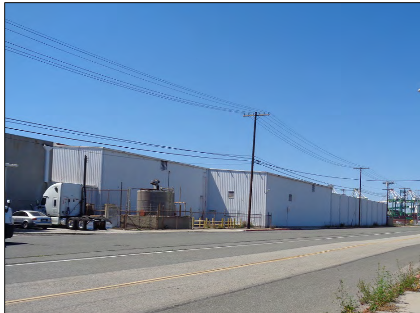
Figure 20: Cannery Block, east elevation with warehouses, showing northern portion of elevation, camera facing northwest. ICF, 2019.
