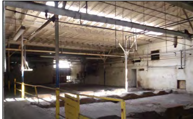
Figure 39: Concrete retort racks. ICF, 2019.
