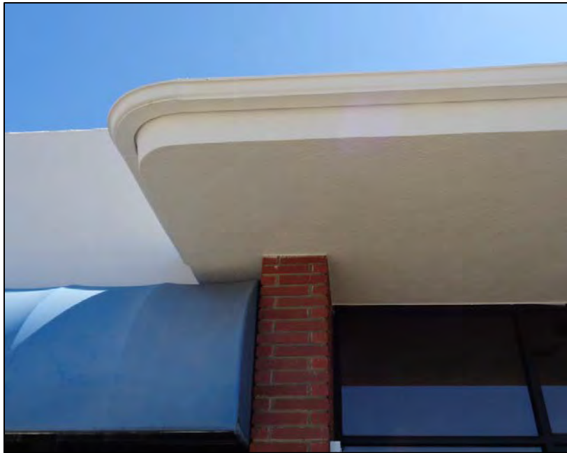
Figure 16: Cannery Block, north elevation, detail showing office building with curved cantilevered porch hood, camera facing west. ICF, 2019.
