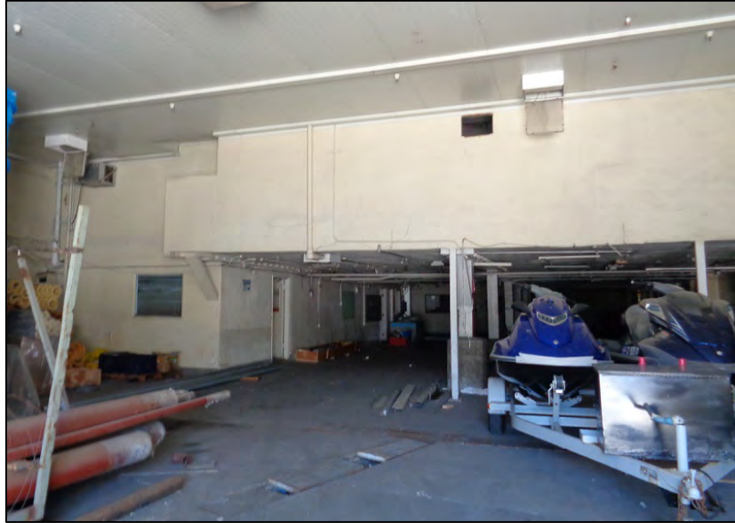
Figure 25: Cannery Block, 1951 warehouse interior, centered between Cannery Street and Sardine Street, just east of Ways Street, camera facing north. ICF, 2019.
