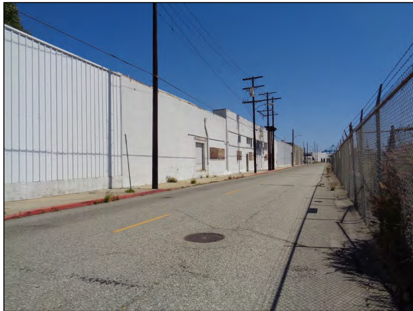
Figure 8: Cannery Block, west elevation, view showing middle of elevation, camera facing south. ICF, 2019.
