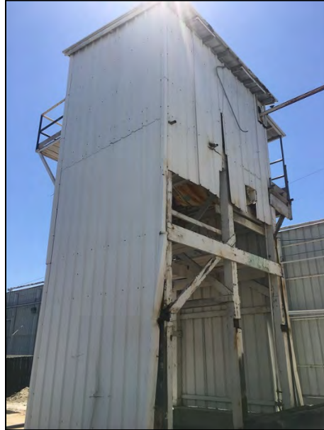
Figure 1: Cannery Block, tuna import tower, located adjacent to Ways Street at western side of block, camera facing west. ICF, 2019.
