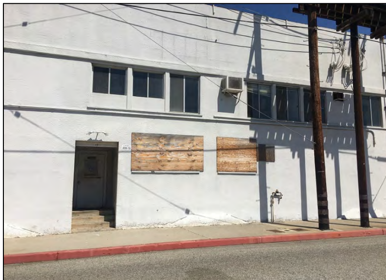
Figure 10: Cannery Block, west elevation, detail showing entrance and windows of the middle portion of the elevation with Moderne-esque features, camera facing east. ICF, 2019.
