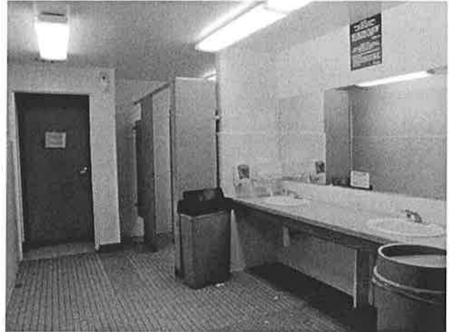
Matching funds from Los Angeles County went towards various ADA improvements, including upgrading existing restrooms.
