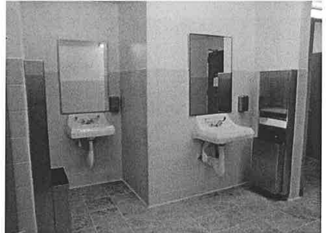
New ADA-upgraded restrooms include new sinks, floors, and accessible stalls.
