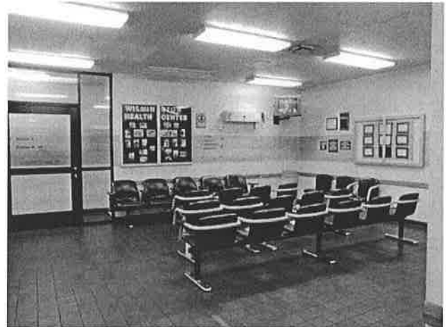
Furniture, flooring, and signage in the lobby had not been updated since the facility was first built in 1970.
