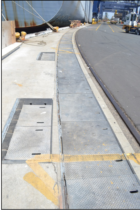
Photograph 1: Existing Landside Crane Rail at Berths 212-216 (100' Gauge)
