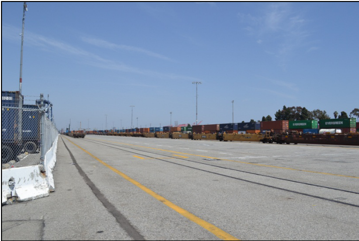
Photograph 1: Existing TICTF On-Dock Rail
