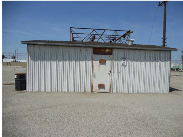
Plate 7. Southern Façade of Structure 2. View to Northwest.
