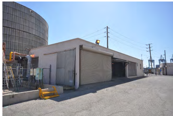
Figure 24: View looking east towards Storage Building 2. (GPA, 2018)
