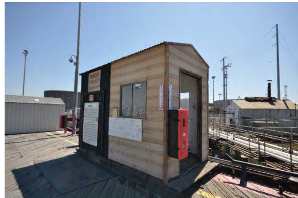
Figure 28: View looking northeast towards Wharf Building 2. (GPA, 2018)
