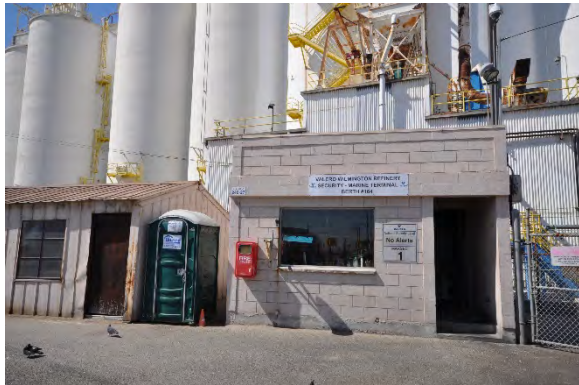
Figure 25: View looking southwest towards Guard Shack 2. (GPA, 2018)
