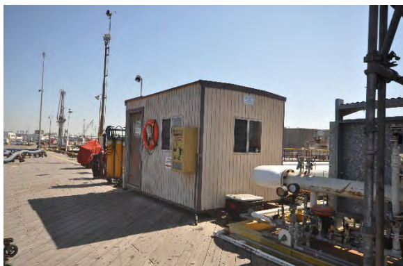
Figure 31: View looking northeast towards Wharf Building 5. (GPA, 2018)
