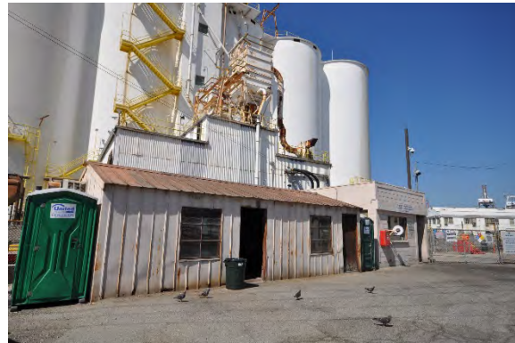
Figure 26: View looking southwest towards Office 5. (GPA, 2018)
