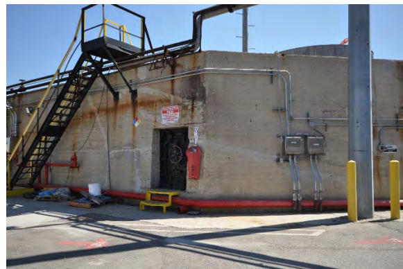
Figure 10: View looking northeast towards Tank Farm 2 dike wall entrance. (GPA, 2018)
