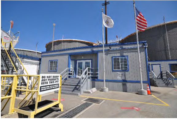
Figure 7: View looking northeast towards Office 1, the larger of the two prefabricated office buildings outside the dike wall. (GPA, 2018)
