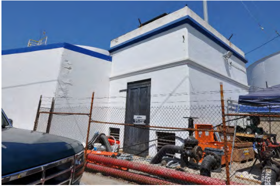
Figure 13: View looking west towards Transformer Building. (GPA, 2018)
