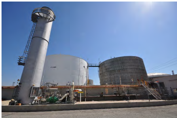
Figure 23: View looking north towards Tank Farm 5, thermal oxidizer at left. (GPA, 2018)
