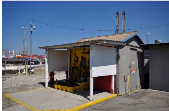
Figure 18: View looking northwest towards the fifth of eight pre-fabricated sheds. Corrugated metal shed. (GPA, 2018)
