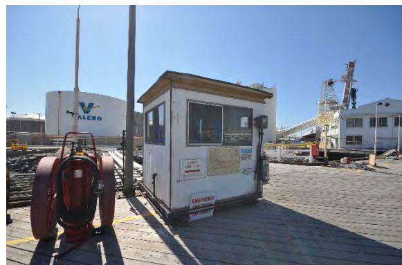
Figure 32: View looking southeast towards Wharf Building 6. (GPA, 2018)
