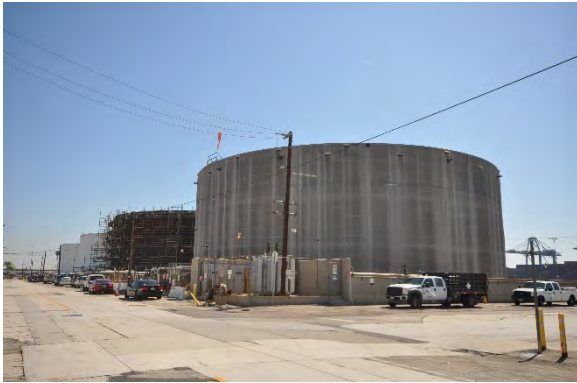
Figure 33: View looking northeast towards Tank Farm 6. (GPA, 2018)
