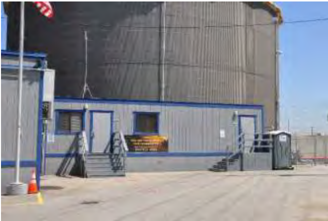
View looking NE towards Office 2, 8/6/2018
