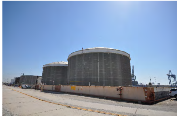
Figure 34: View looking northeast towards Tank Farm 7. (GPA, 2018)
