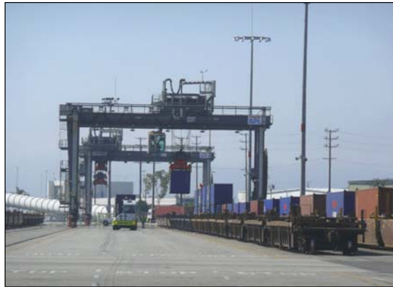
RMG at the existing on-dock railyard
