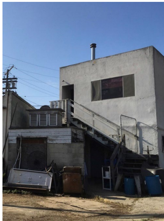
Figure 3: 264 22nd Street, north (rear) elevation, view south. ICF 2023.
