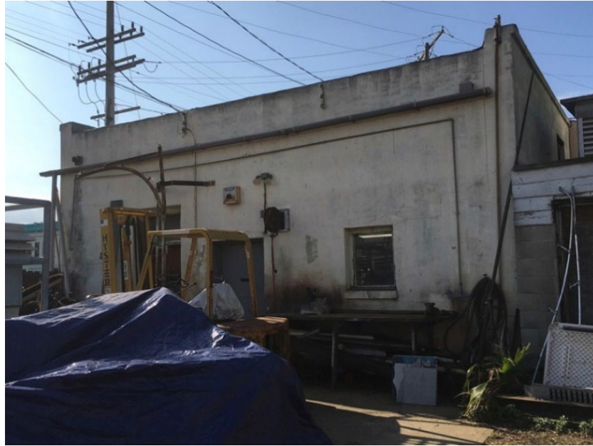
Figure 3: 266–270 22nd Street, north (rear) elevation, view southeast. ICF 2023.
