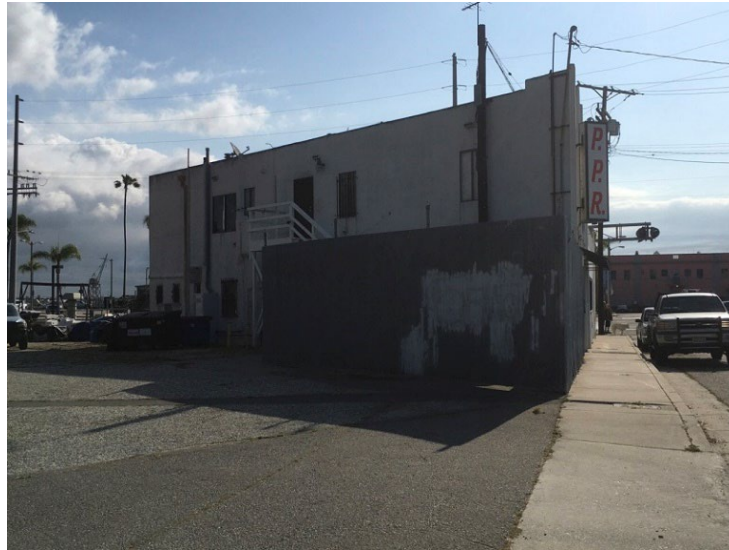
Figure 2: 264 22nd Street, west (side) elevation, view east. ICF 2023.
