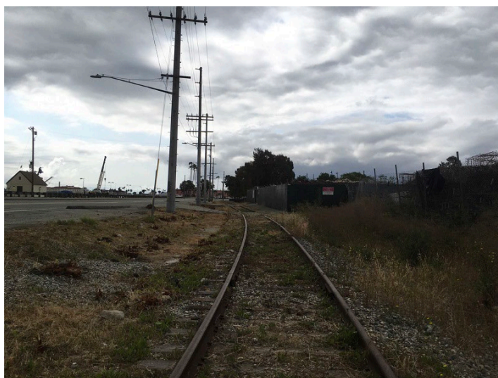
Figure 3: Former SPRR/San Pedro Waterfront Red Car Line, Port of Los Angeles, track located in the eastern section of the study area showing one spur line near Harbor Boulevard, view south (ICF 2023).
