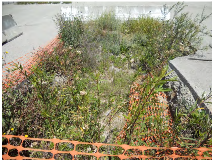
Plate 3. Open Trench at Southwest Corner of Project Site. View to Northeast.
