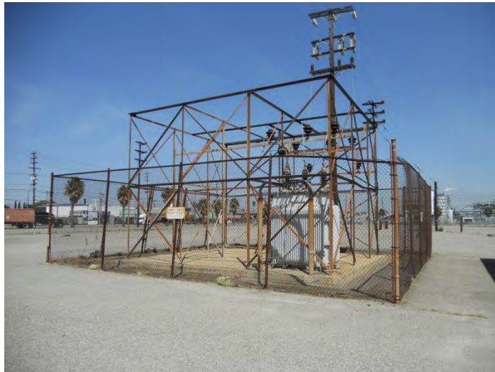
Plate 6. Structure 1 Enclosed by Fencing. View to Northeast.
