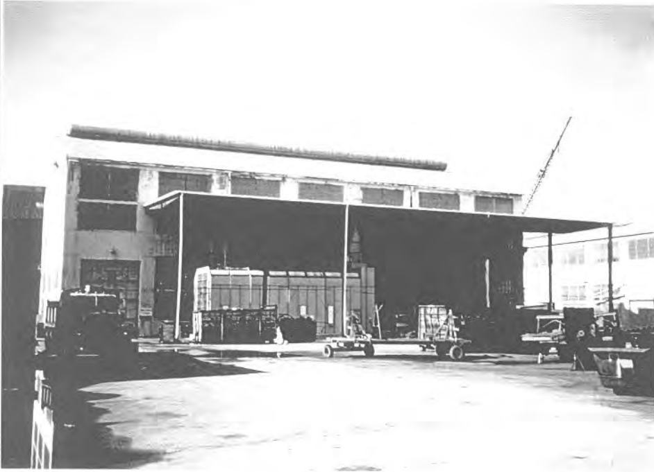
Photograph 2. Metal shelter at rear of building
