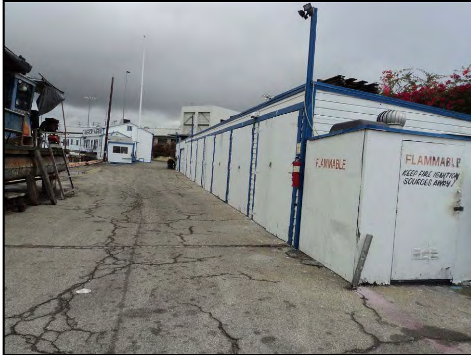
Photograph 34. Overview of Garage 12-19 at American Marine Corporation; view to the north
