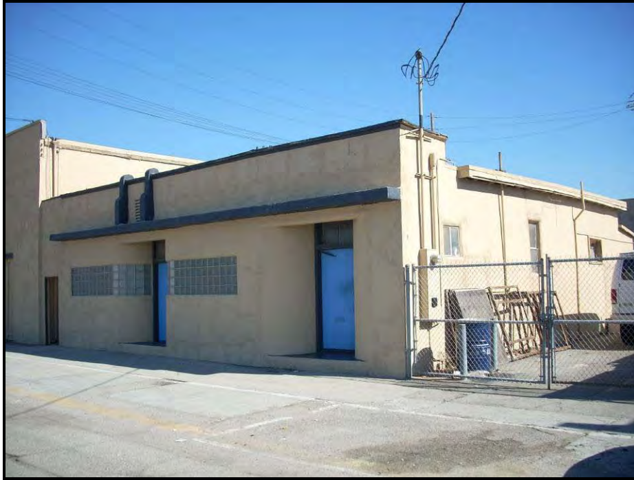
Photograph 19. Overview of 712–716 Tuna Street; view to the northeast
