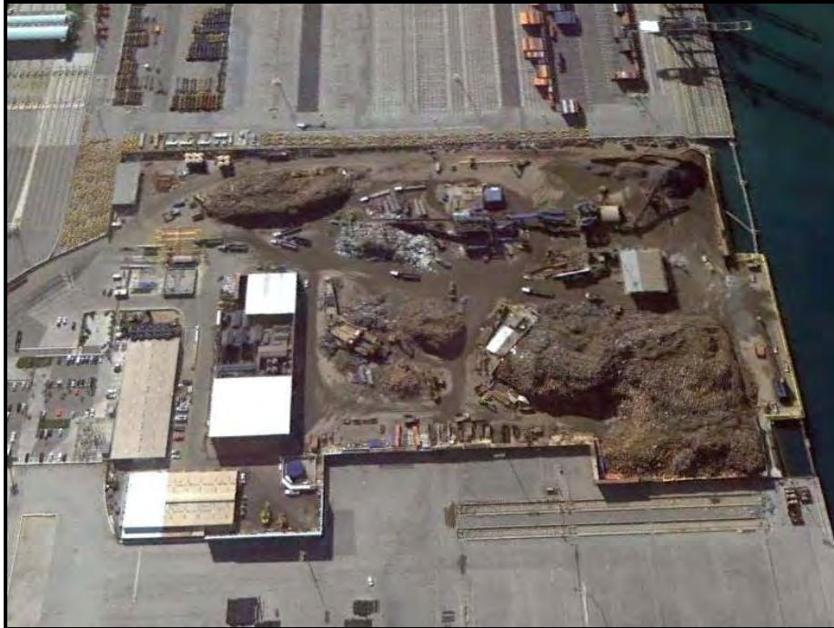
Photograph 4. Overview of SA Recycling; view to the west (Source: Google Earth)
