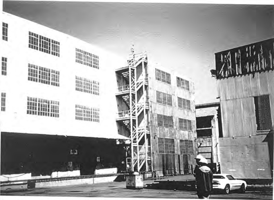
Photograph 2. Exterior metal stairs
