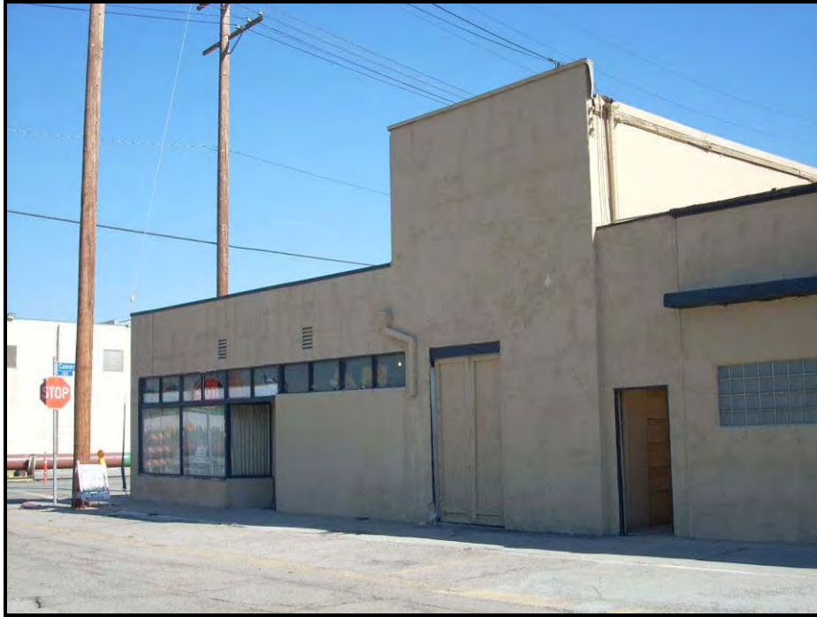
Photograph 17. Overview of 700–702 Tuna Street; view to the northeast
