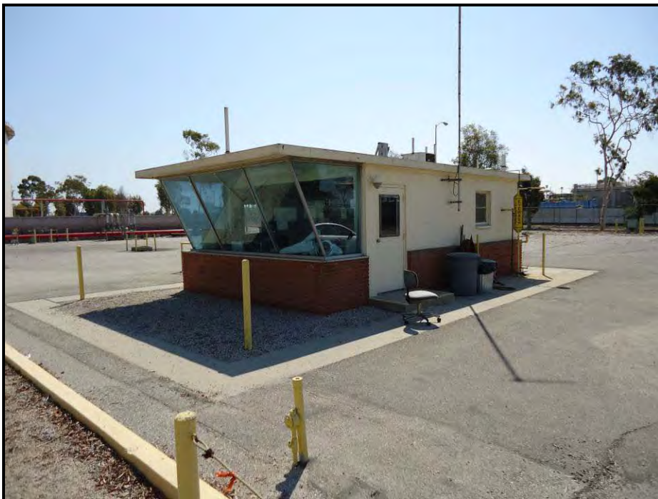
Photograph 11. Operation building at ExxonMobil Tank Farm; view to the southeast
