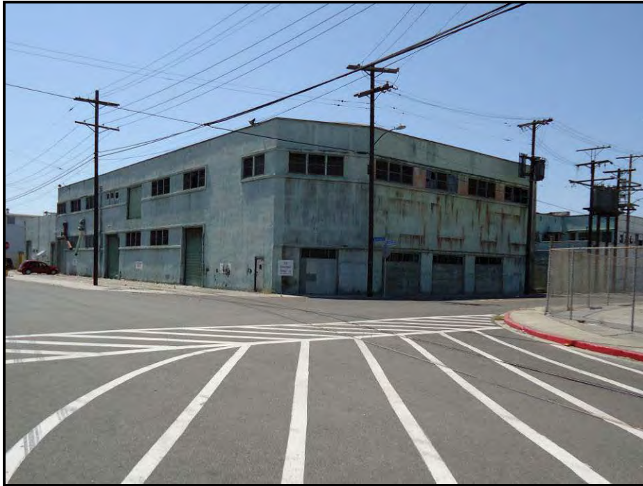
Photograph 27. Overview of can warehouse at Pan Pacific Cannery; view to the southwest.
