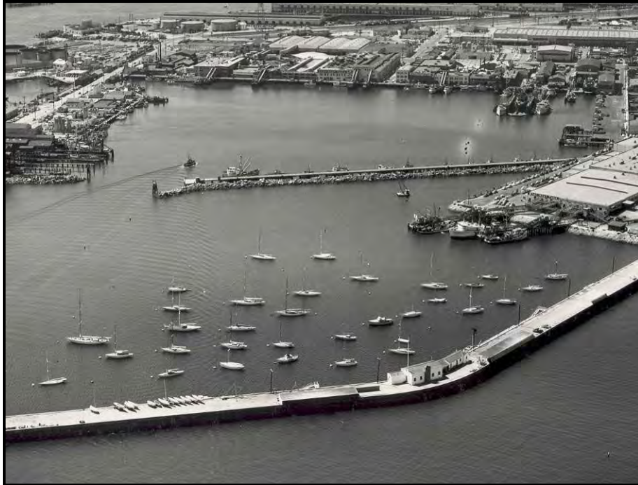
Photograph 36. View of Los Angeles Yacht Club, 1955 (Source: Los Angeles Harbor Department archives)
