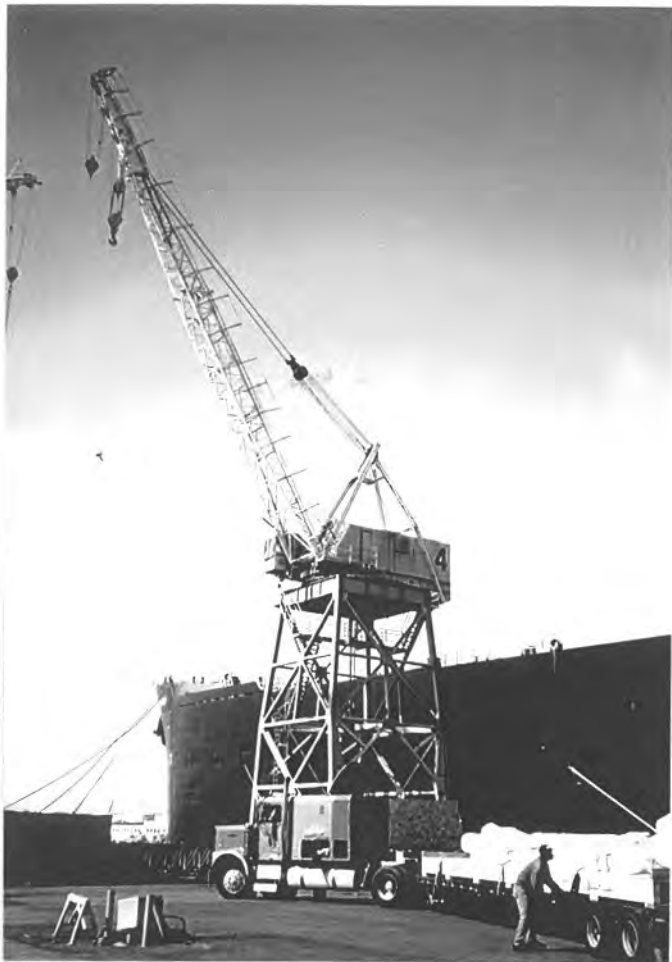
Photograph 1. Colby Crane southeast view
