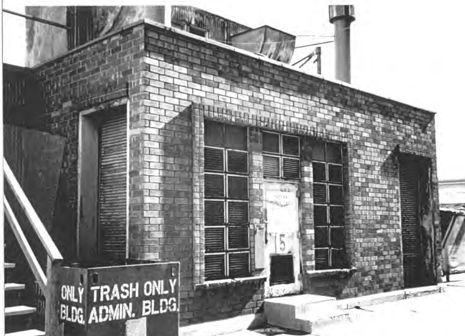
Photograph 2. Substation, southwest elevation
