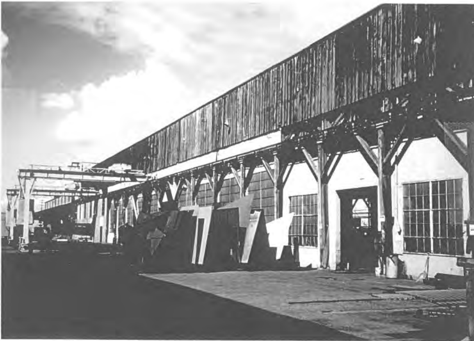
Photograph 2. West elevation showing wood trusses
