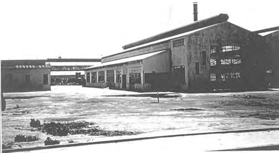
Photograph 2. Shed-roofed, metal-sided extension
