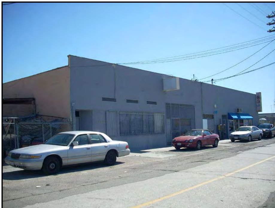
Photograph 21. Overview of northern portion of 742–748 Tuna Street; view to the southeast
