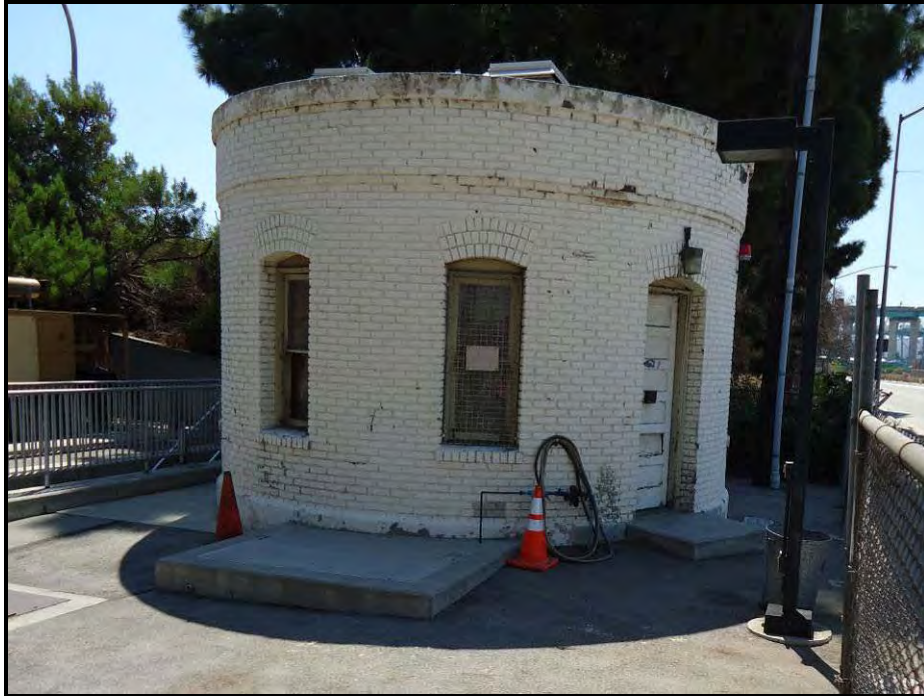
Photograph 6. Overview of Sewage Pump Station #669; view to the west
