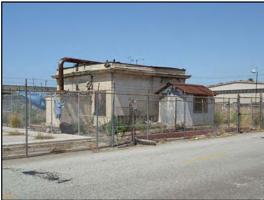
Photograph 16. Overview of Pumphouse on Ways Street; view to the northwest
