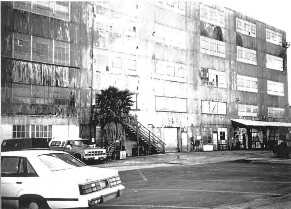
Photograph 3. Replacement windows and metal awning
