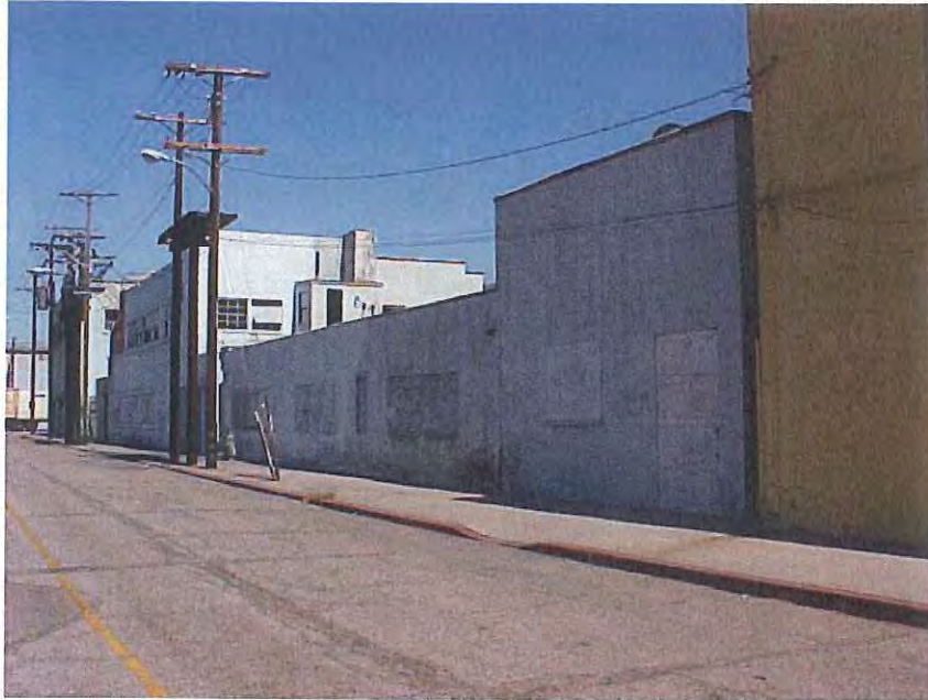
View along Sardine Street, facing southeast, January 2004 Note: former Marine Hardward Building (razed) along right edge
