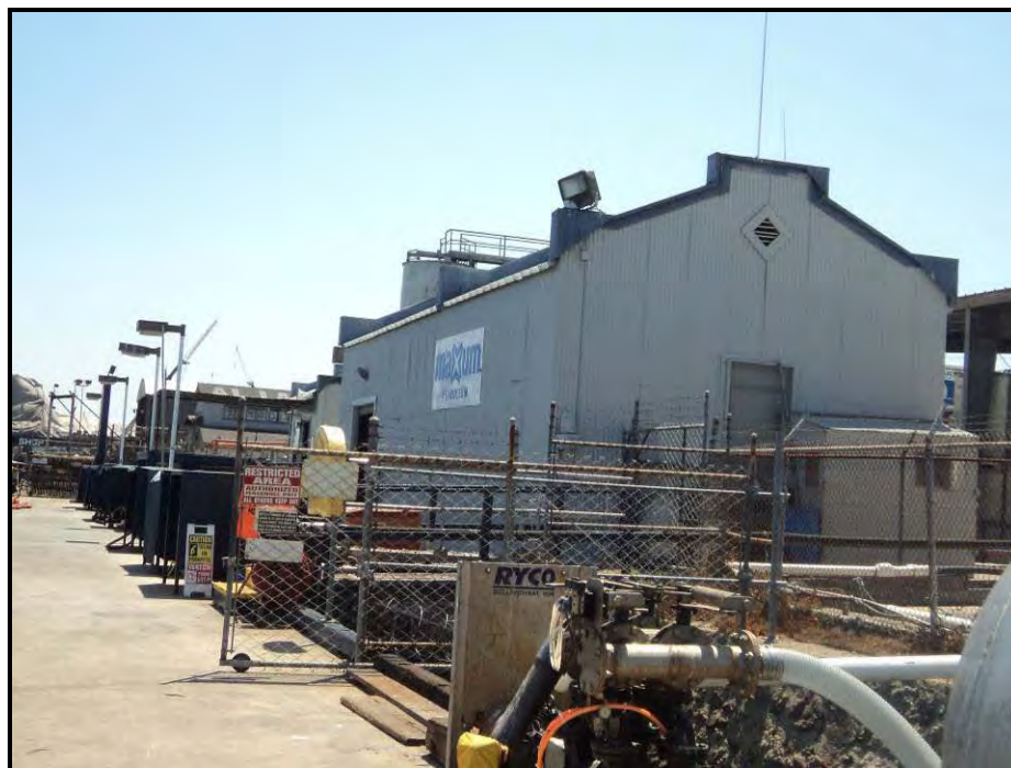
Photograph 31. Warehouse and dock at Maxum Petroleum; view to the south
