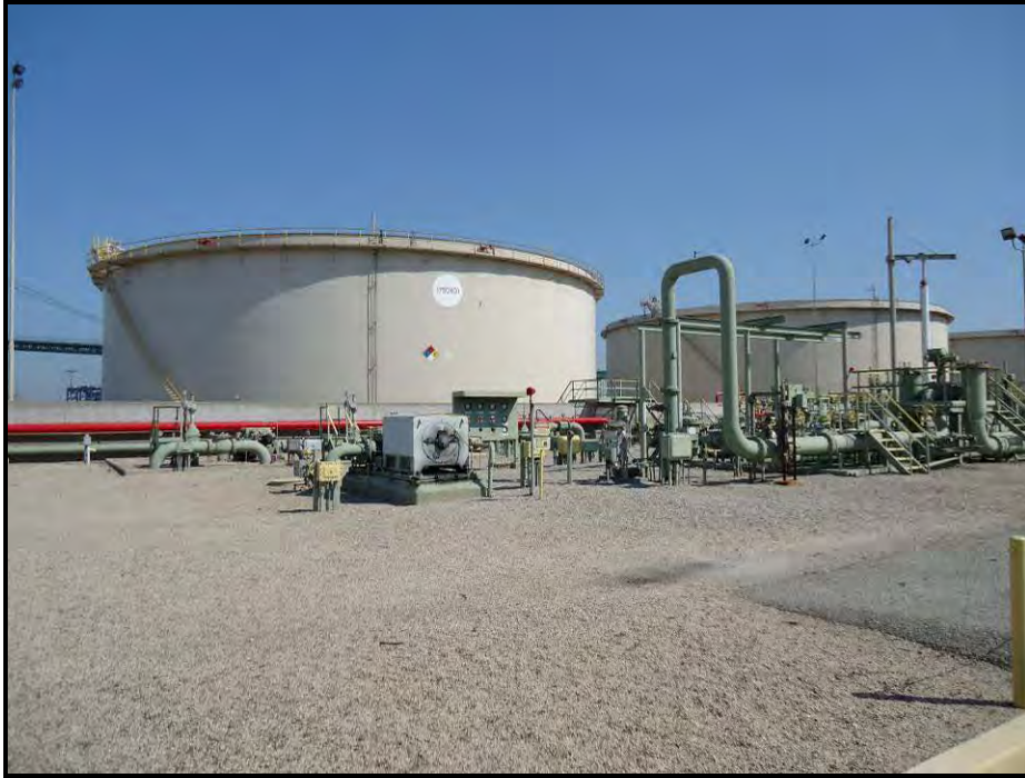
Photograph 10. Overview of ExxonMobil Tank Farm; view to the northeast
