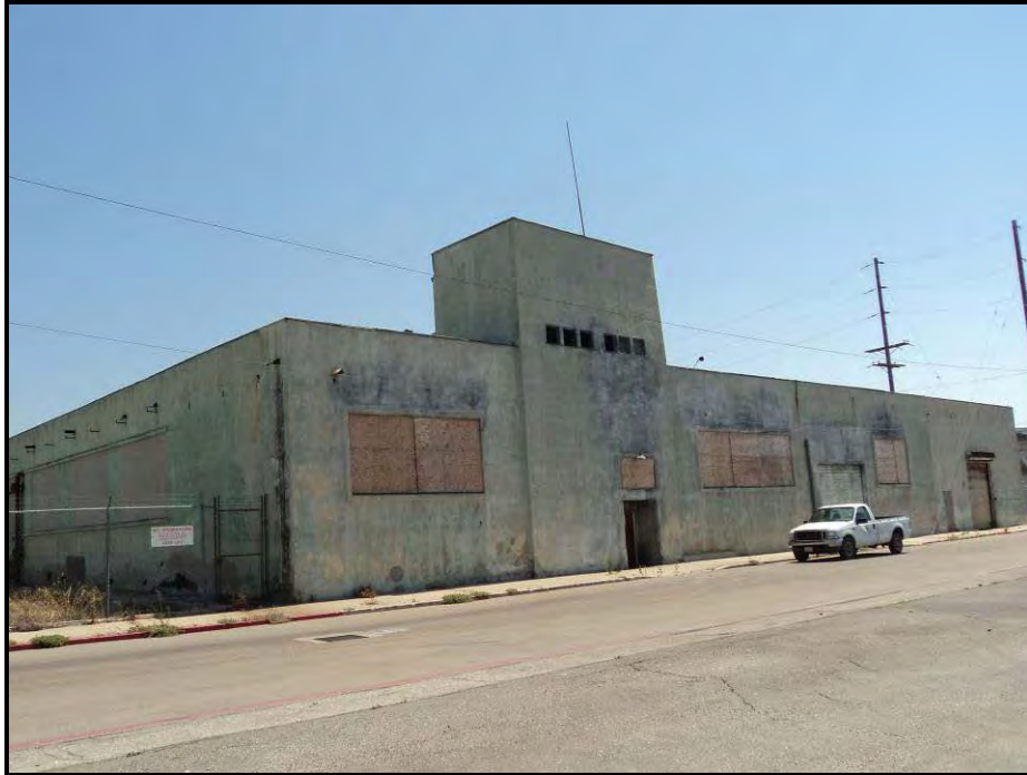
Photograph 29. Main building at Pan Pacific Cannery; view to the southeast
