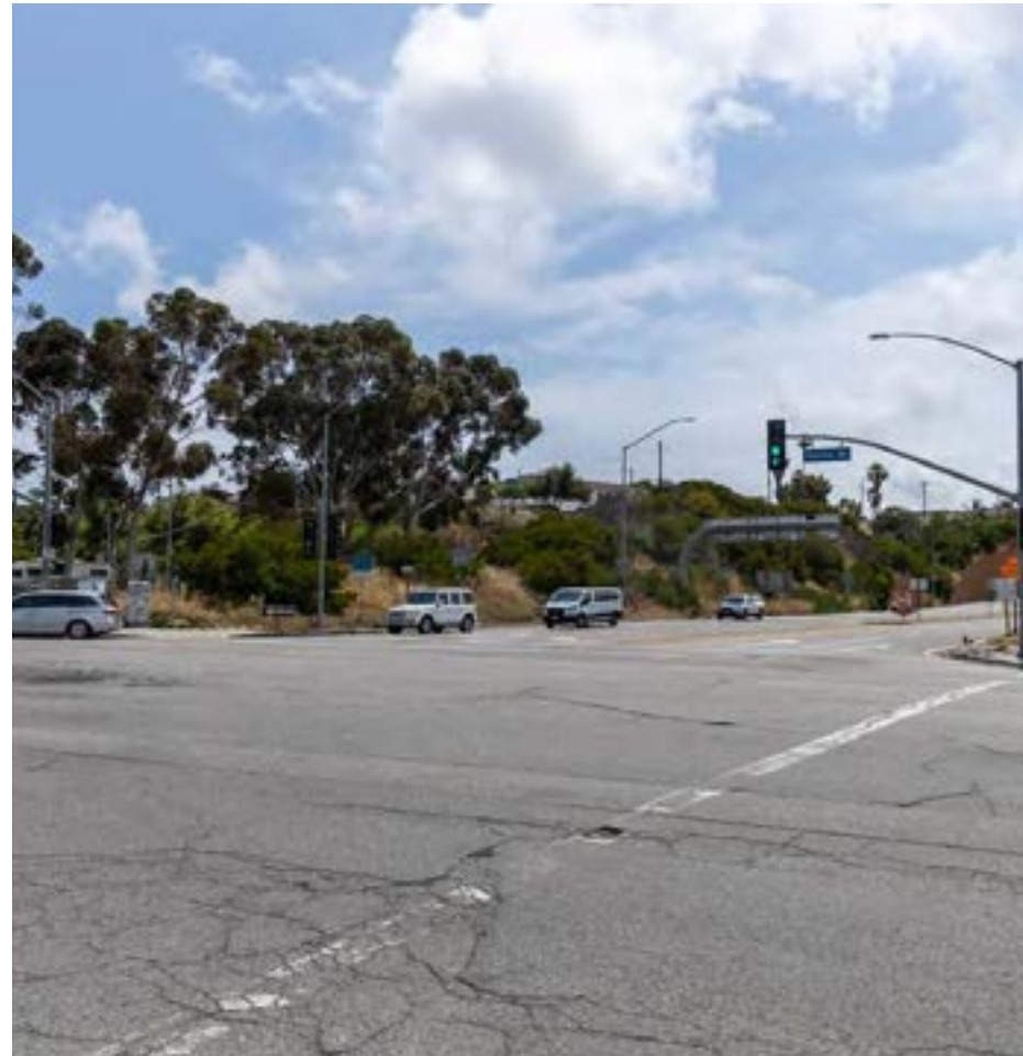
Harbor Boulevard & Swinford Street Freeway Exit
