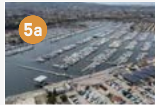
5a Day Use Guest Docks at Cabrillo Harbor: Transient slips that are incorporated into any new landside development at Cabrillo Harbor
