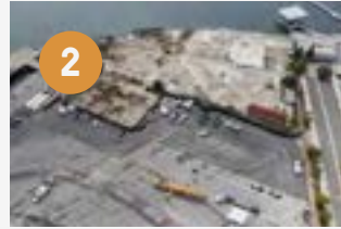
2 Berth 44 Boatyard: Redeveloped boat storage space
