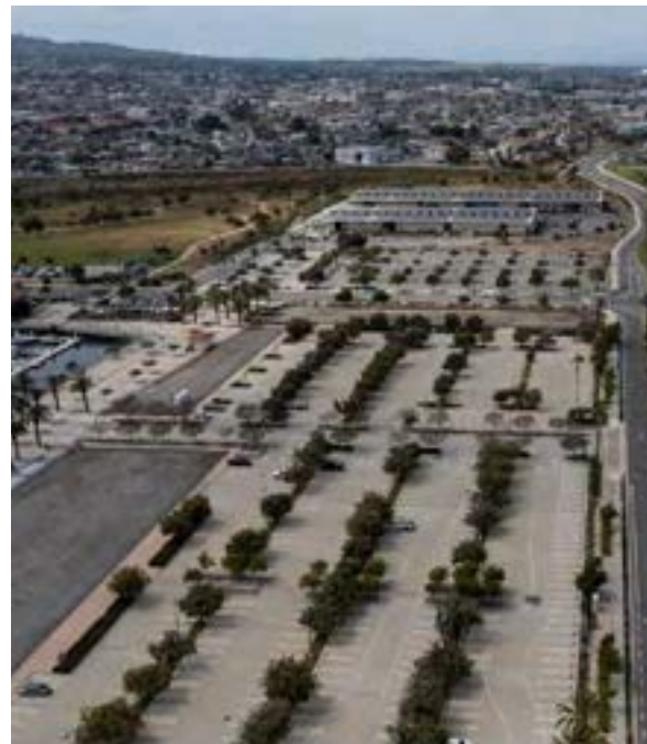
Parking for Cabrillo Way Marina and CRAFTED/Brouwerij West
