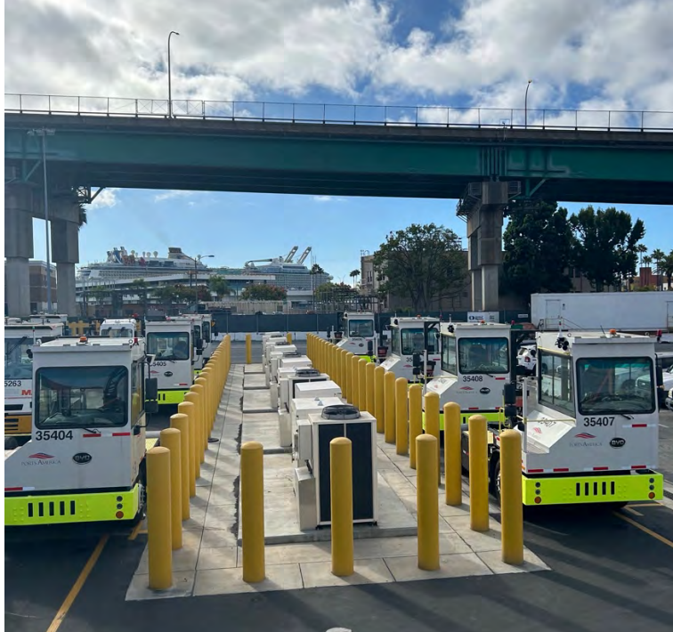
FIGURE 4: Main Equipment Charging Corral with five primary battery cabinets and 10 inductive charging pads. Eight of the battery-electric yard tractors are parked over the pads accepting a charge. This photo is the same as above, but taken from the opposite direction.
