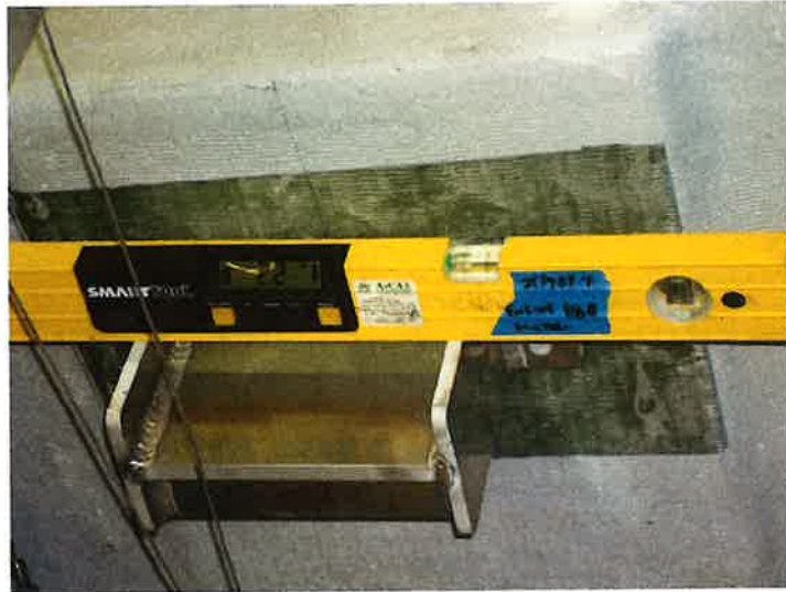
Figure 8: Digital level equipment being used during engine mount installation
