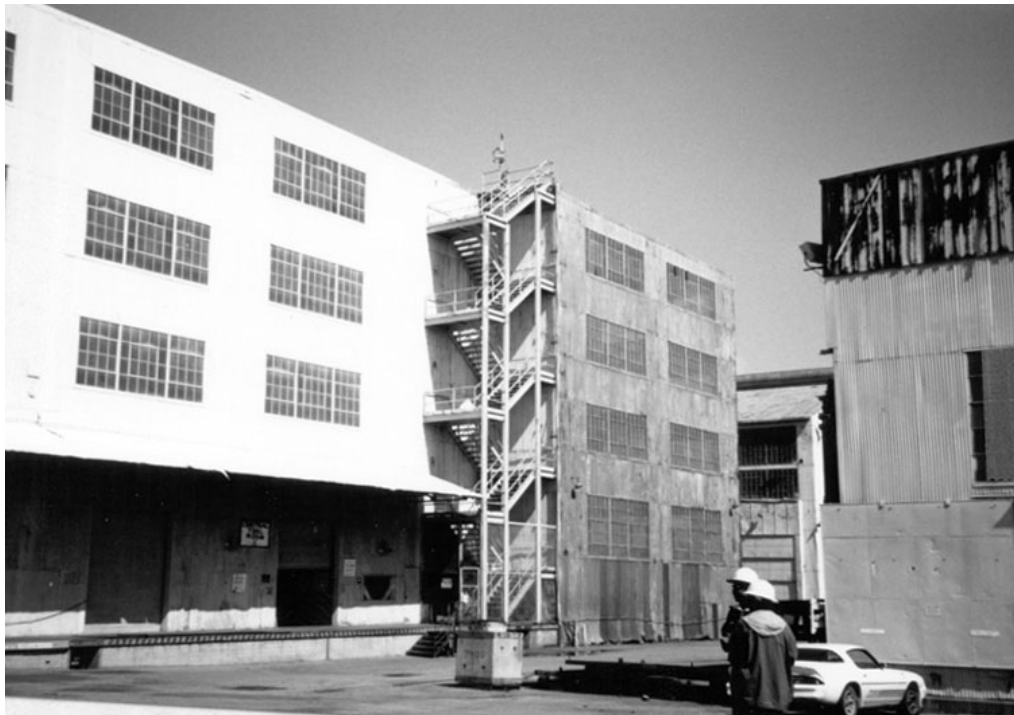
Photograph 2. Exterior metal stairs
