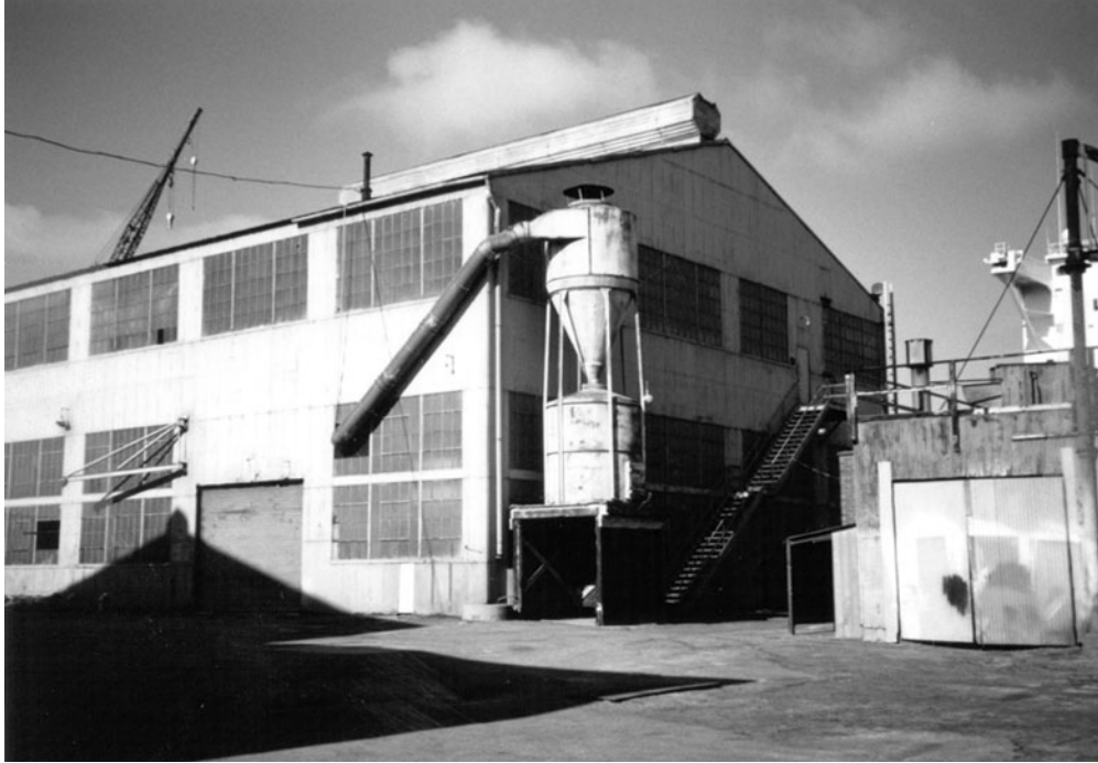
Photograph 2. Sawdust silo at north elevation
