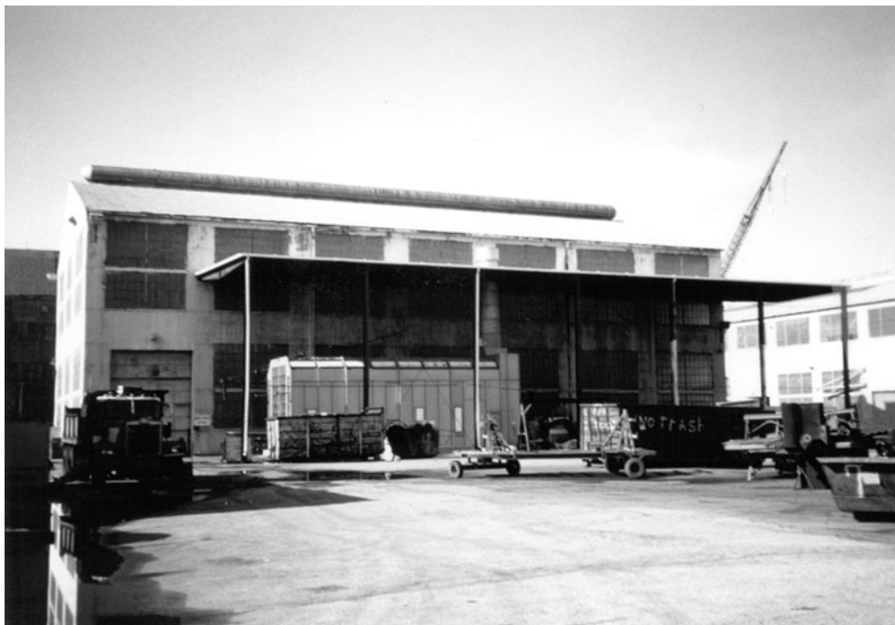
Photograph 2. Metal shelter at rear of building
