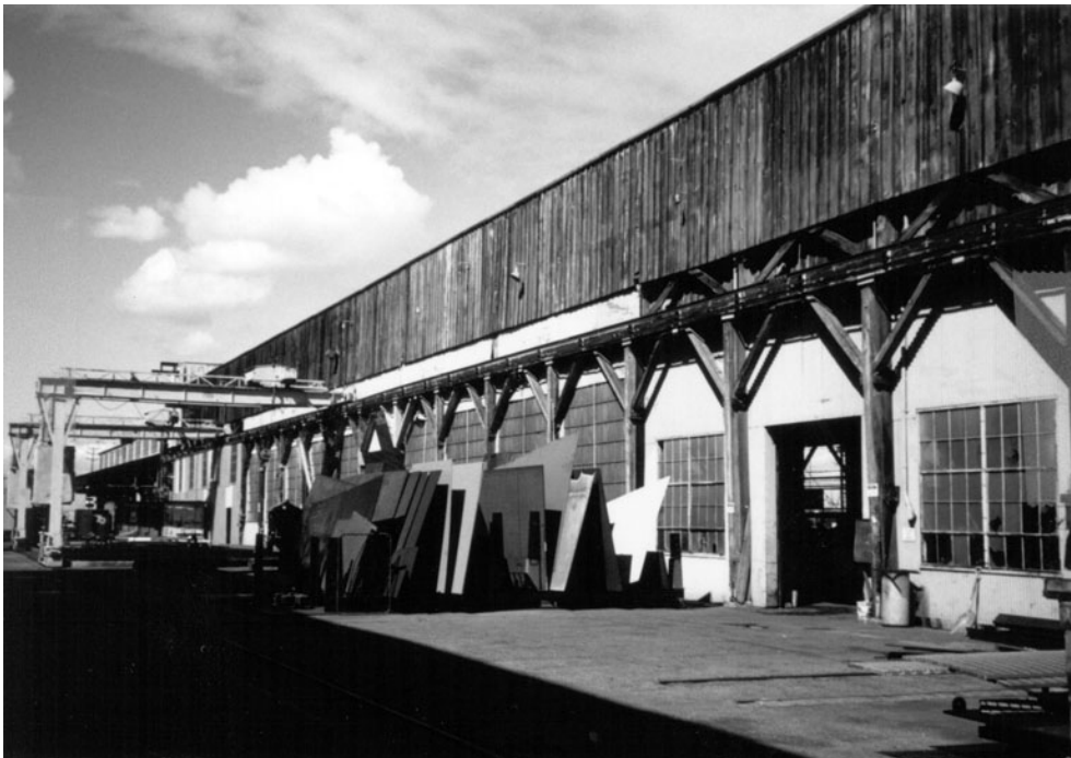
Photograph 2. West elevation showing wood trusses
