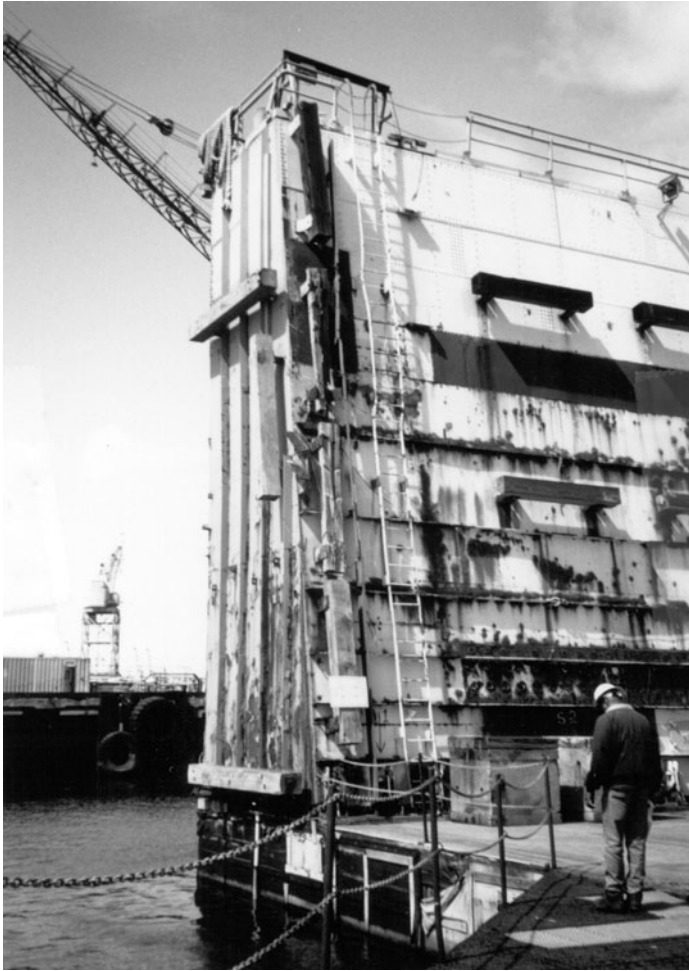
Photograph 2. Front of Dry Dock #1 wing wall, southwest elevation
