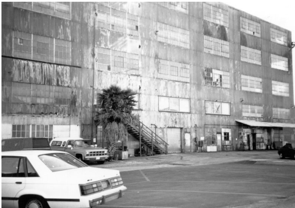
Photograph 3. Replacement windows and metal awning
