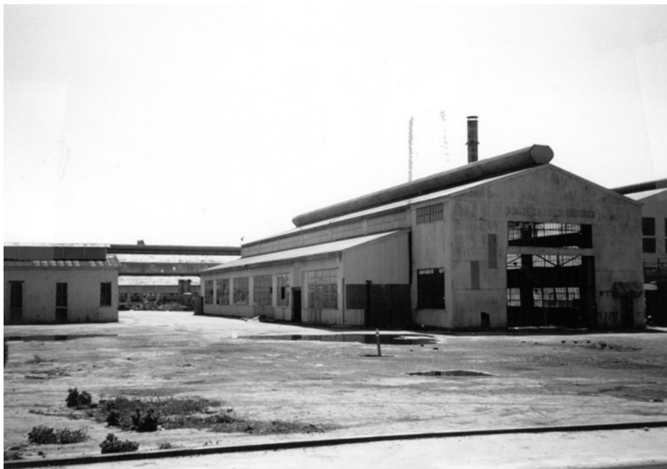
Photograph 2. Shed-roofed, metal-sided extension
