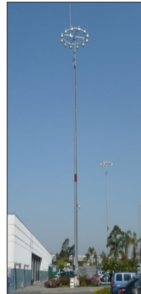
Photograph 8: Example of light poles
