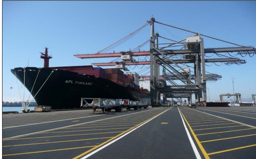
Photograph 1: View of existing wharf, cranes, and berthed vessel
