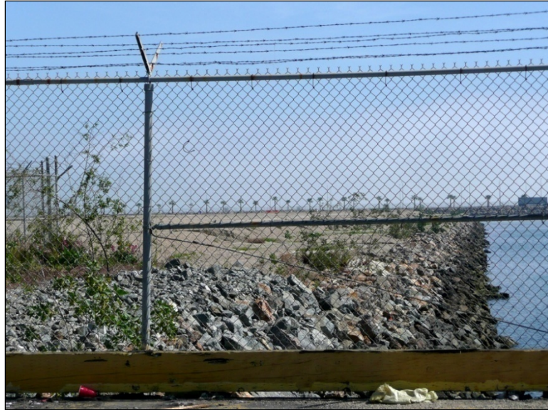
Photograph 2: Area of new wharf along Berth 306
