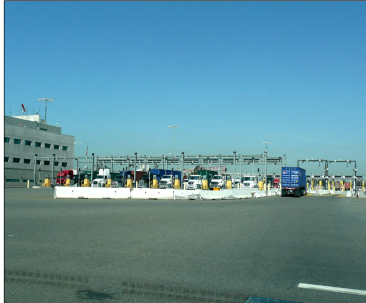
Photograph 7: Existing in-gate and out-gate
