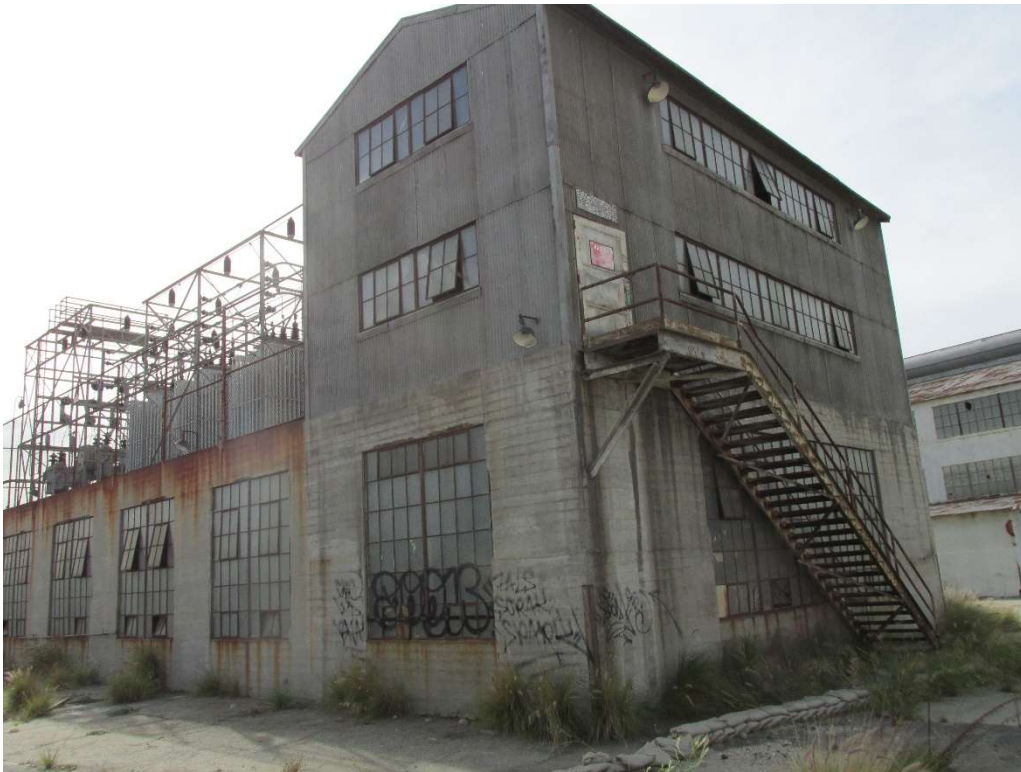
Figure 5. Transportation Shop #4, Northeast Elevation, IMG_9465
