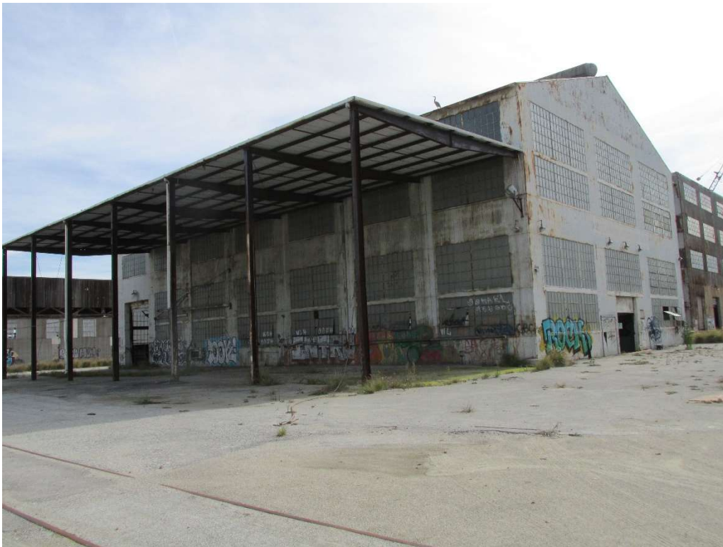
Figure 10. Shop #9, Northwest Elevation, IMG_9410
