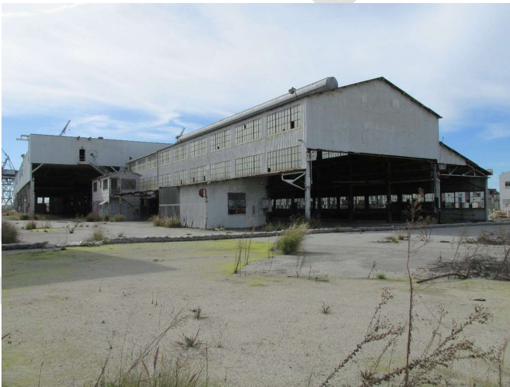
Figure 6. Blacksmith and Anglesmith Shop, Northeast Elevation, IMG_9107
