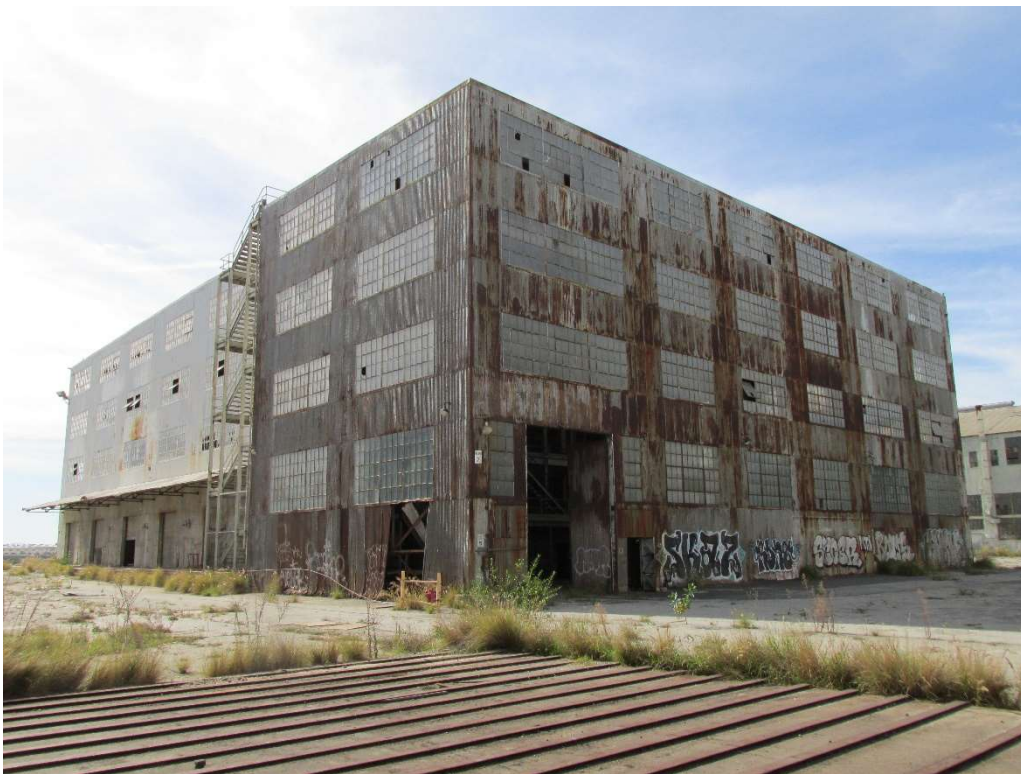
Figure 13. Machine Shop and Warehouse #7, Northeast Elevation, IMG_9332
