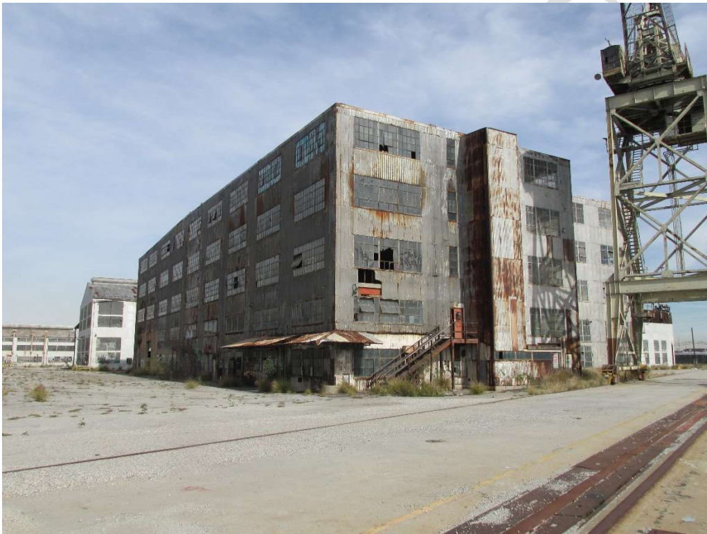
Figure 12. Machine Shop and Warehouse #7, Southwest Elevation, IMG_9279
