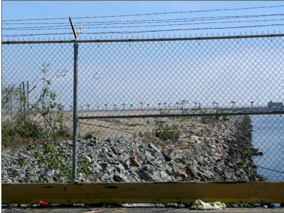
Photograph ES-2: Area of new wharf along Berth 306
