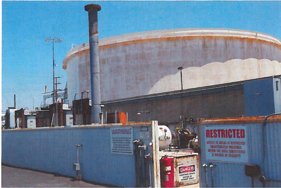
Photograph 5 Tank Farm, view facing east, 7/30/2012
