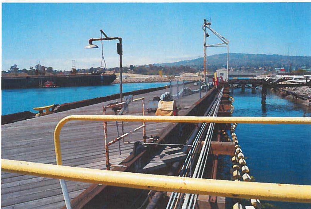
Photograph 2 Berth 119, 7/30/2012, view facing southwest
