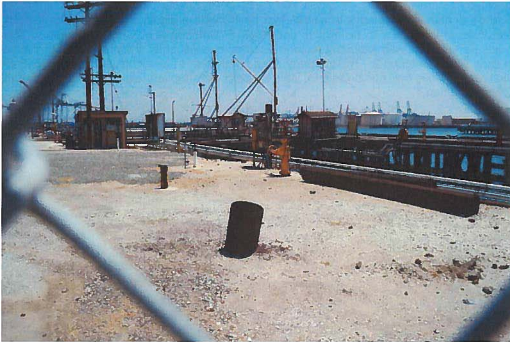
Photograph 3 Berth 120, view facing southeast, 7/30/2012
