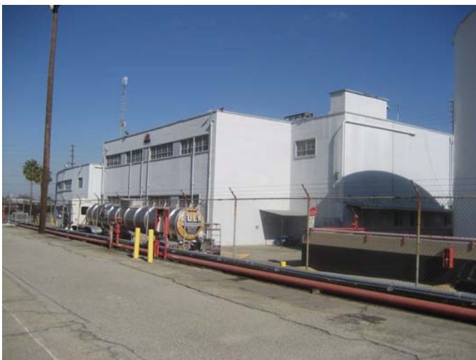
Office Building by Berth 187
