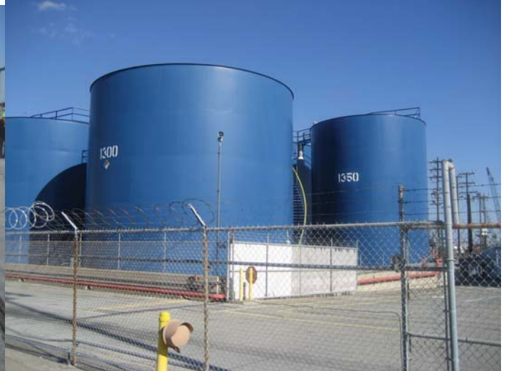
Tank Farm By Berth 188
