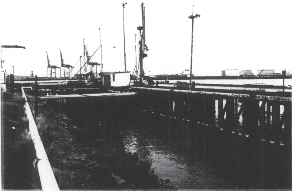
Photograph 5. Wharf at Berth 120
