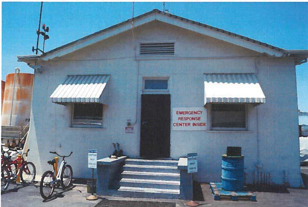
Photograph 4 Office Building, view facing east, 7/30/2012
