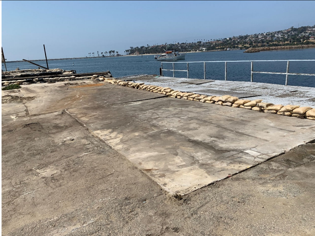
P-12 (Exterior – Conc Slabs along Seawall Directly South of Bldg)
