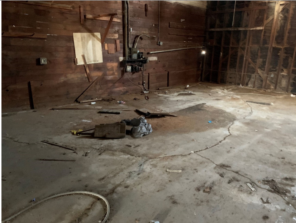
P-11 (Interior – Wood Shop Floor and Partition Wall w/ Public Counter)
