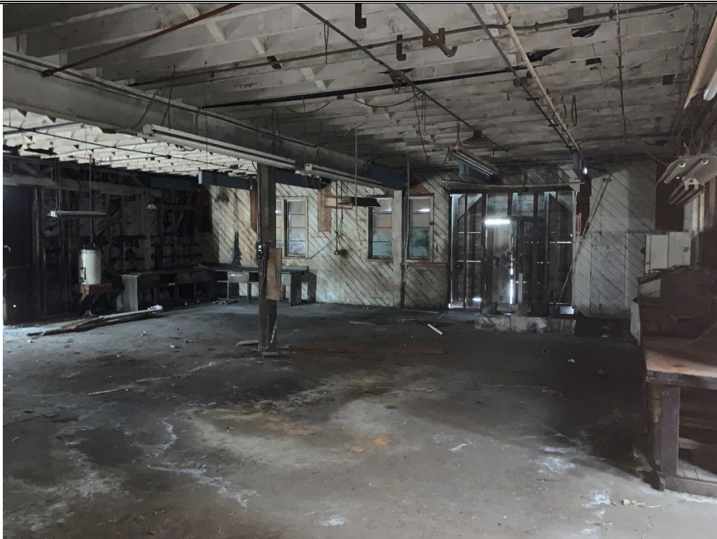
P-8 (Interior – Machine Shop, South and West Wall)
