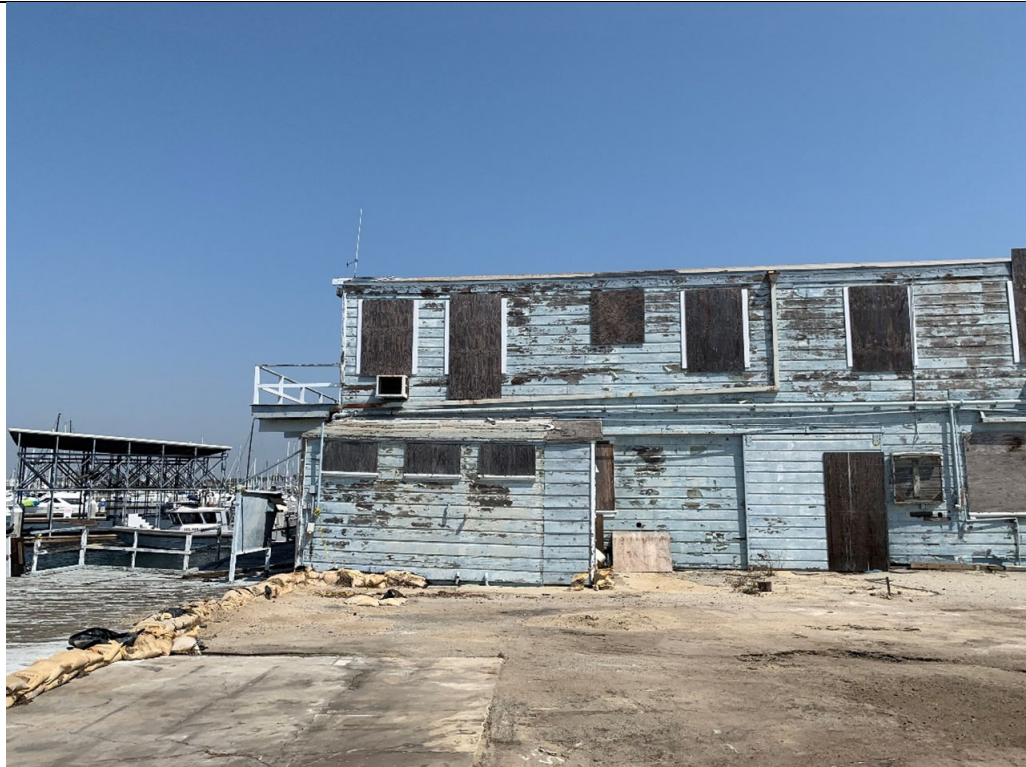
P-4 (Exterior – South Side)
