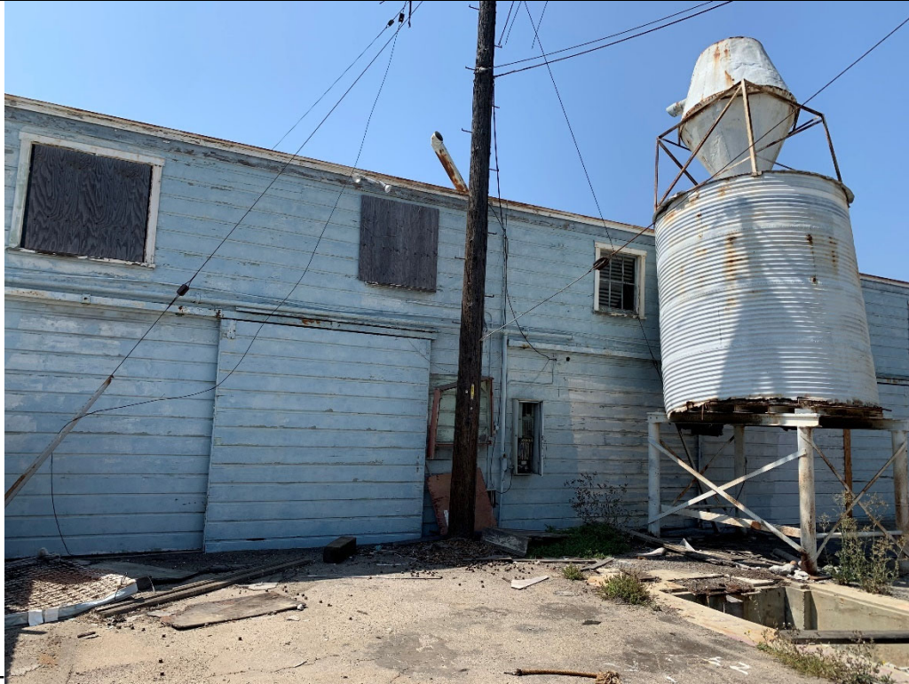
P-1 (Exterior – North Side Lumber Shed)
