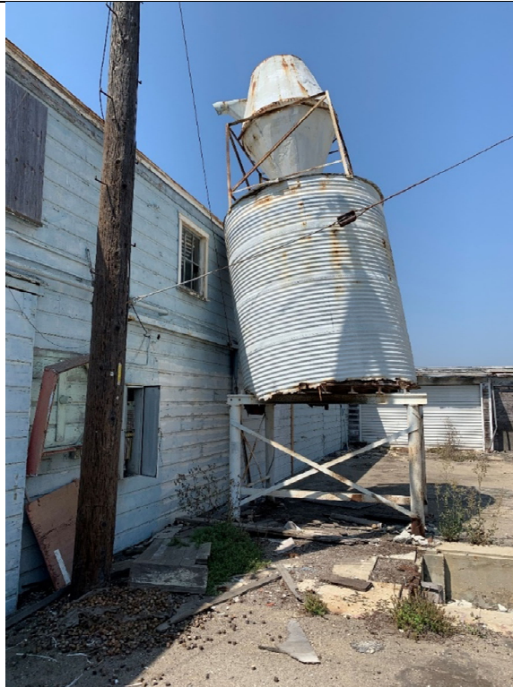
P-2 (Exterior – N Side Lumber Shed, E Side Original Bldg, Silo)
