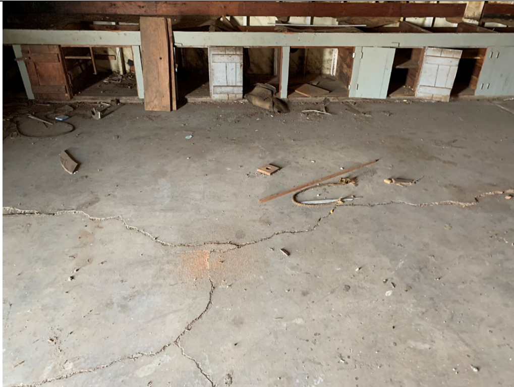
P-10 (Interior – Wood Shop Floor and Partition Wall w/ Machine Shop)
