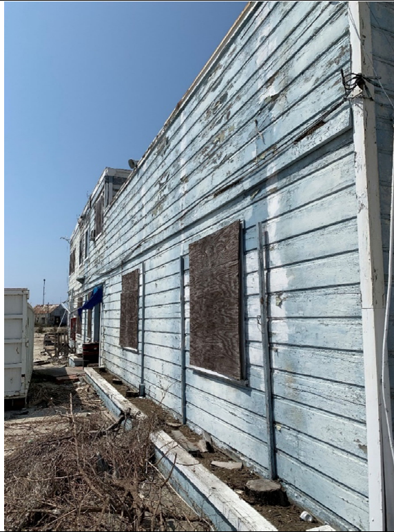
P-3 (Exterior – East Side Lumber Shed, Office/Shop)
