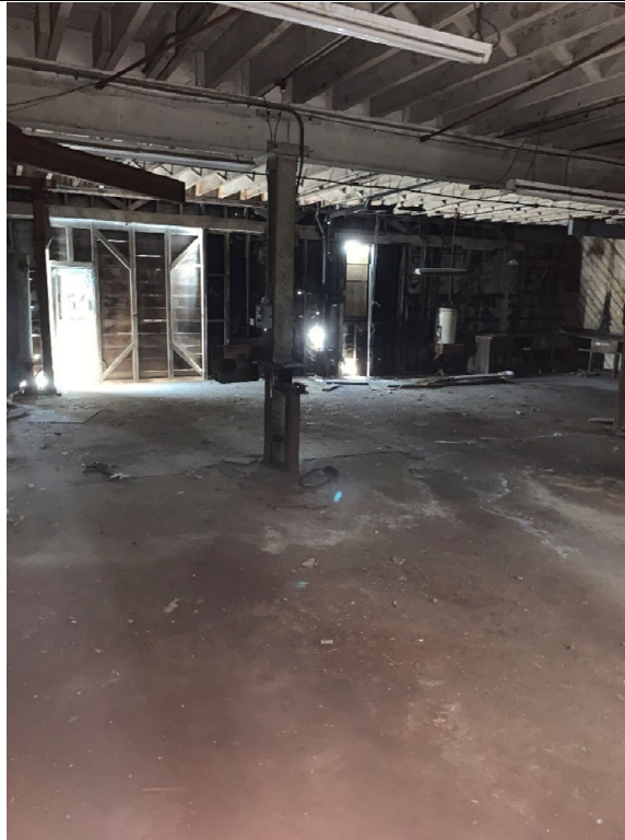
P-9 (Interior – Wood Shop Floor and South Wall)
