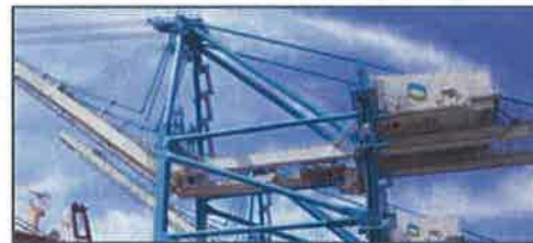
EFFICIENCY UPGRADES TO SHORE CRANES
