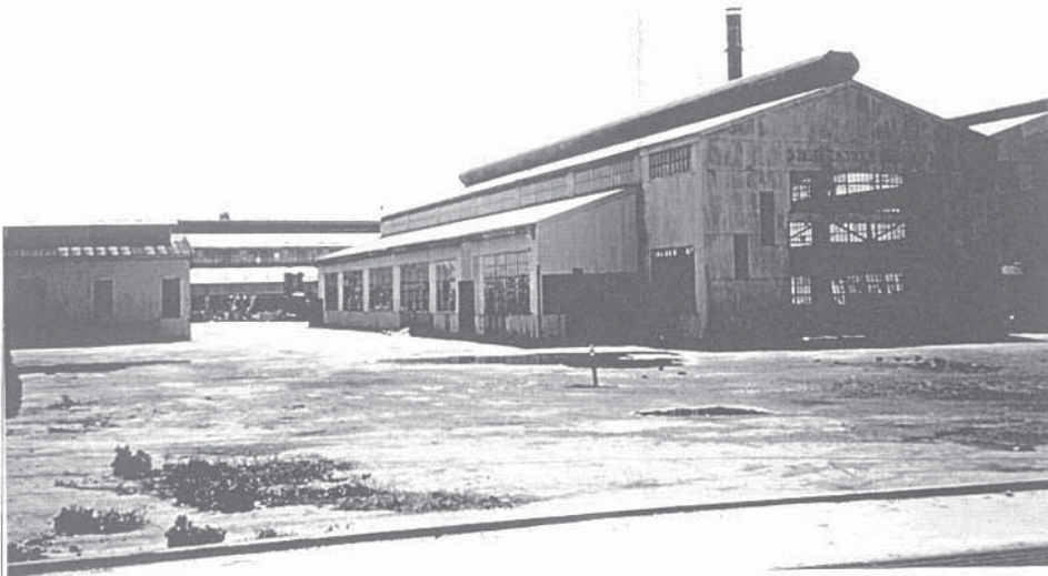
Photograph 2. Shed-roofed, metal-sided extension
