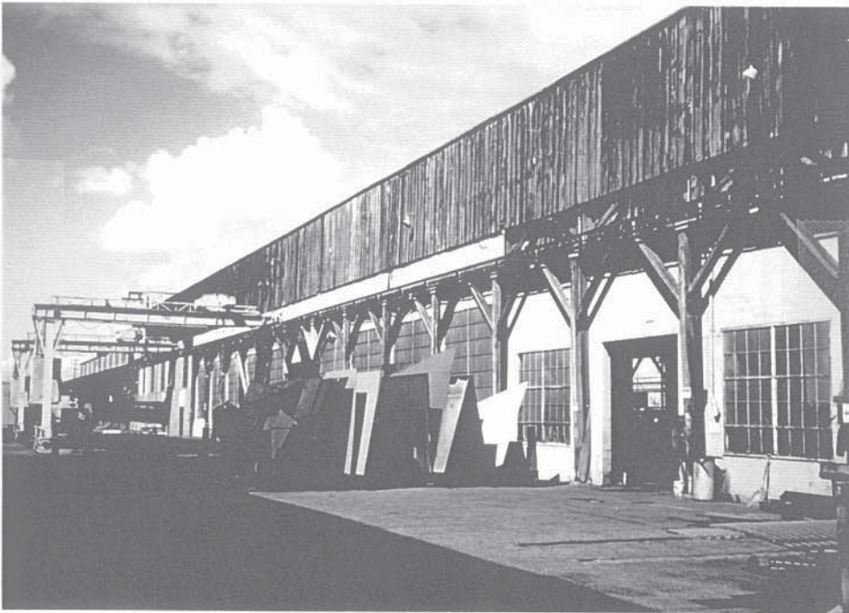
Photograph 2. West elevation showing wood trusses
