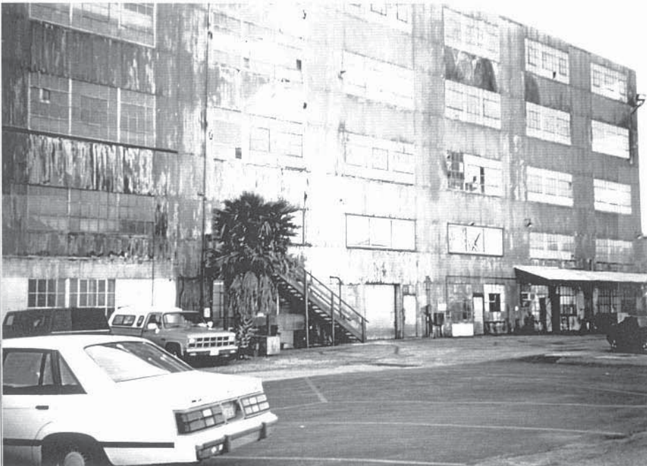
Photograph 3. Replacement windows and metal awning
