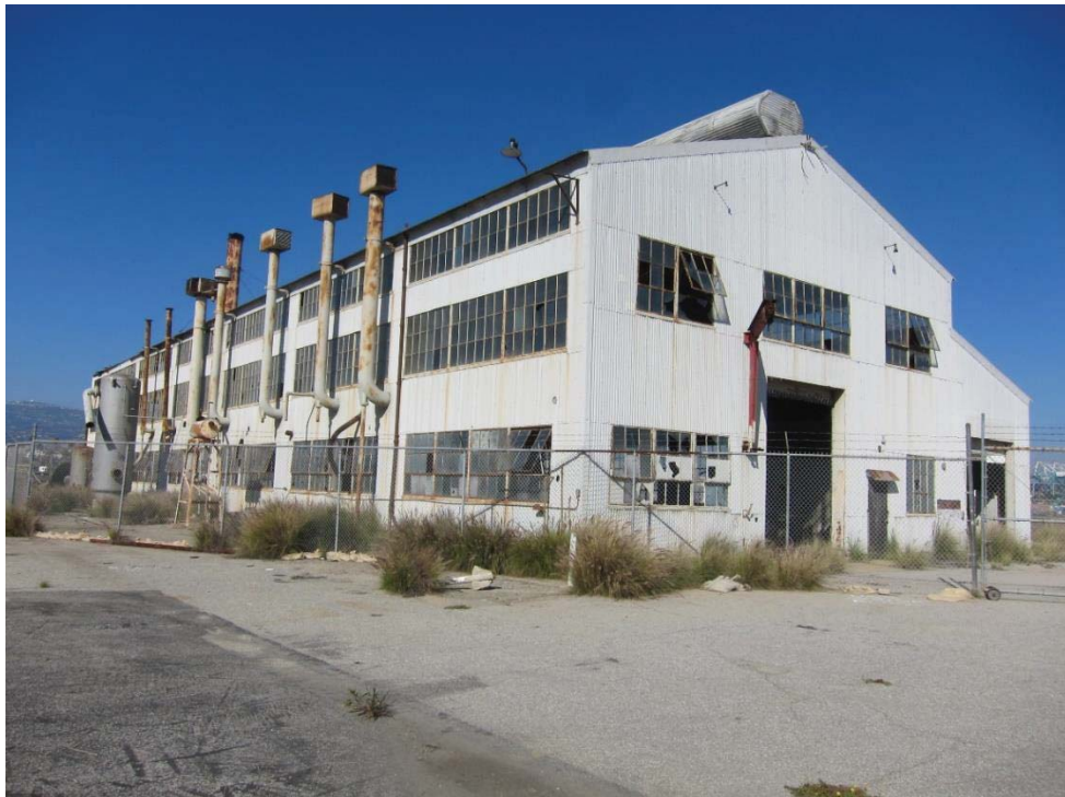
Figure 4 Southeast Elevation of Compressor House
