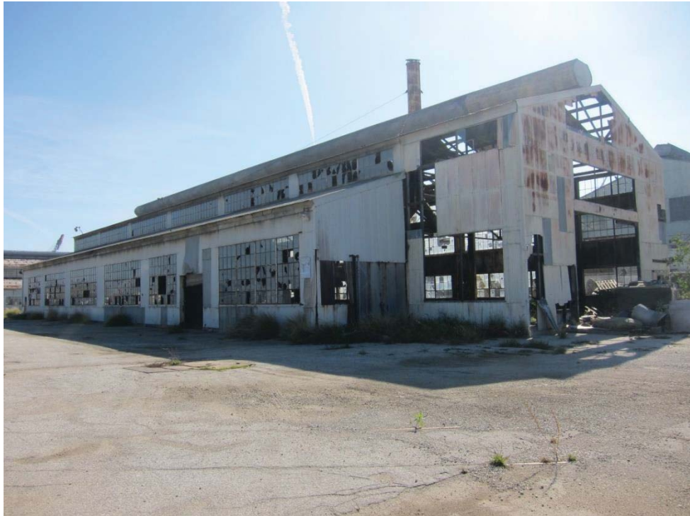
Figure 5 Northwest Elevation of Compressor House
