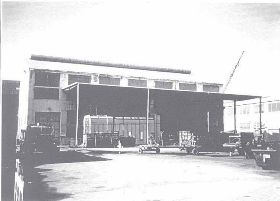
Photograph 2. Metal shelter at rear of building
