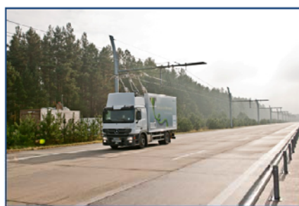
Figure 6 Truck Catenary (Siemens)
