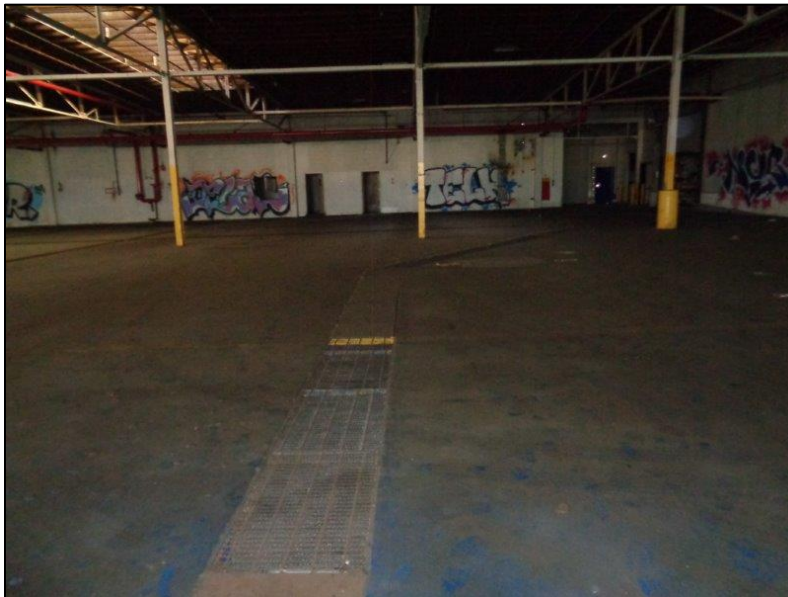
Figure 28: Star-Kist Plant No. 4, interior, warehouse/manufacturing area showing drains in floor, camera facing east. ICF, 2018.
