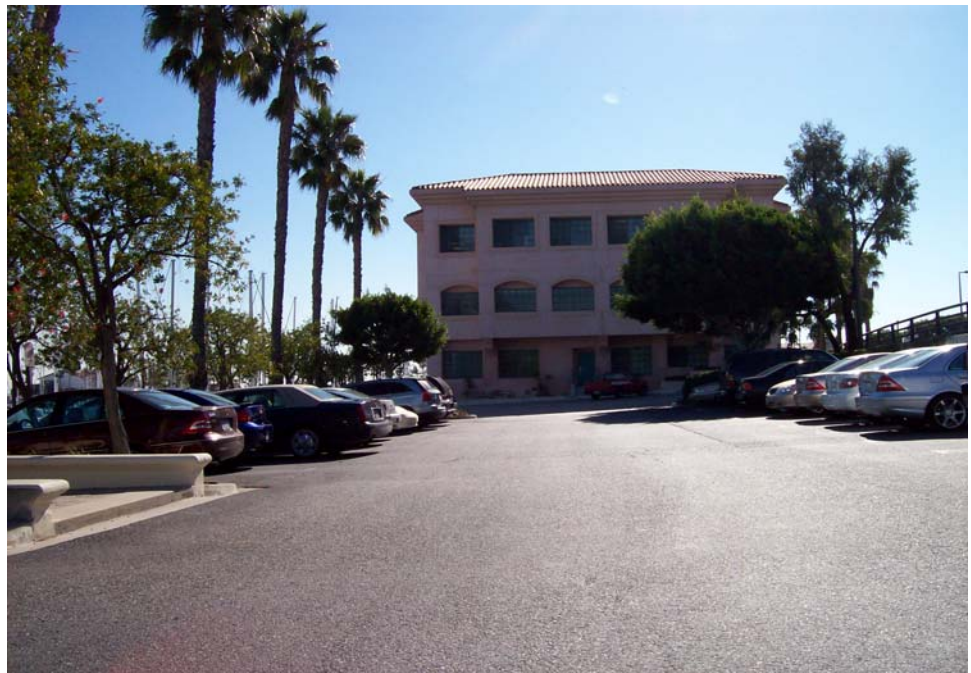
Photograph No. 12: Typical office building located in Area D.
