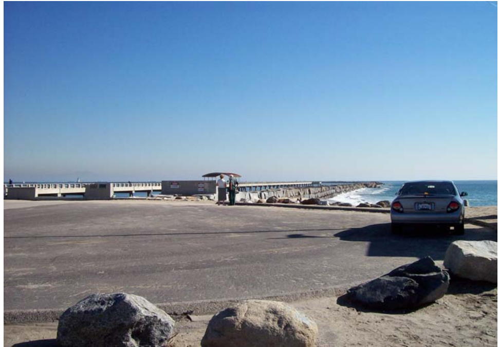
Photograph No. 27: Breakwater located in Area F.
