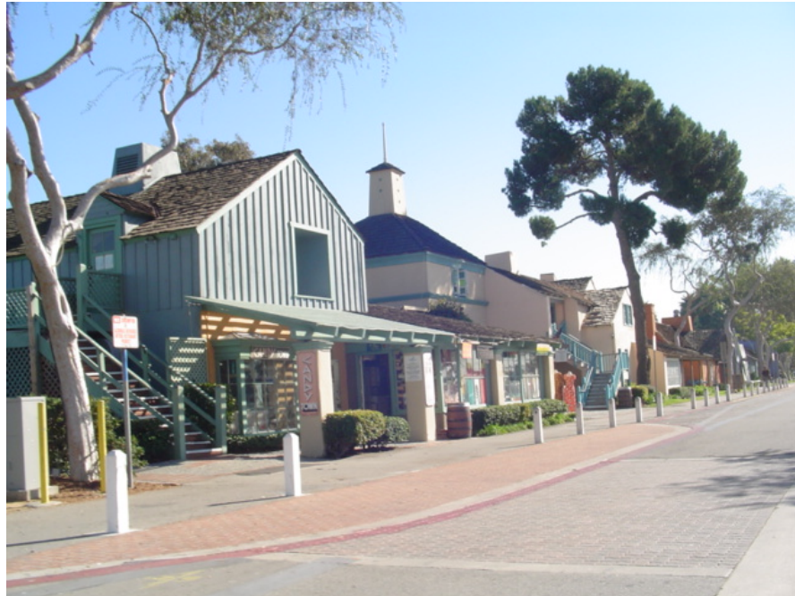
Photograph No. 7: View along the Port O' Call Village along Nagoya Way located in Section C.
