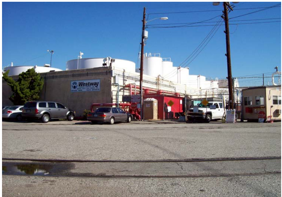
Photograph No. 14: Looking east at the Westway Terminal Tank Farm located in Area E.
