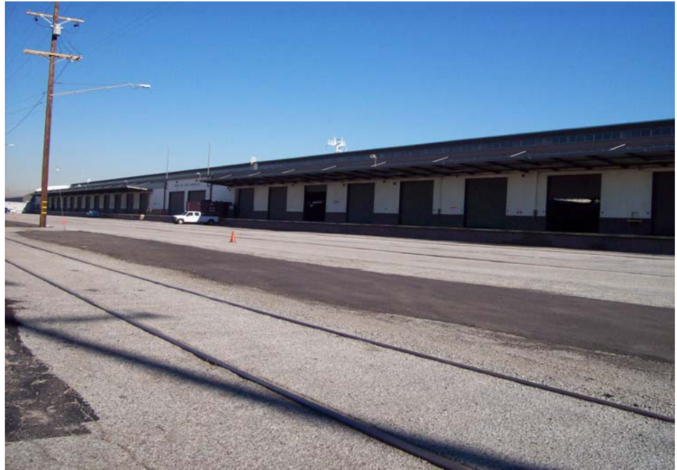
Photograph No. 15: Typical POLA warehouses located in Area E.
