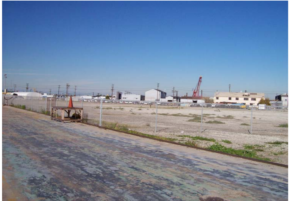
Photograph No. 29: Looking northeast at the Berth 240 area from the wharf.
