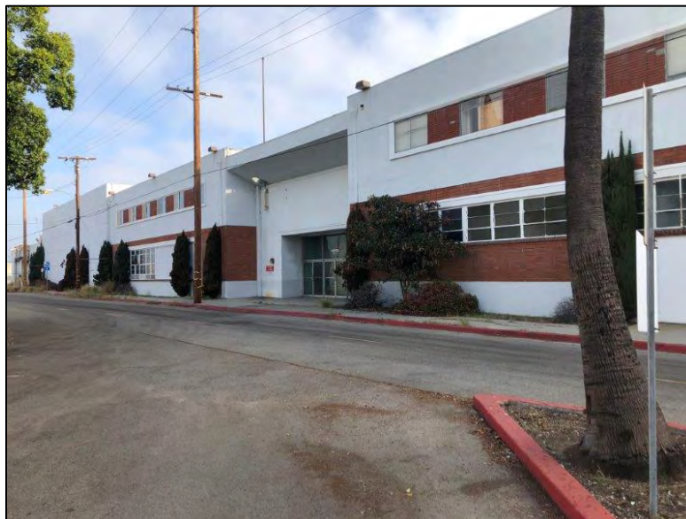
Figure 2: Star-Kist Plant No. 4, primary (west) elevation showing entrance, camera facing northeast. ICF, 2018.
