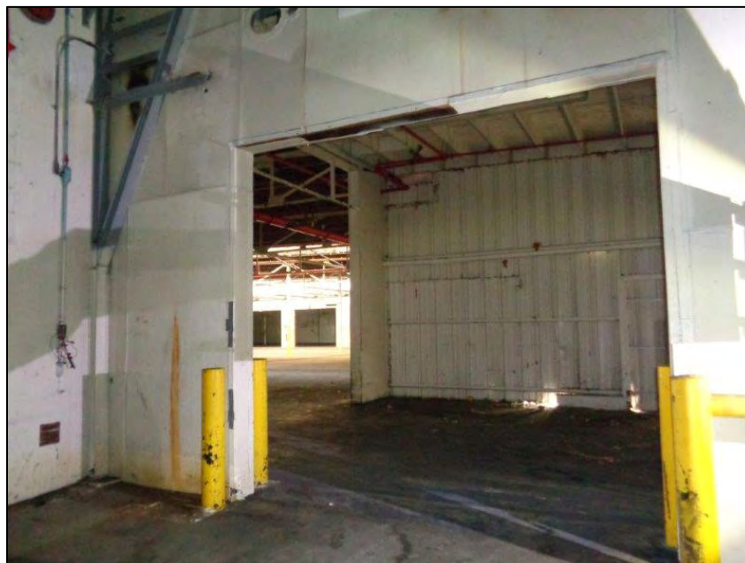
Figure 30: Star-Kist Plant No. 4, interior, warehouse/manufacturing area, camera facing east. ICF, 2018.
