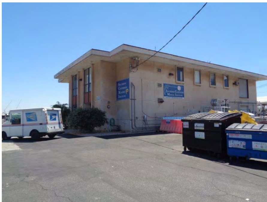
Figure 10-12. Southern California Marine Institute, primary (north) and west elevations, camera facing southeast.
