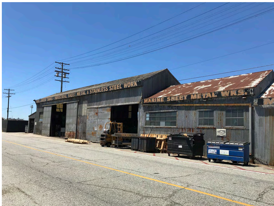
Figure 10-5. DeVries Sheet Metal, primary (west) elevation, camera facing southwest.
