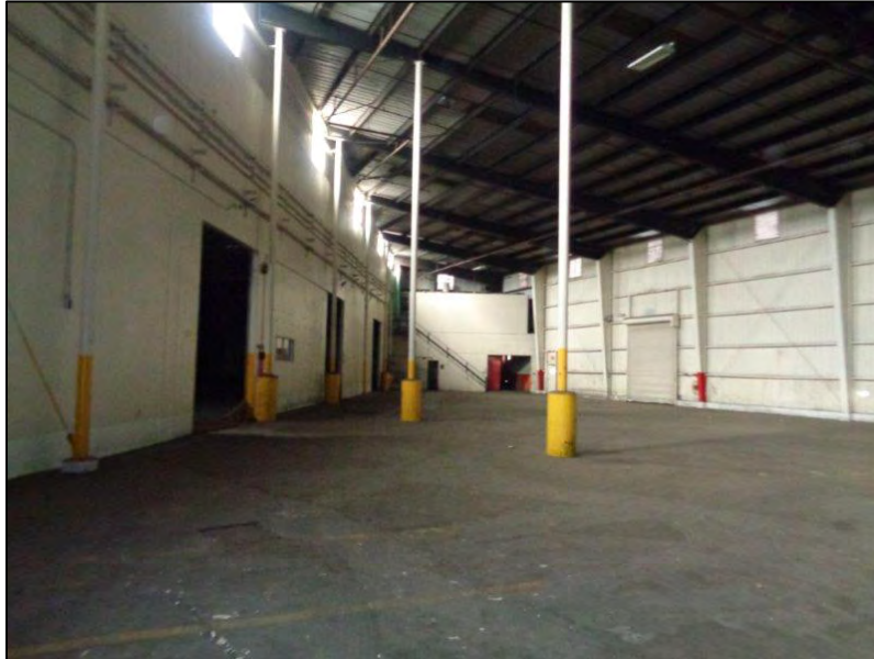
Figure 29: Star-Kist Plant No. 4, interior, warehouse/manufacturing area at north portion of Plant, camera facing west. ICF, 2018.
