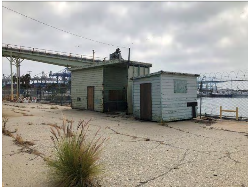
Figure 19: Star-Kist Plant No. 4, south elevation's ancillary/related buildings/structures, showing tuna import bridge in background, camera facing southeast. ICF, 2018.
