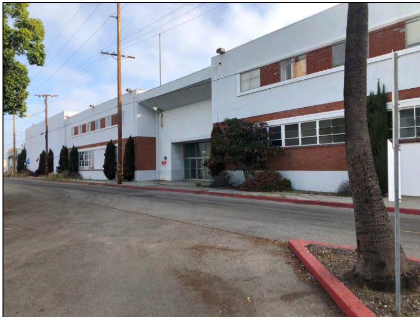
Figure 5-3. Star-Kist Plant No. 4, primary (west) elevation showing entrance, camera facing northeast. ICF, 2018.
