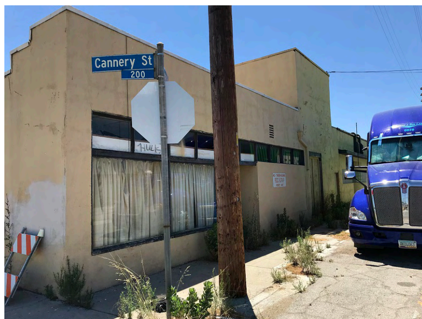
Figure 10-2. Nakamura Multi-Use Building, primary (west) elevation, camera facing southeast. ICF, 2020.
