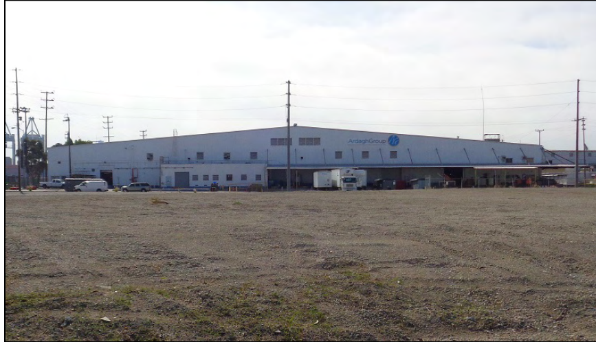
Photograph 1: North elevation, Can Manufacturing (formerly Impress Plant) portion of facility, camera facing south. ICF, 2018.
