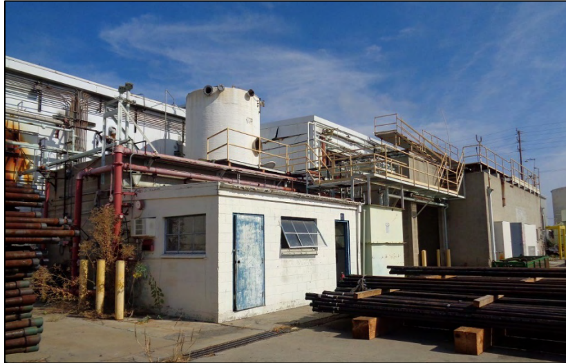
Photograph 5: South elevation, Cold Storage portion of the facility, camera facing northeast. ICF, 2018.
