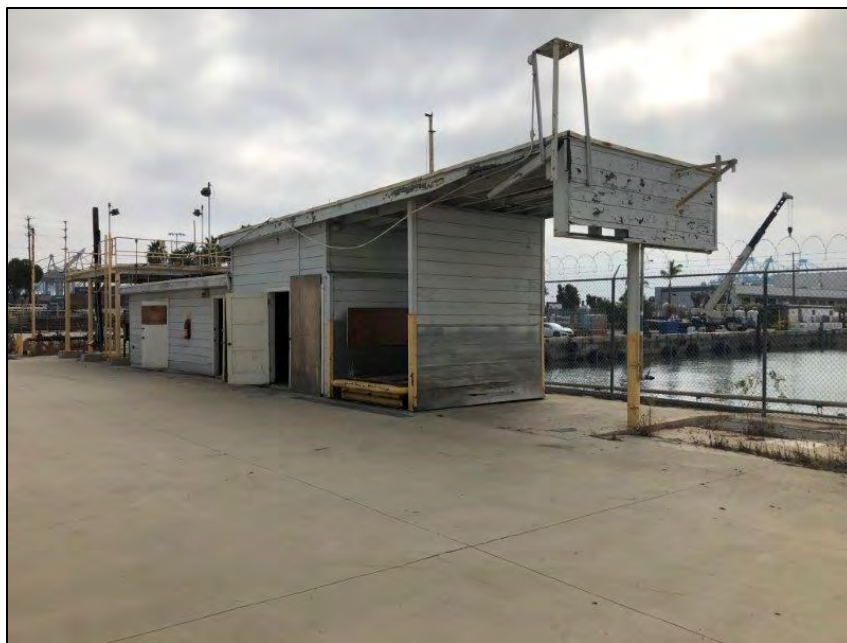
Figure 5-22. Star-Kist Plant No. 4, ancillary/related buildings/structures adjacent to south elevation, southeast corner of Plant No. 4, camera facing southeast.
