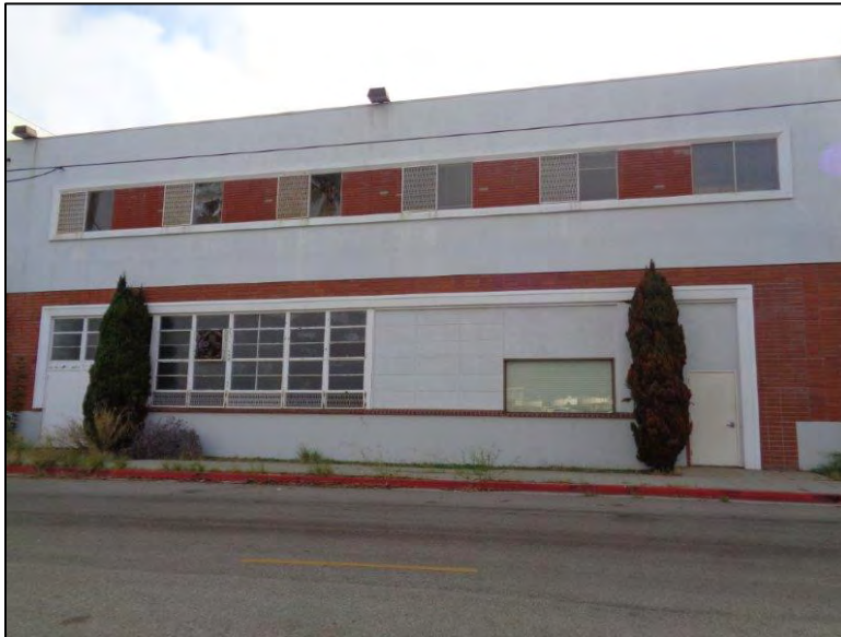
Figure 5: Star-Kist Plant No. 4, primary elevation, detail of third volume from the north, north wing, camera facing east. ICF, 2018.
