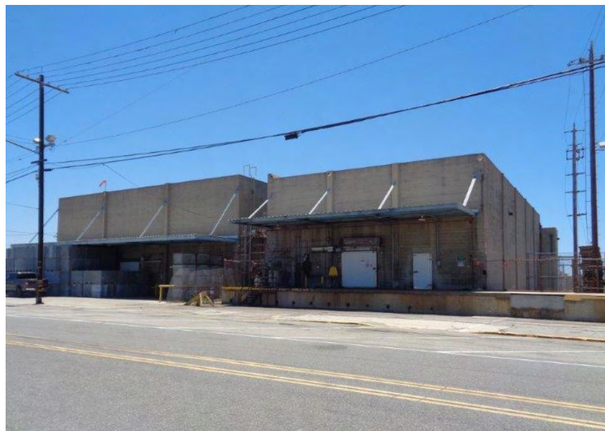
Figure 10-11. Van Camp Sea Food Company, primary (north) elevation and west elevation, camera facing southeast.
