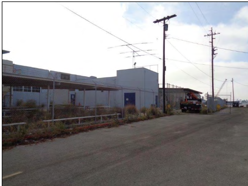
Figure 12: Star-Kist Plant No. 4, primary (west) elevation, overview of southwest corner of Plant No. 4 (volumes 7-9), camera facing southeast. ICF, 2018.
