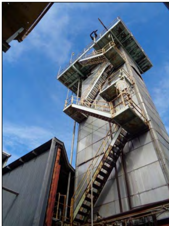
Figure 5-25. Star-Kist Plant No. 4, rear (east) elevation, multi-story tower at center of rear (east) elevation, camera facing north.
