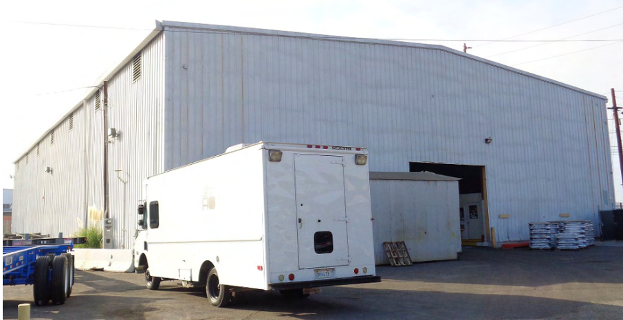
Figure 5-33. North and west elevations, camera facing south.
