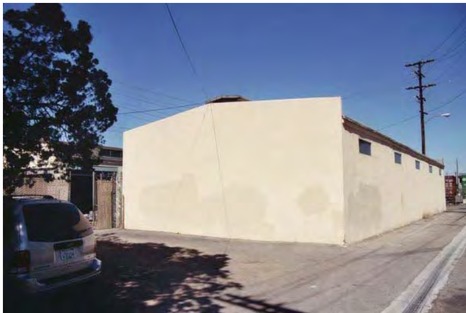
Photo 29. Looking northeast at the western elevation of the Net Repair Sheds (“Boneyard”)
