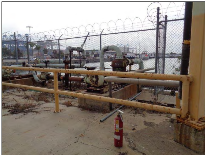
Figure 20: Star-Kist Plant No. 4, ancillary/related buildings/structures adjacent to south elevation, showing pipes, railings, fencing, and concrete pads, camera facing southeast. ICF, 2018.
