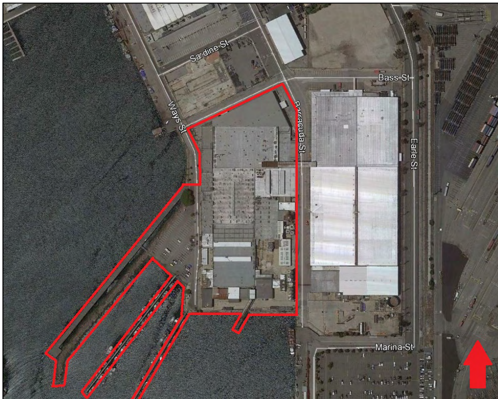
Figure 5-1. Aerial map showing Plant No. 4 boundary.
