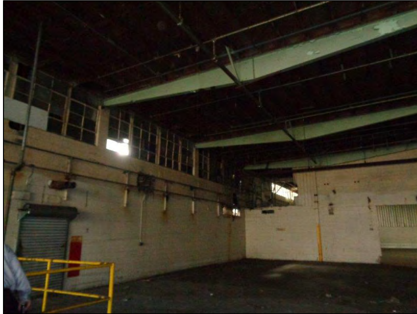
Figure 31: Star-Kist Plant No. 4, interior, warehouse. ICF, 2018.
