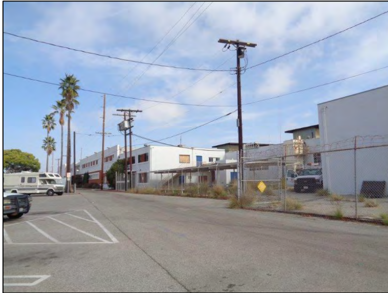
Figure 1: Star-Kist Plant No. 4, primary (west) elevation, camera facing northeast. ICF, 2018.
