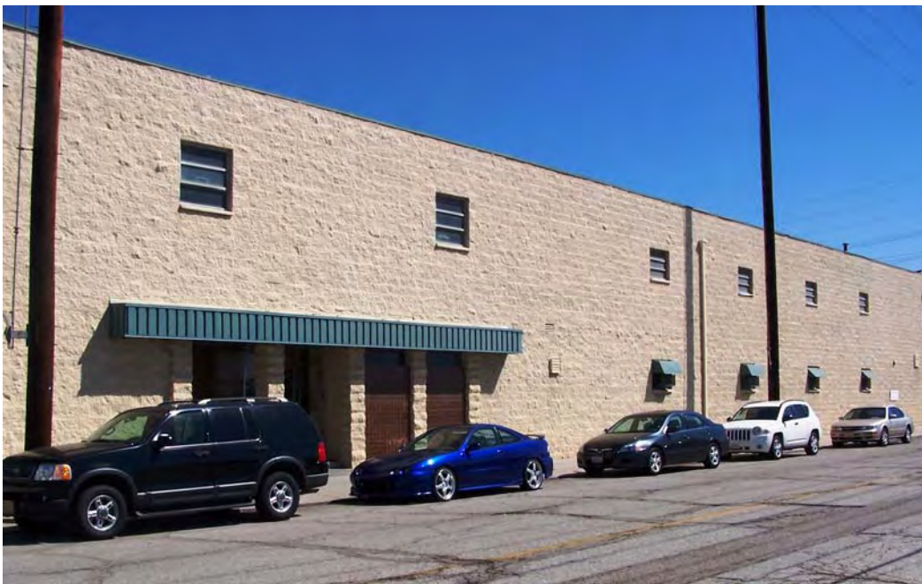
Photo 28. Looking southeast across Tuna Street at the western elevation of the Pilot Plant
