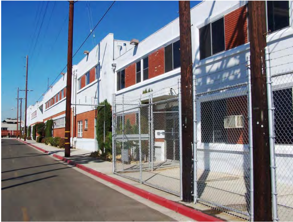
Photo 20. Looking northeast at the center of the western elevation of original plant
