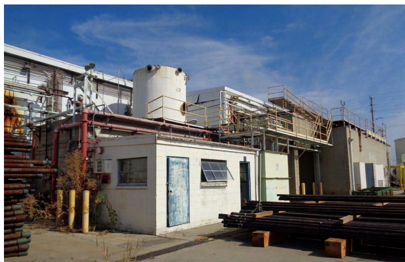
Figure 5-40. South elevation, Cold Storage portion of the facility, camera facing northeast. ICF, 2018.
