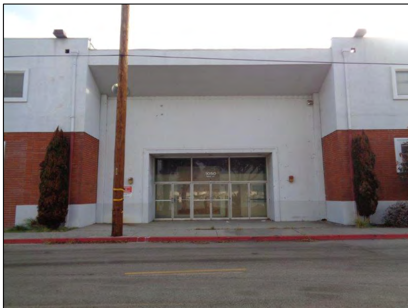
Figure 5-4. Star-Kist Plant No. 4, primary (west) elevation, detail of third volume from the north, entrance pylon, camera facing east. ICF, 2018.
