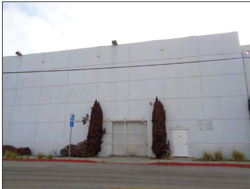
Figure 8: Star-Kist Plant No. 4, primary (west) elevation, detail of second volume from the north, camera facing east. ICF, 2018.
