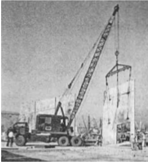
Figure 7-1. Construction of Star-Kist Plant No. 4.
