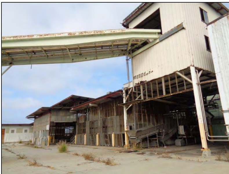
Figure 5-16. Star-Kist Plant No. 4, south elevation, southwest corner of Plant, showing remaining tuna import bridge, camera facing northwest.
