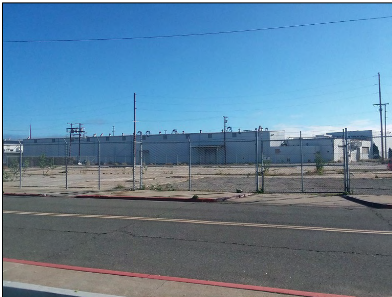
Figure 14: Star-Kist Plant No. 4, north elevation, camera facing south. ICF, 2019.
