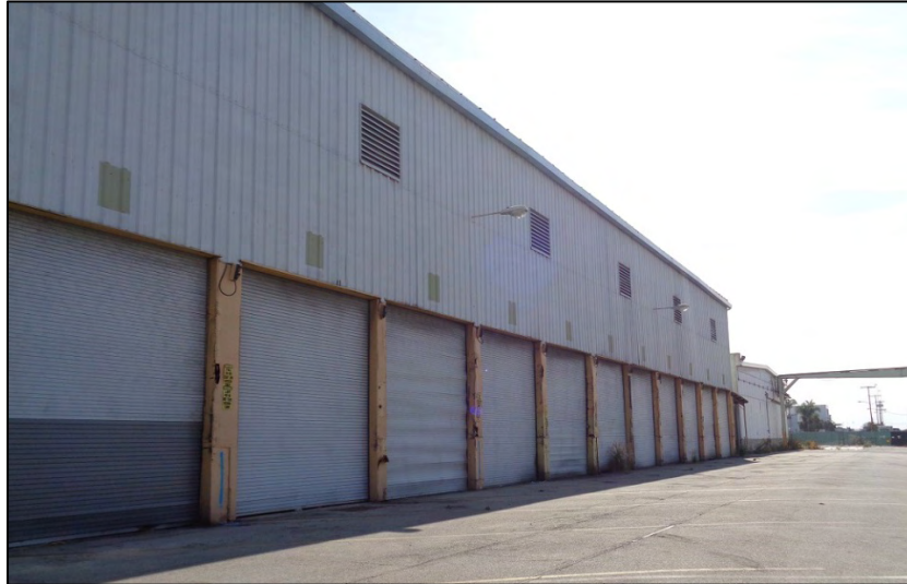
Photograph 3: West elevation, Warehouse (formerly distribution) portion of facility in foreground (left) and Cold Storage portion in the distance (right), camera facing south. ICF, 2018.
