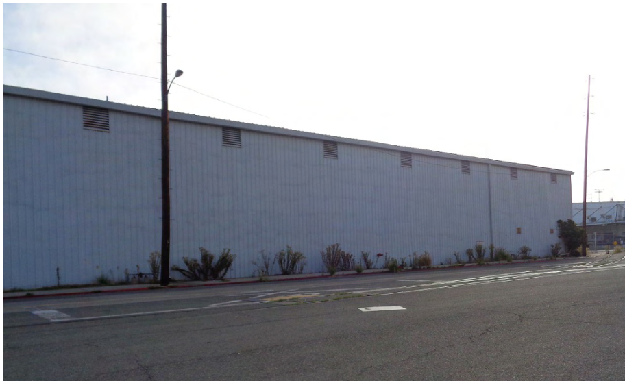
Figure 5-34. West elevation, camera facing southwest.
