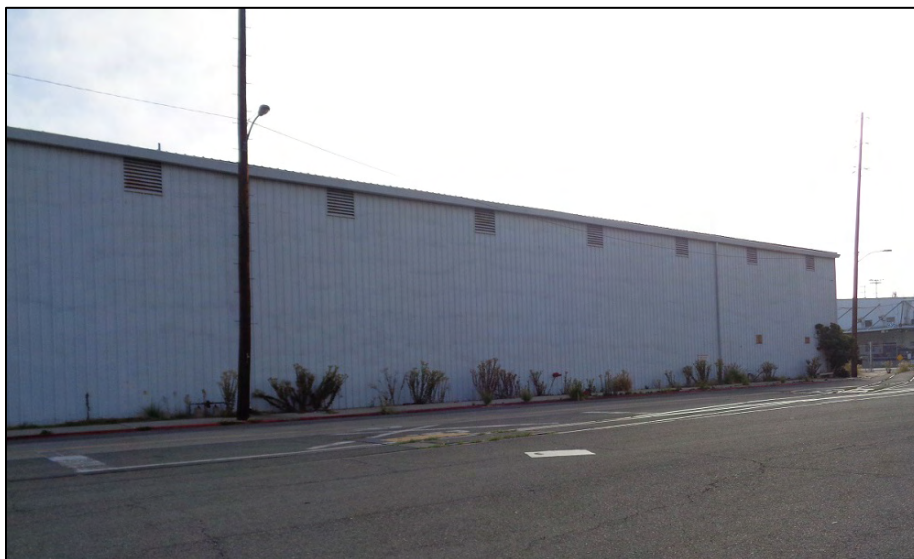
Photograph 2: west elevation, camera facing southwest. ICF, 2018.
