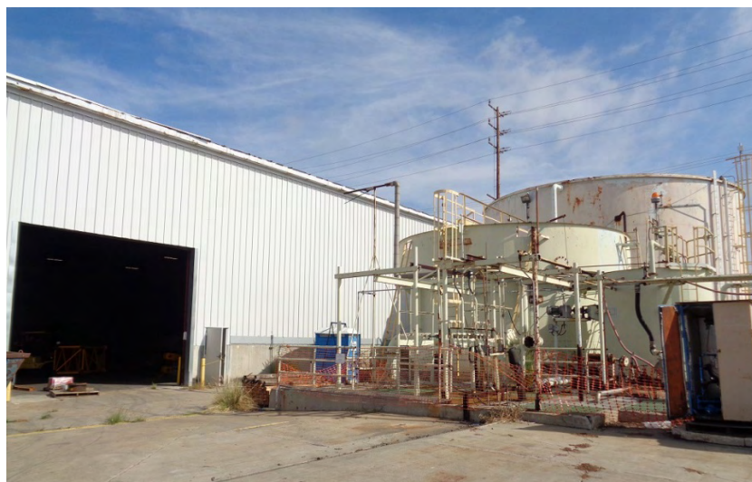
Figure 5-39. South elevation, Cold Storage portion of the facility, camera facing northeast. ICF, 2018.
