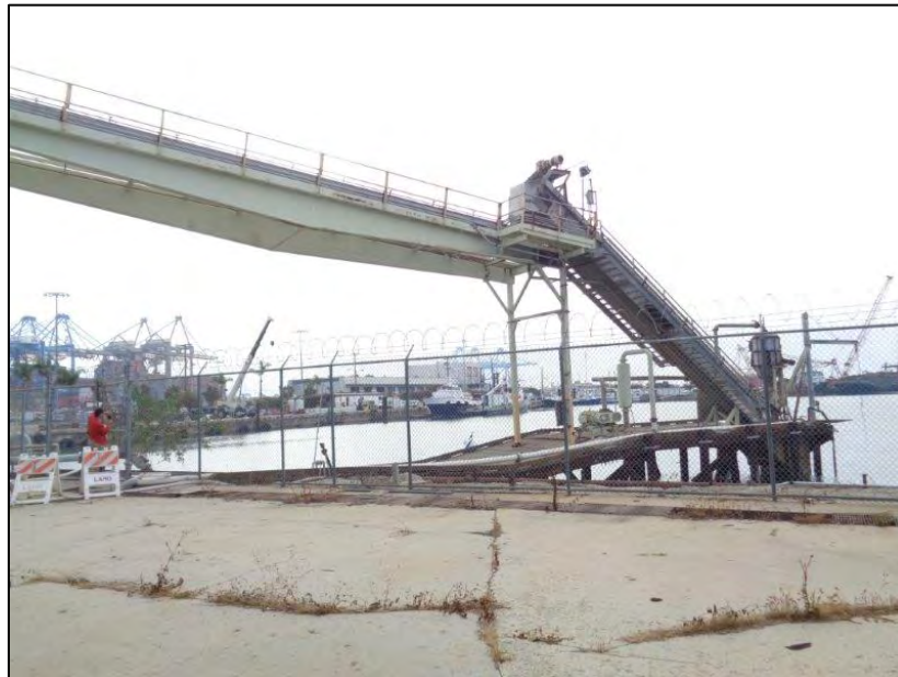
Figure 16: Star-Kist Plant No. 4, ancillary/related buildings/structures adjacent to south elevation, showing the only remaining tuna import bridge and dock, camera facing south. ICF, 2018.
