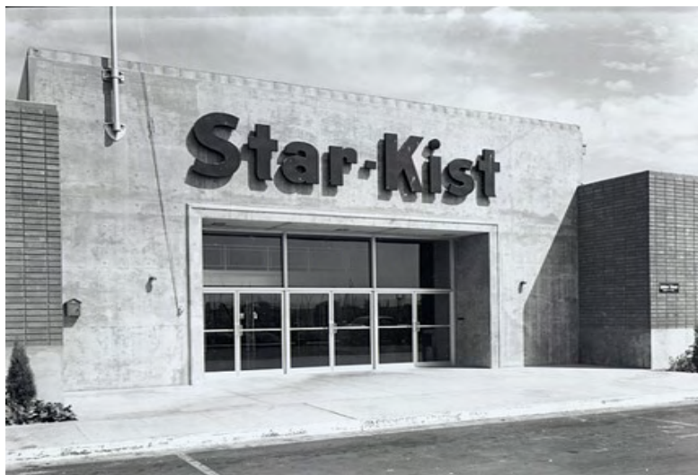
Photo 18. Entrance (L) as Identified in the Above Historic Aerial/Oblique (Source: Star-Kist Company pamphlet)
