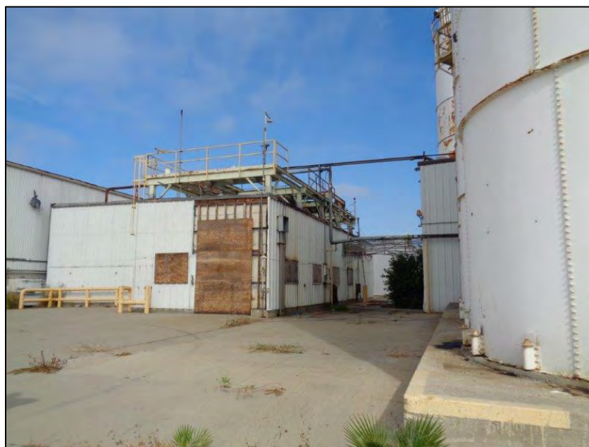
Figure 5-19. Star-Kist Plant No. 4, south and rear (east) elevations, southeast corner of Plant No. 4, camera facing north. ICF, 2018.
