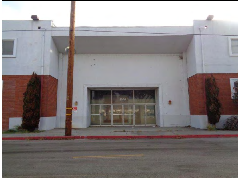
Figure 3: Star-Kist Plant No. 4, primary (west) elevation, detail of third volume from the north, entrance pylon, camera facing east. ICF, 2018.
