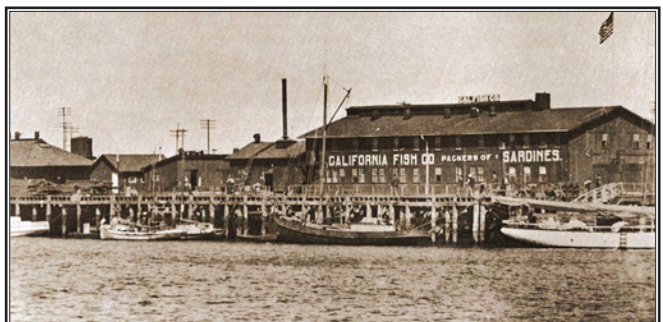
California Fish Company's first building, destroyed by fire in 1914 (Queenan 1983).
