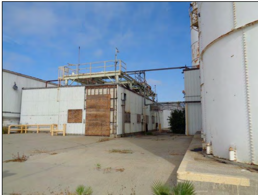
Figure 18: Star-Kist Plant No. 4, south and rear (east) elevations, southeast corner of Plant No. 4, camera facing north. ICF, 2018.
