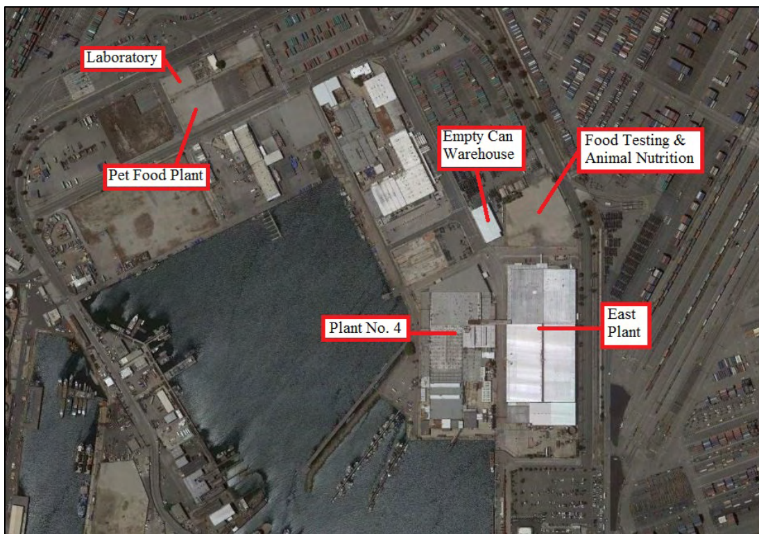
Figure 7-8. Star-Kist Facilities Associated with Plant No. 4.
