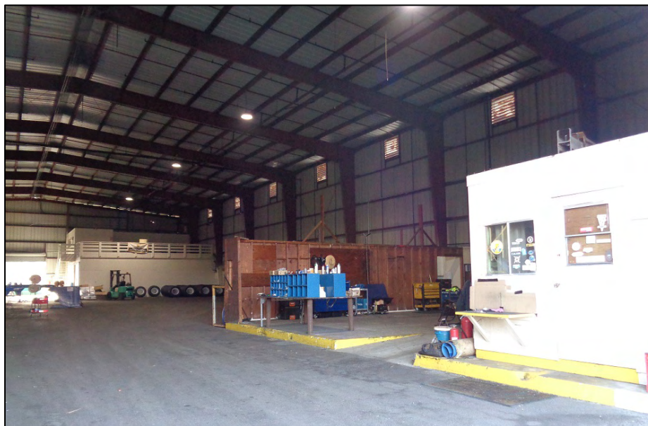
Photograph 3: Interior, camera facing south. ICF, 2018.
