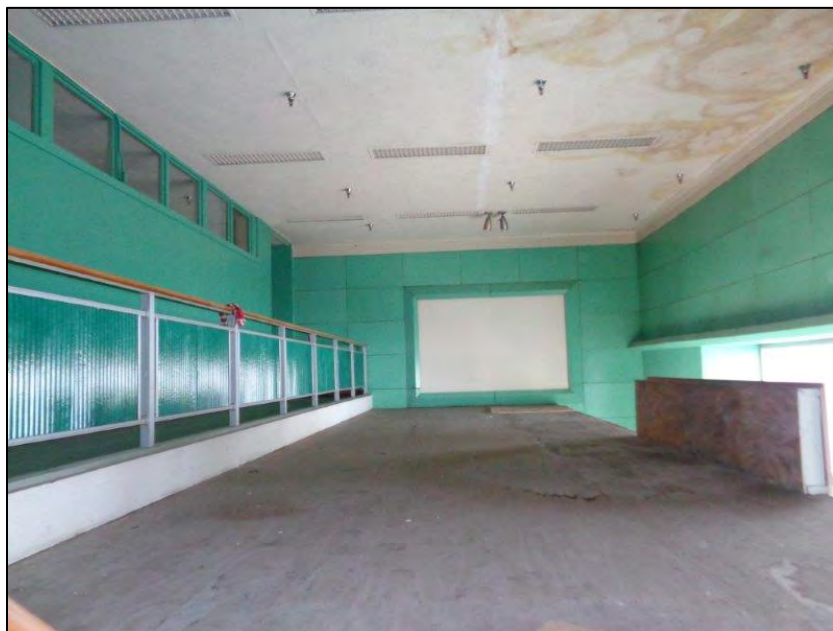
Figure 26: Star-Kist Plant No. 4, interior, entrance lobby shown from staircase landing, camera facing south. ICF, 2018.
