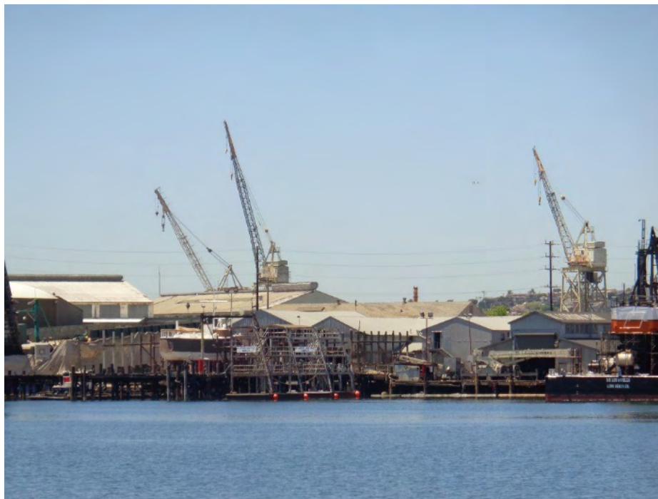
Figure 10-4. Al Larson Boat Shop, multiple buildings shown from Fish Harbor, camera facing west.
