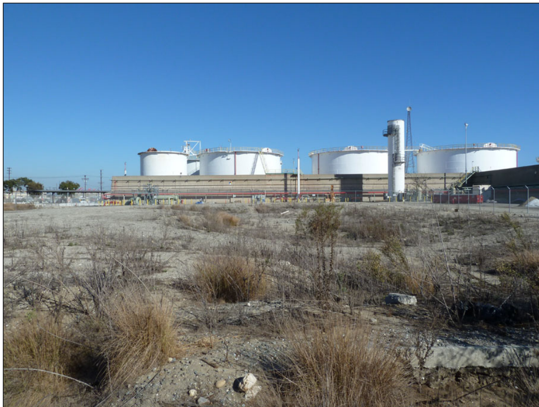
13 14 Photograph 2-2: Existing conditions at the 1.5-acre expansion area.
