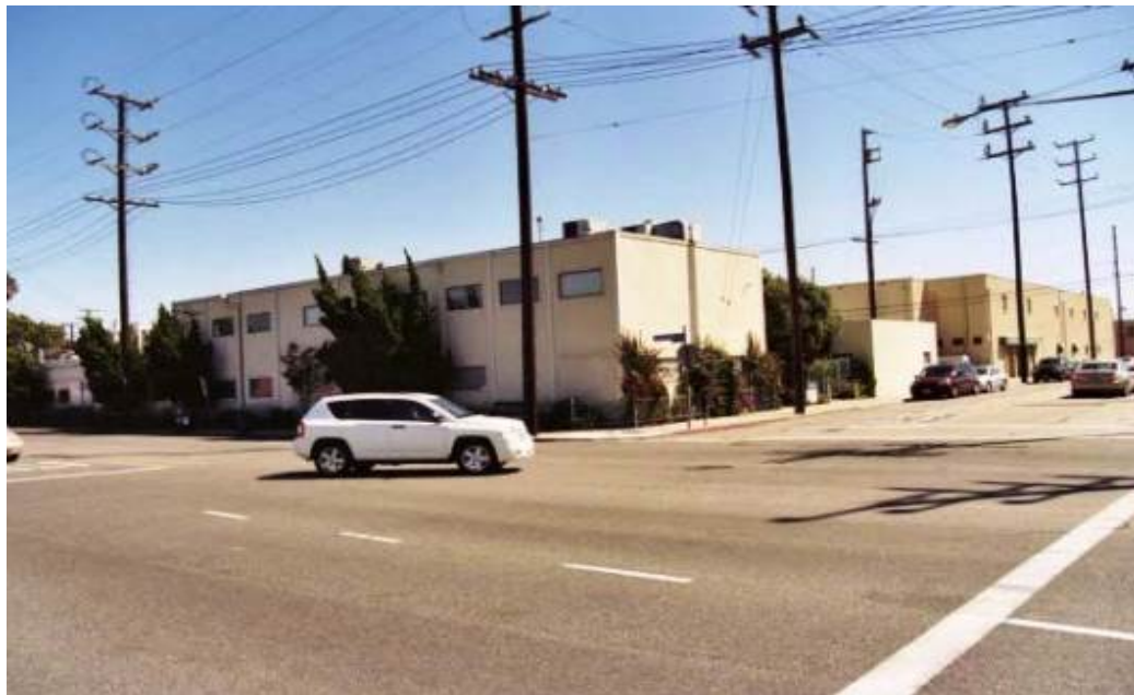
24 Photograph 2-5: Looking southeast across Terminal Way at the northwestern corner of 25 the Research Laboratory Complex. 26
