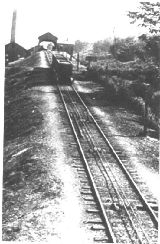
Figure 8.2. These coal carts from the late 1800s ran from mine to delivery station using gravitational forces. The central cable is wrapped around a two-pulley system to guide the cart along the tracks, and so empty carts can be manually hauled back up the hill.
