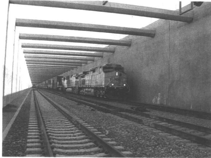
Figure 1.1: Mid-Corridor Trench with third rail.
