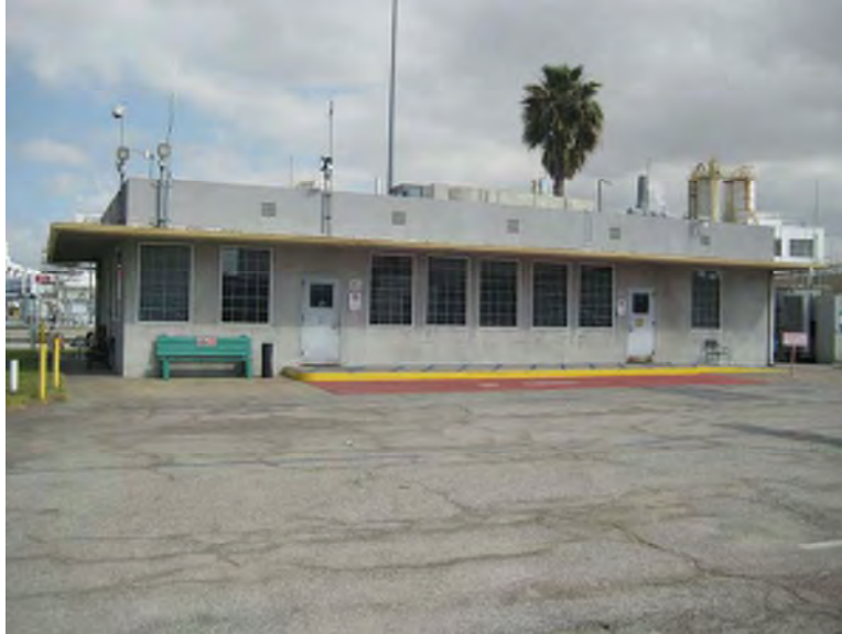
Photograph 2. View of office building, to the northeast.
