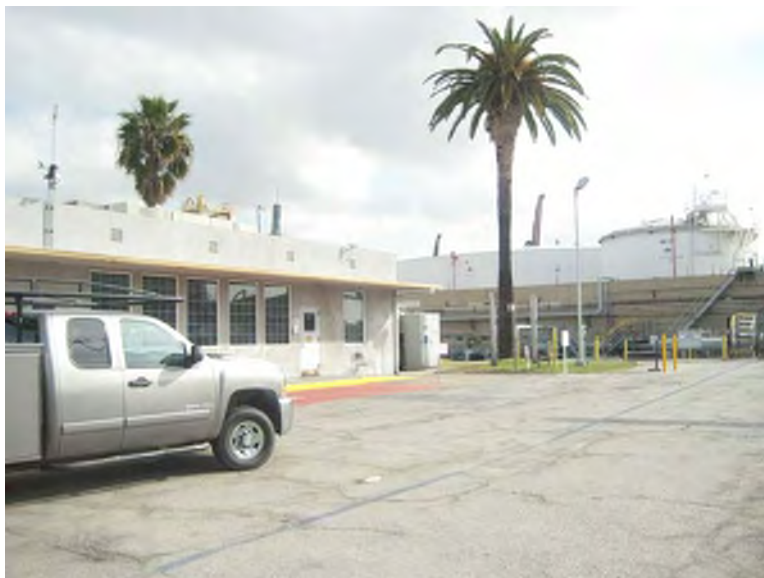
Photograph 3. View of storage tanks M-2 and M-17, view northeast.
