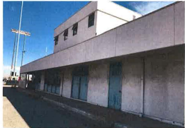
2. Gate Office Building
