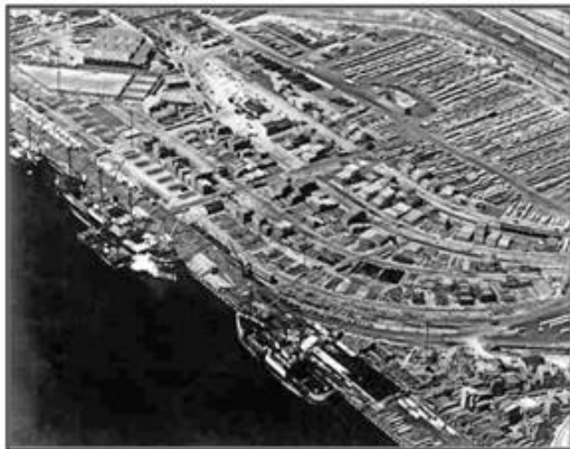
Aerial view of the inner harbor terminal in Wilmington (LAPL Photo Database).
