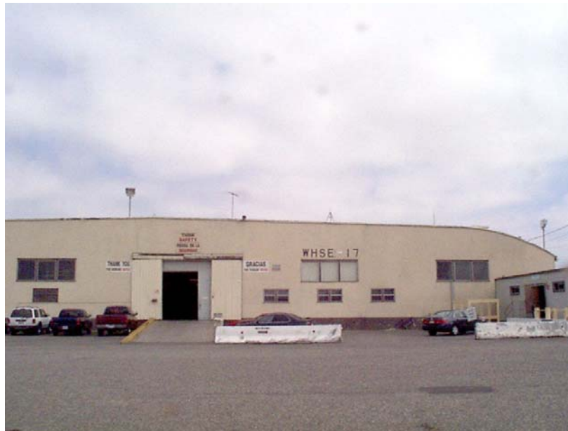
Looking north at building (warehouse) 17, south elevation.
