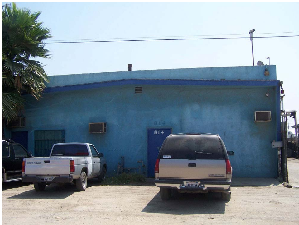
814 Sampson Avenue, looking east. Year built: 1965
