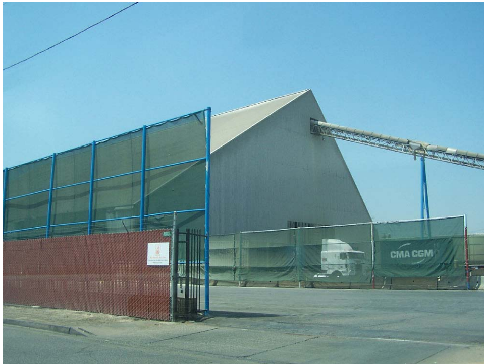
1001 Schley Avenue (processing building) looking northwest from corner of Schley Avenue and East I Street. Year built: c. 1983
