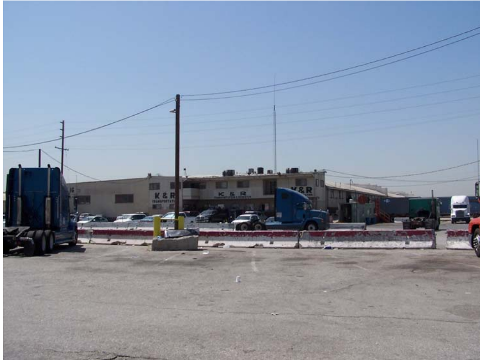
Photograph 3: Storage area and asphalt parking lot, looking south toward Phase I site.
