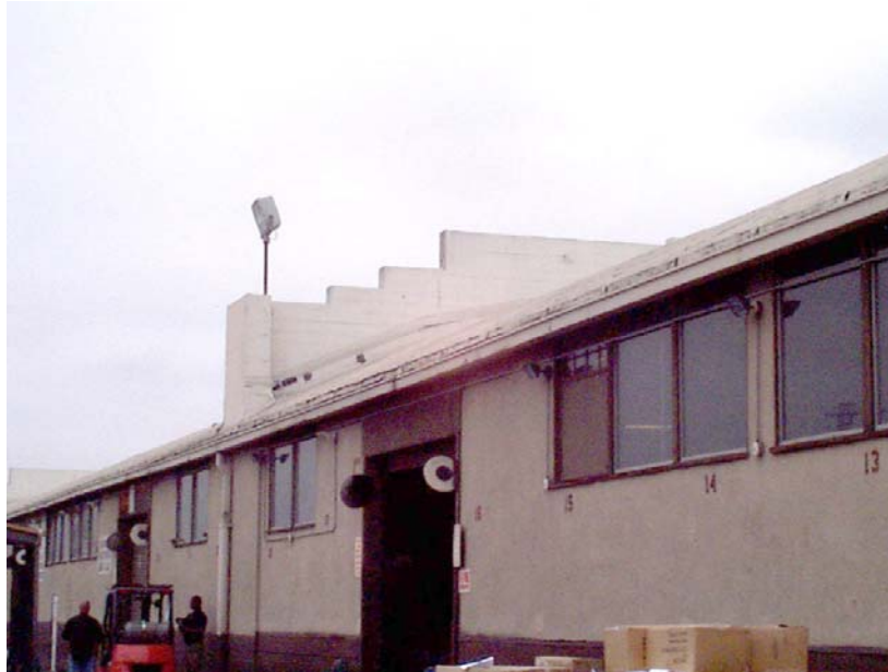
Looking southwest at building (warehouse) 13, east elevation.
