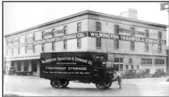
Northeast elevation of building at the corner of Fries Avenue and C Street (no date).
