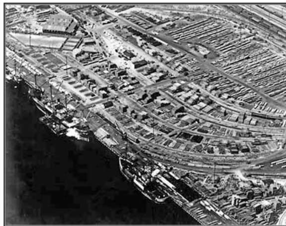
Aerial view of the inner harbor terminal in Wilmington (LAPL Photo Database).
