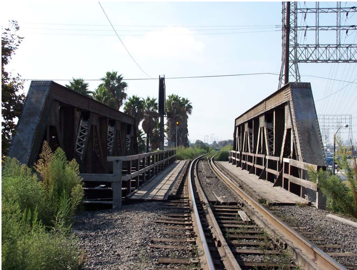
Looking south through the Sepulveda Boulevard Overcrossing at Willow Street
