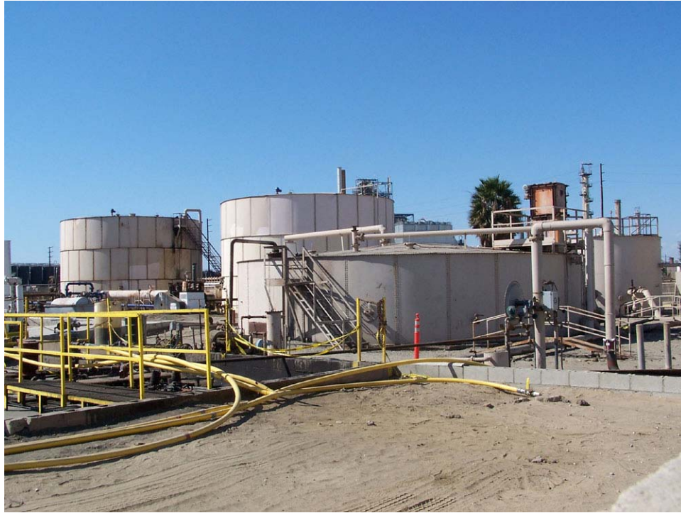
Warren E&P Tanks, 2209 E. I Street, looking northwest. Year built: c. 1960
