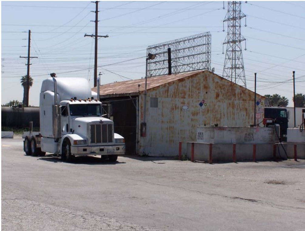
Photograph 1: Metal storage shed, looking east.
