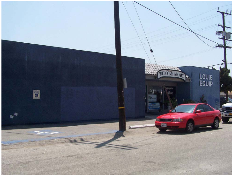
2401 East Anaheim Street, looking southeast from Schley Avenue. Year built: 1972/1979
