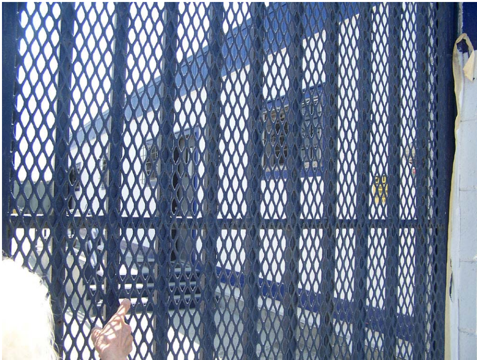
Structure on Schley Ave, north of East I Street, looking east. Address unknown; Year built: unknown
