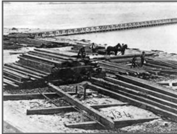
Construction of breakwater in Wilmington in 1876 (LAPL Photo Database).
