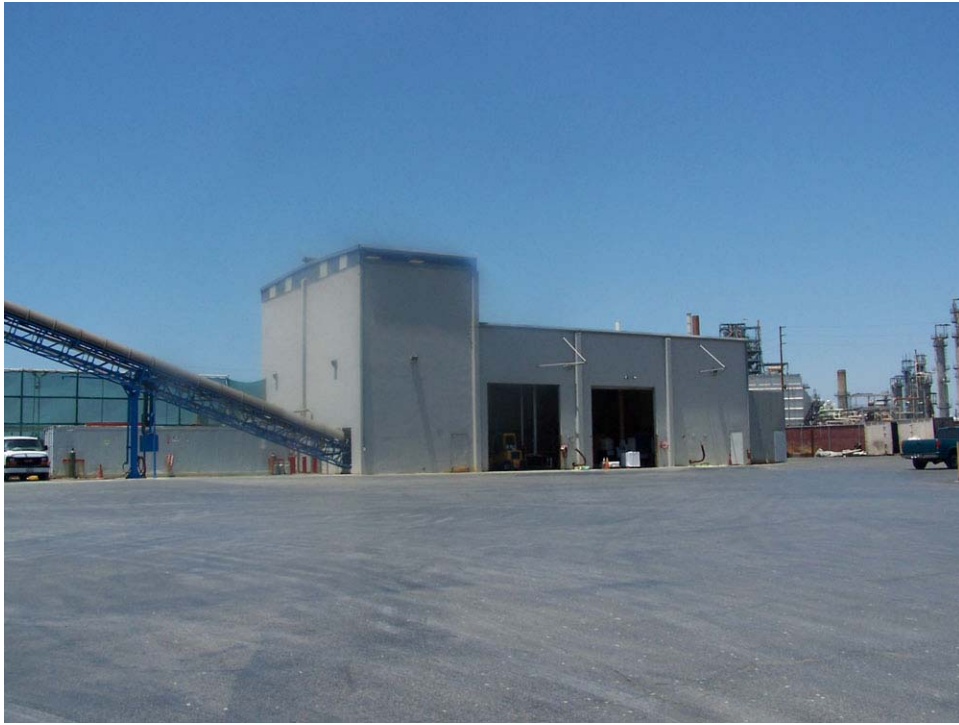
1001 Schley Avenue (storage barn), looking west. Year built: c. 1983
