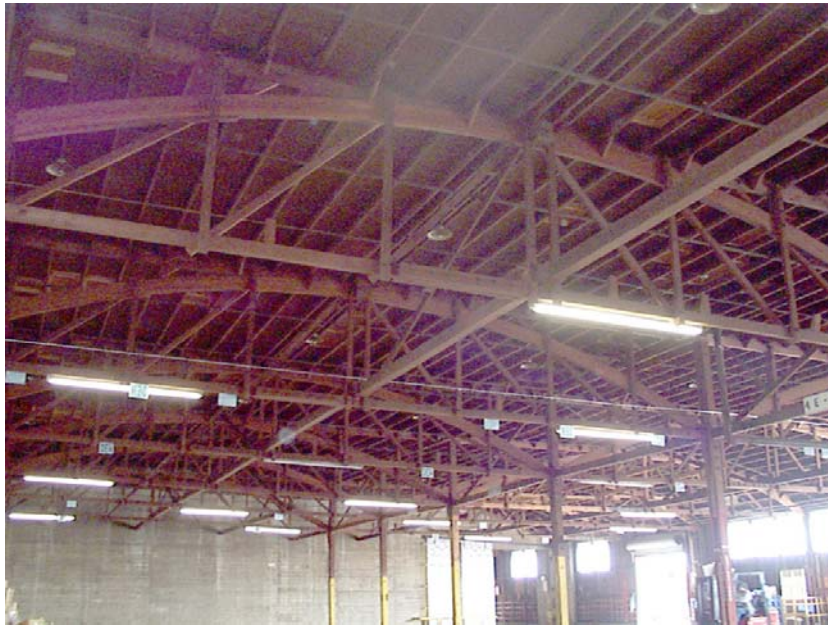
Looking northeast, inside building (warehouse) 16.
