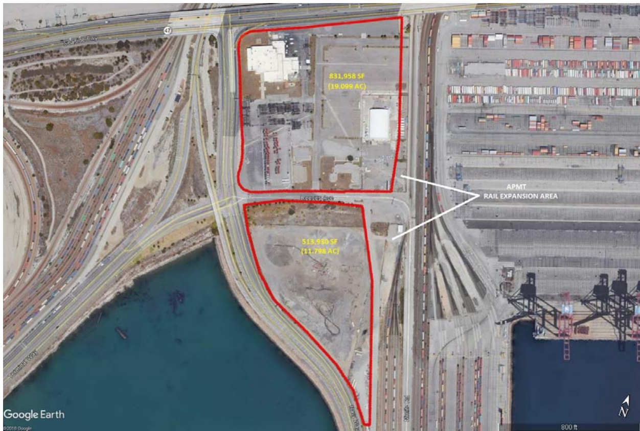
Figure 2 – Site Boundary: Pacific Crane Maintenance Company
