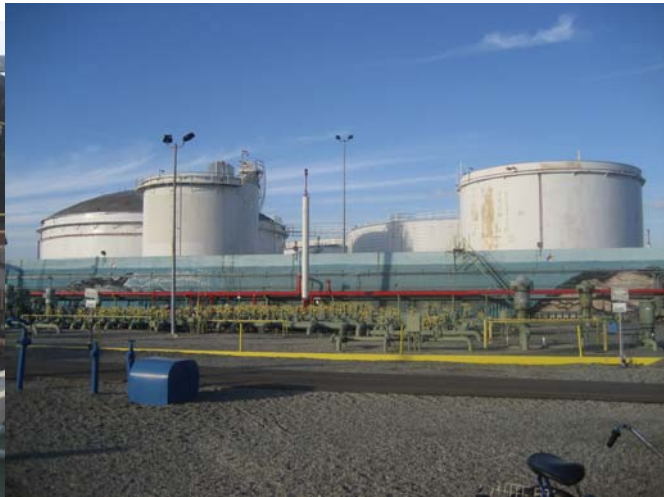
Tank Farm (background) and Valve Field (foreground)
