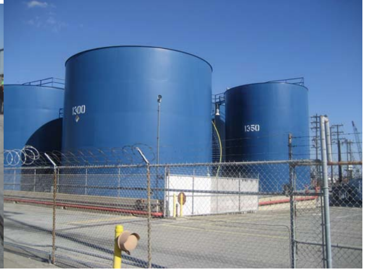
Tank Farm By Berth 188
