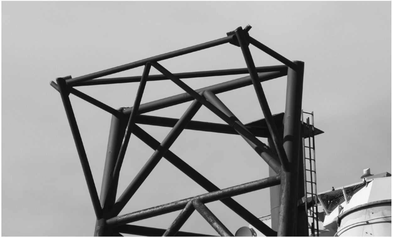
REMAINDER OF MAST AFTER PLATFORMS REMOVED
