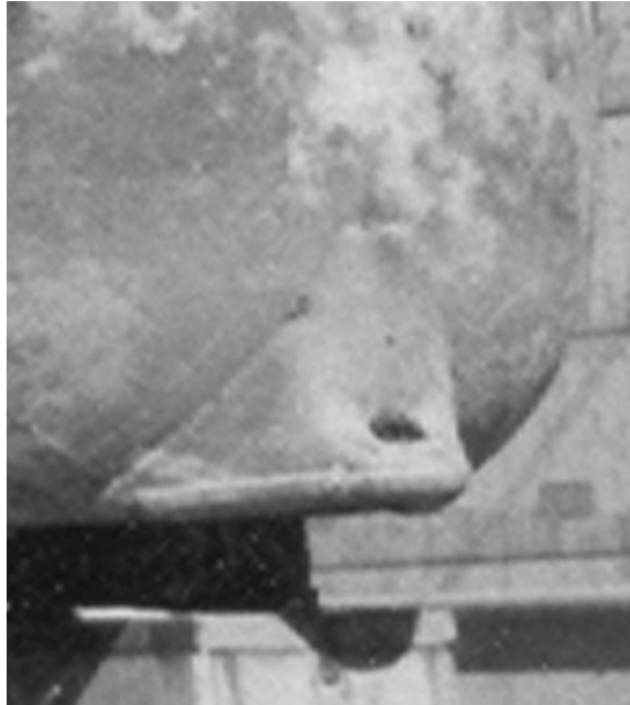
Close up of Forefoot Skeg/Paravane Eye that corroded inside the bellmouth and flooded the Forepeak tank.
