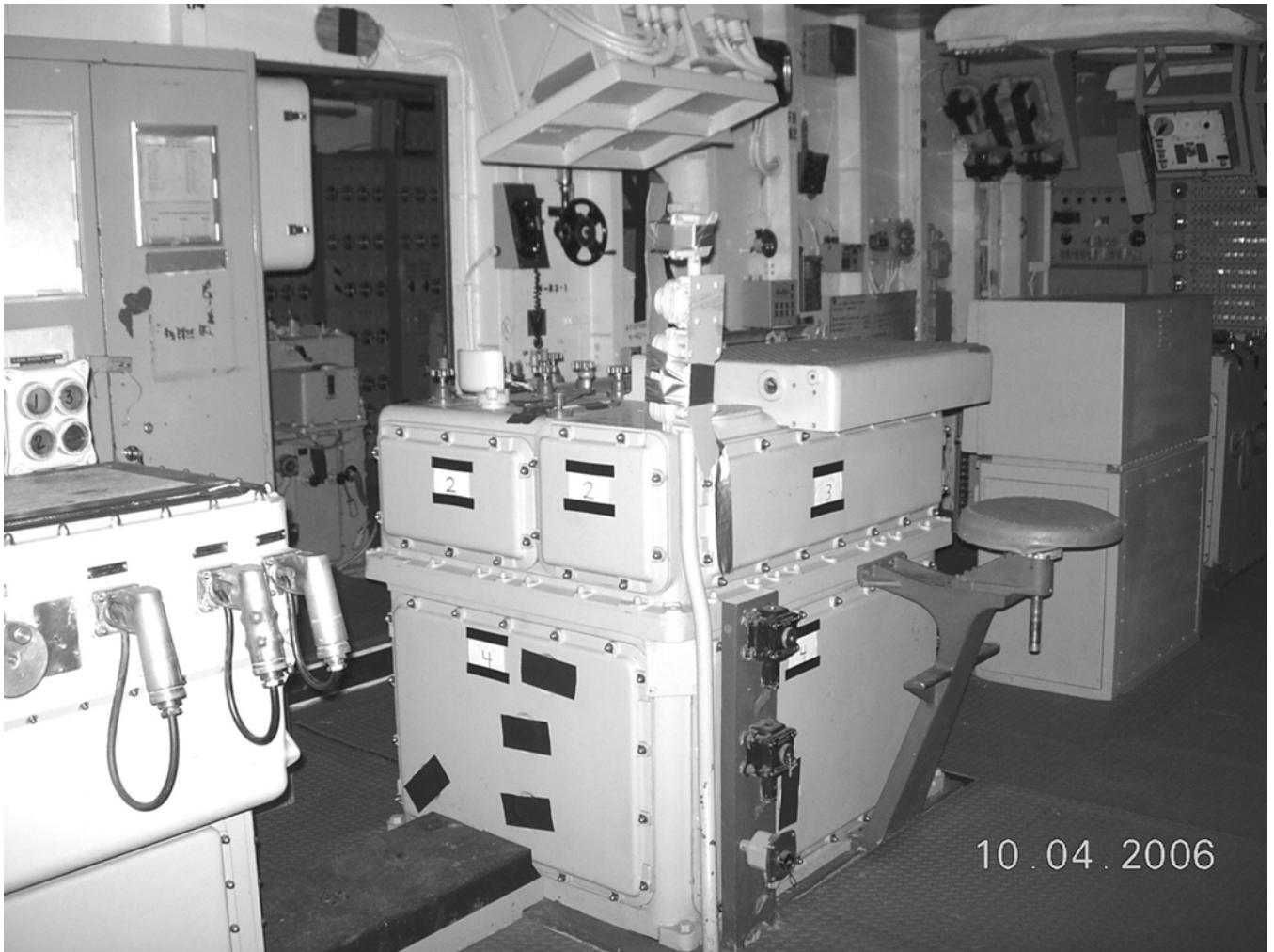
Mk-48 COMPUTER IN FWD MAIN BATTERY PLOT THAT CAN BE RELOCATED TO AFT MAIN BATTERY PLOT FOR VISITOR DISPLAY
