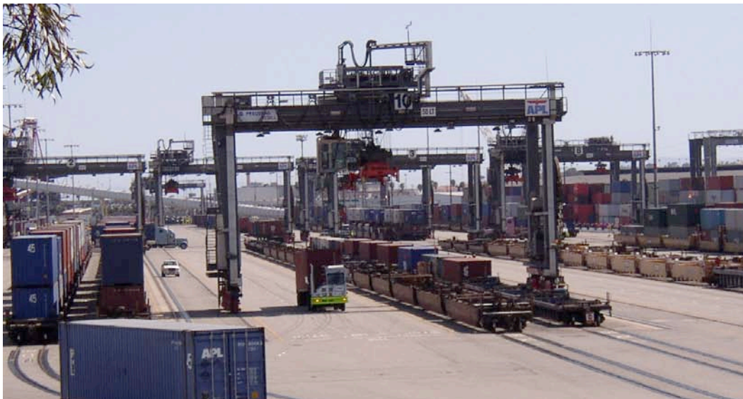
Image 1: Rail-mounted gantry (RMG) crane transferring container from yard hostler onto rail
