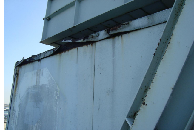
Exterior of Machinery House
