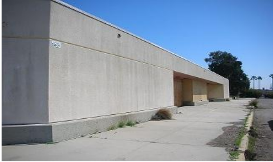
Figure 2-3 West Side of Navy Commissary Building 390 Navy Way
