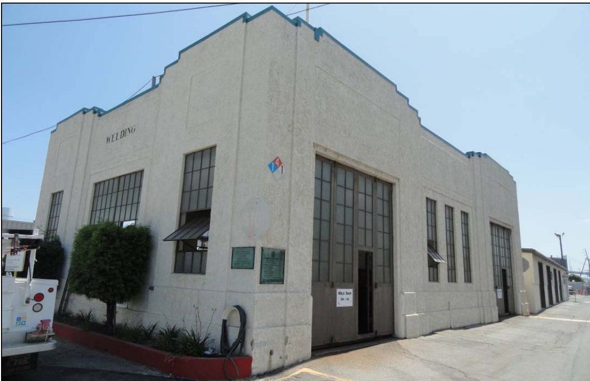
Figure 42 North and east facades of the blacksmith and welding shop, looking southwest (Applied EarthWorks, August 21, 2012).
