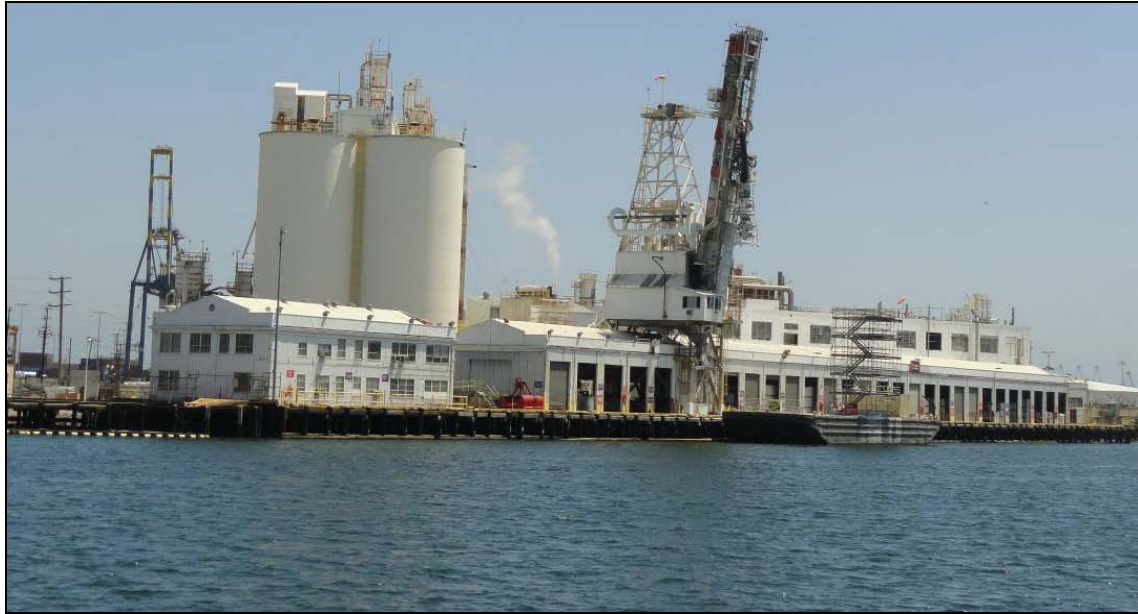
P5. Description of Photo: View looking View southeast at the Wharf Office, bulk storage bins/silos, warehouse, bulk ship loading conveyor, and the wharf at Berths 165–166.
