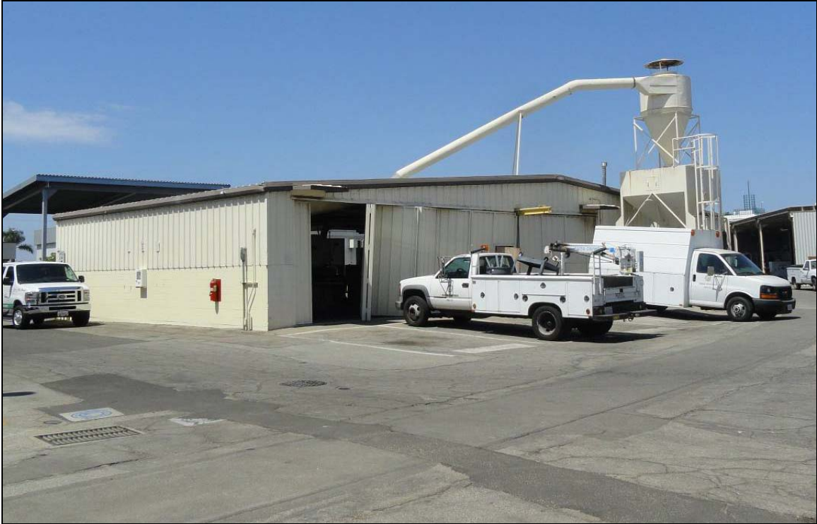
Figure 50 South and west facades of the cabinet shop and mill, looking northeast (Applied EarthWorks, August 21, 2012).
