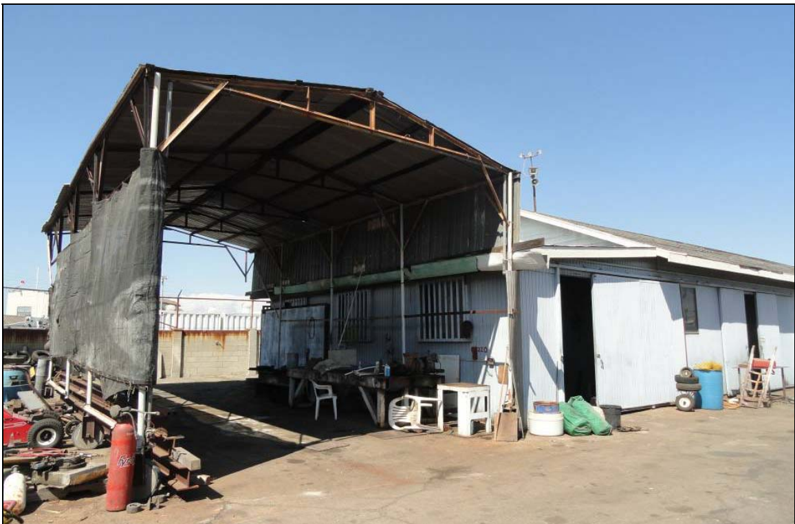
Figure 30 Pole shed adjacent to the shop addition, looking northeast (Applied EarthWorks, August 29, 2012).
