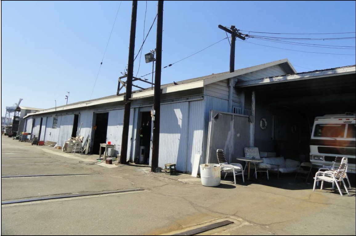
Figure 29 Shop 2, looking northwest (Applied EarthWorks, August 29, 2012).
