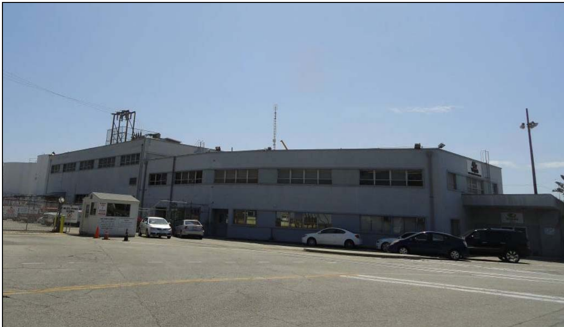
Figure 63 Vopak office building, looking southwest (Applied EarthWorks, Inc., August 21, 2012).
