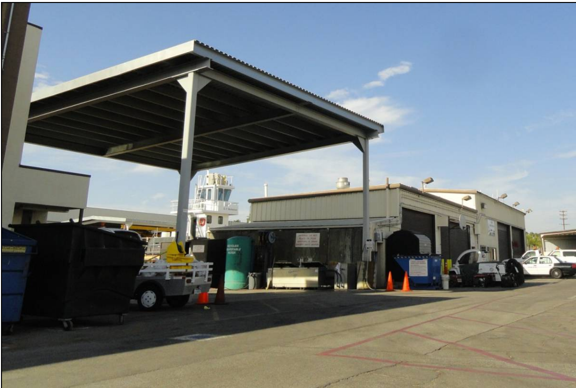
Figure 51 West and south facades of the auto repair garage and the new wash rack, looking northeast (Applied EarthWorks, October 5, 2012).
