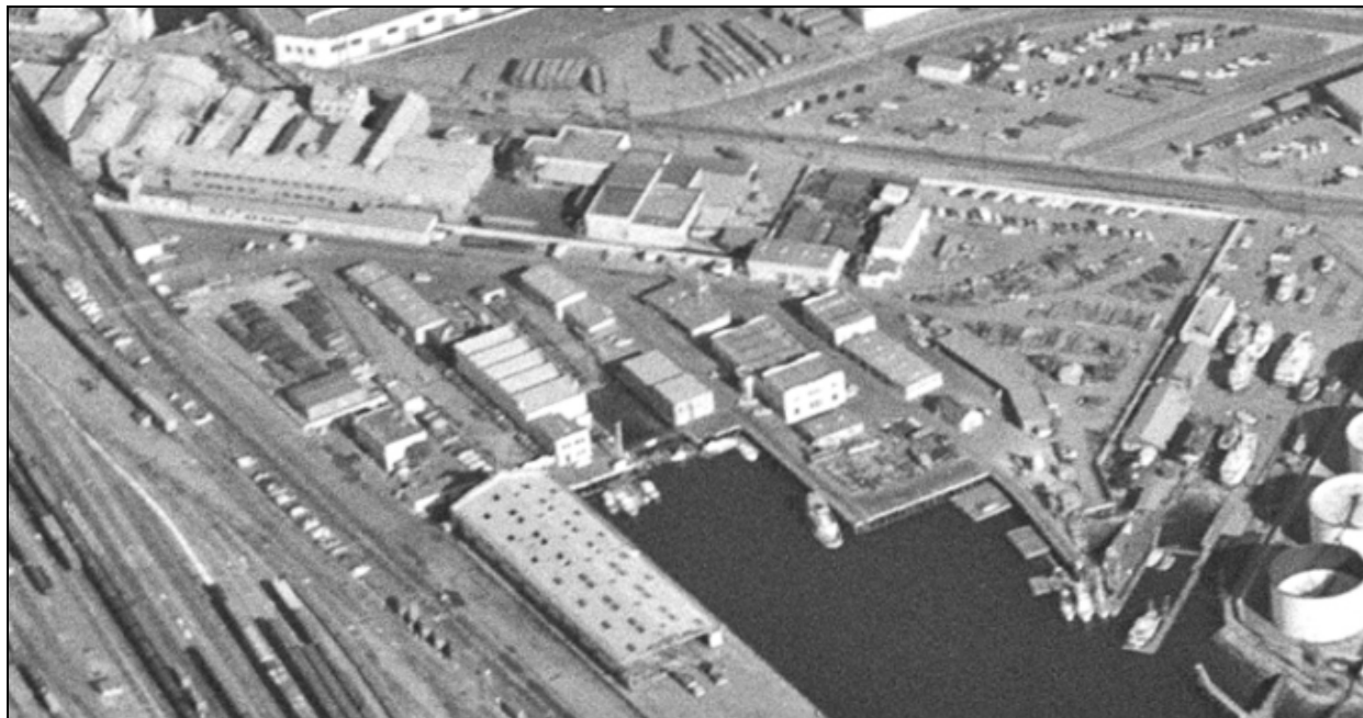
Figure 35 A bird's-eye view of the Harbor Department Construction and Maintenance Yard, looking east (LAHD Archives, November 29, 1971).
