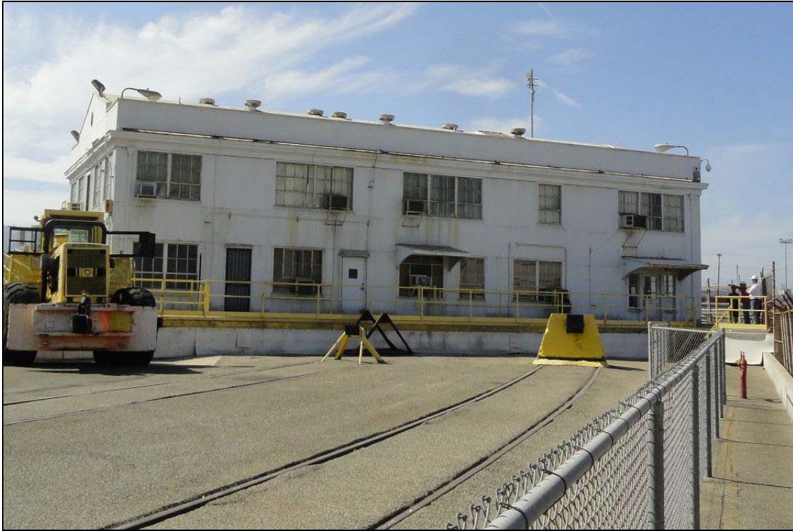
P5. Description of Photo: View looking west at the east façade of the wharf office.
