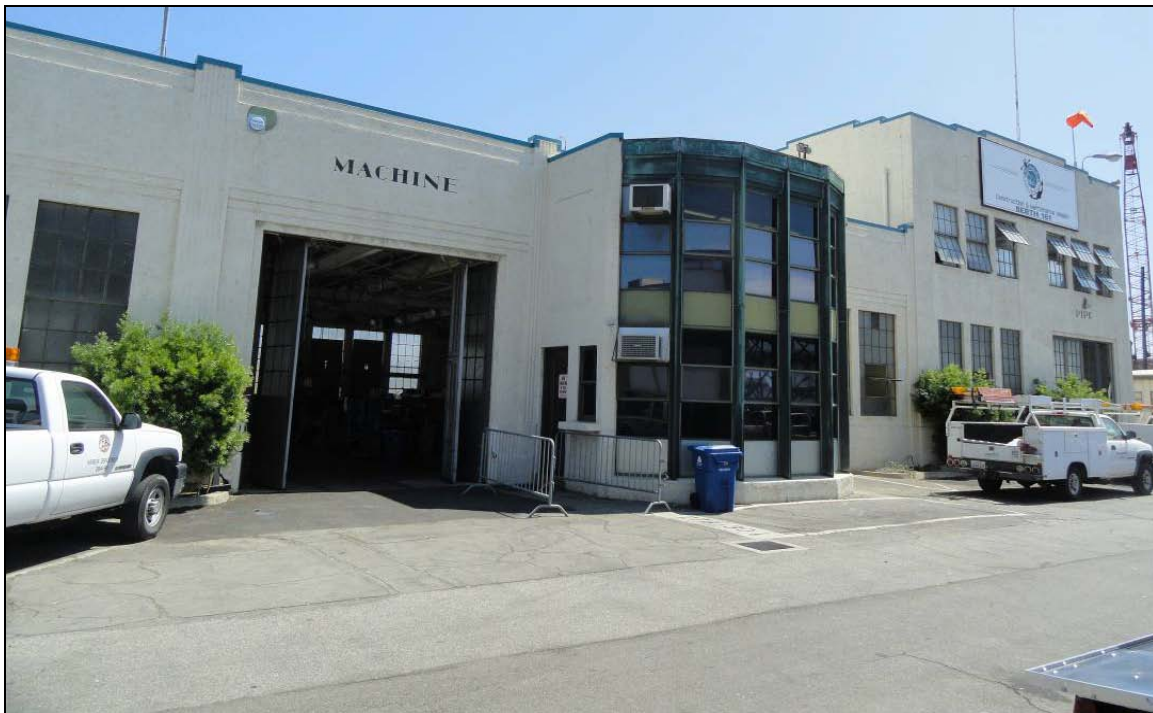
P5. Description of Photo: View looking southwest at the north facade of the Consolidated Shops.
