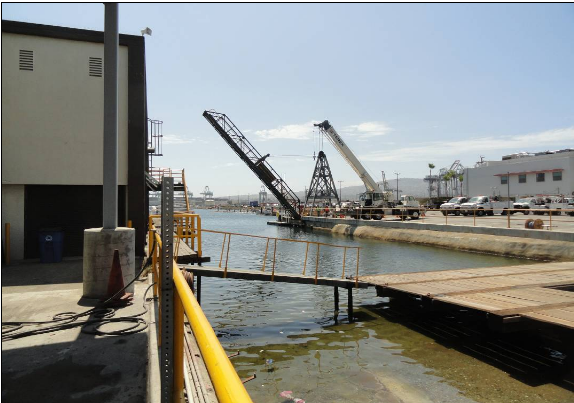
Figure 55 Drawbridge, looking northwest (Applied EarthWorks, August 21, 2012).
