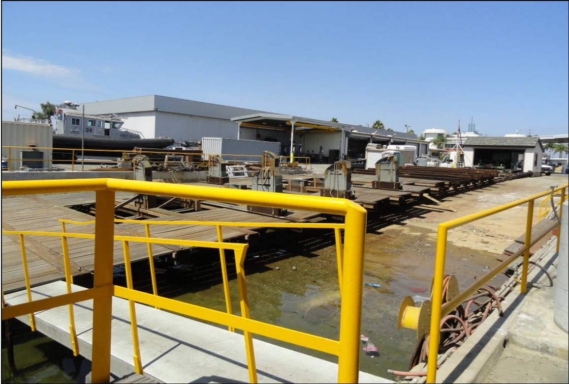
Figure 54 Winch house and rail car, looking northeast (Applied EarthWorks, August 21, 2012).
