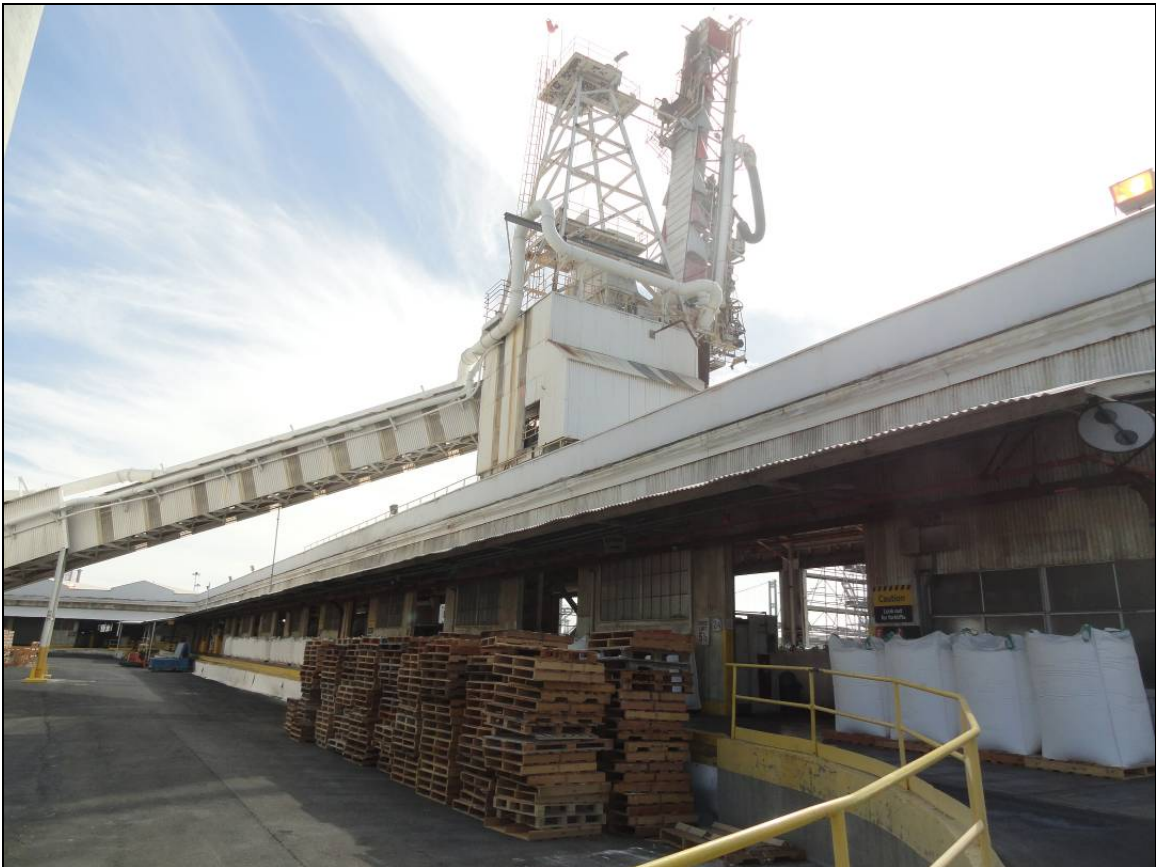
Figure 22 Bulk ship loading conveyor, looking south, with north facade of the connecting shed in the far left background (Applied EarthWorks, October 5, 2012)
