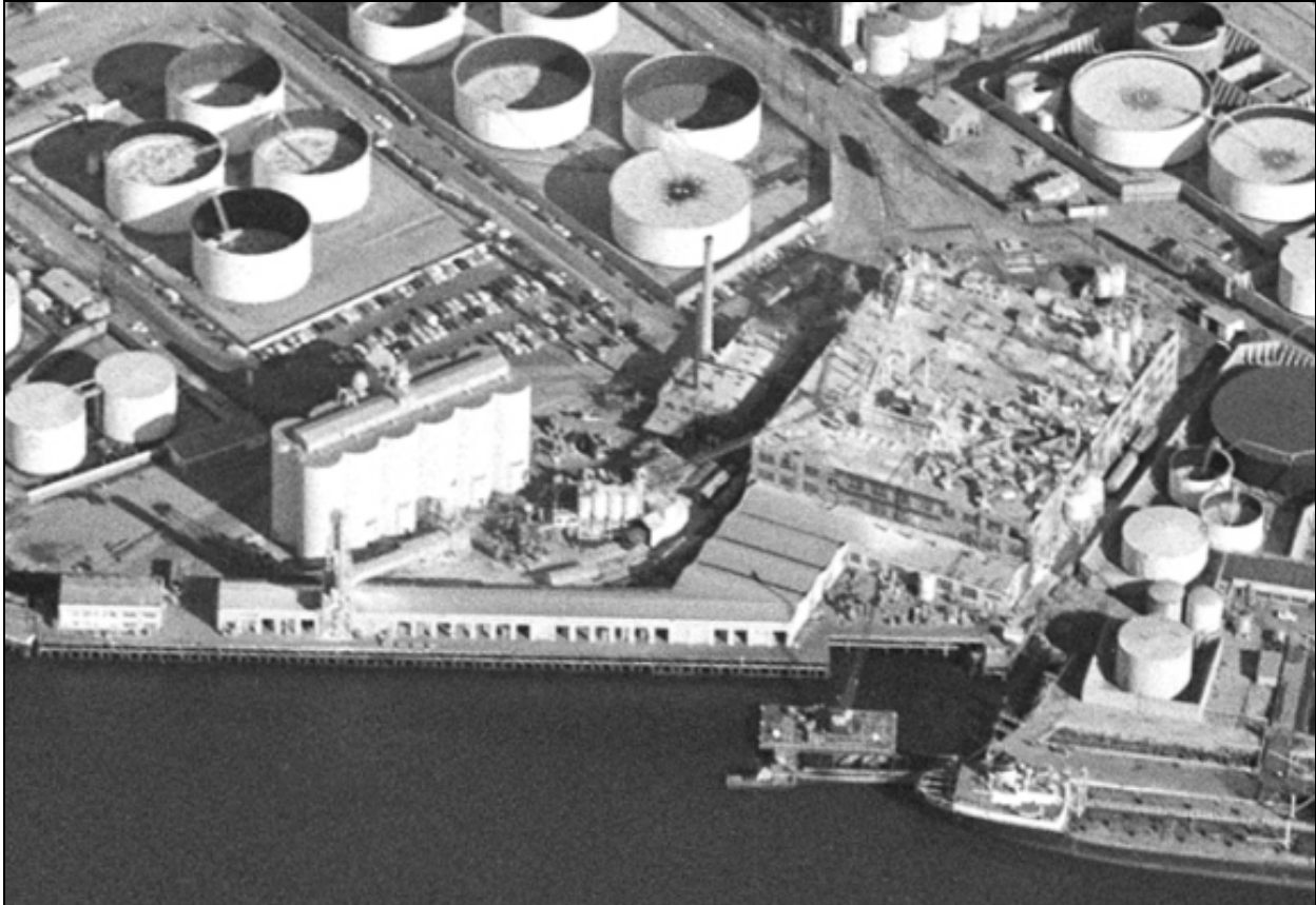
Figure 12 A bird’s-eye view of the Borax Plant, looking east (LAHD Archives, November 29, 1971).
