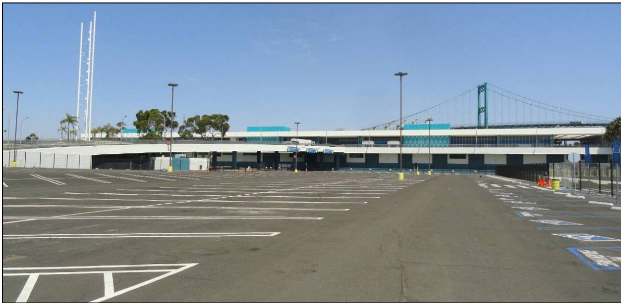
Figure 4 Overview of the eastern portion of the southwest elevation of the Los Angeles Cruise Terminal, looking northeast (Applied EarthWorks, August 21, 2012).
