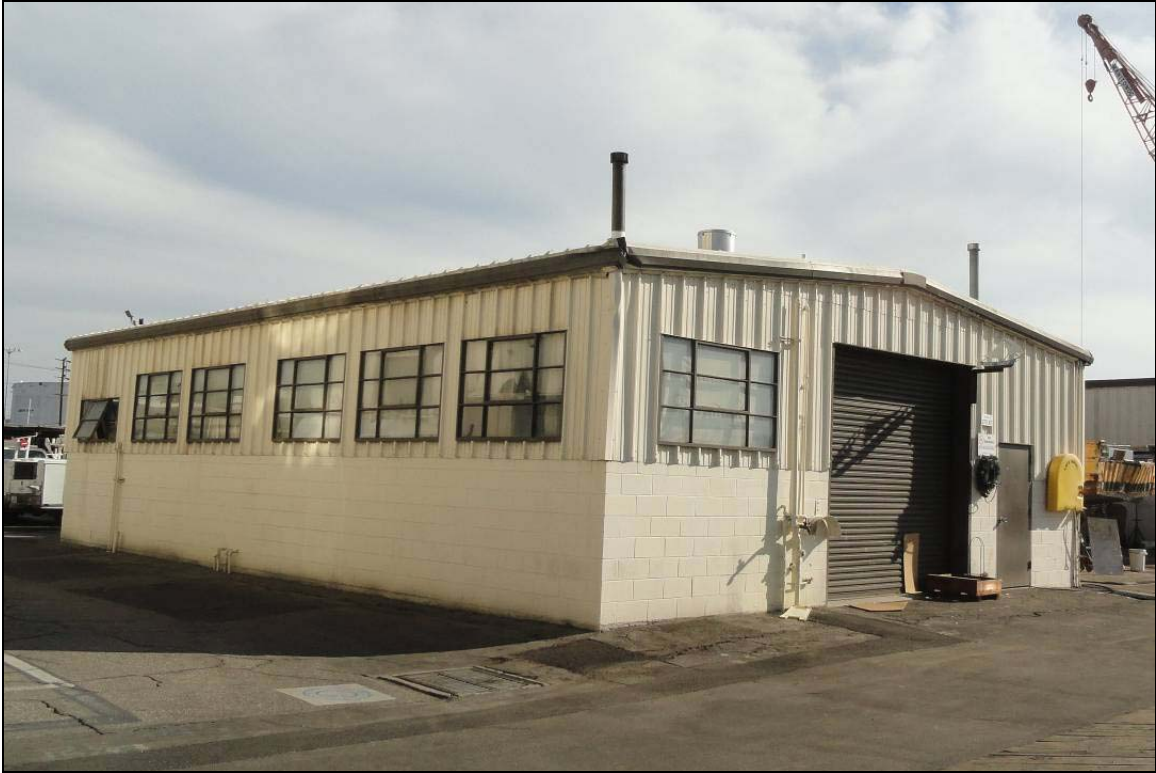
Figure 48 North and east facades of the boat shop, looking southwest (Applied EarthWorks, October 5, 2012).
