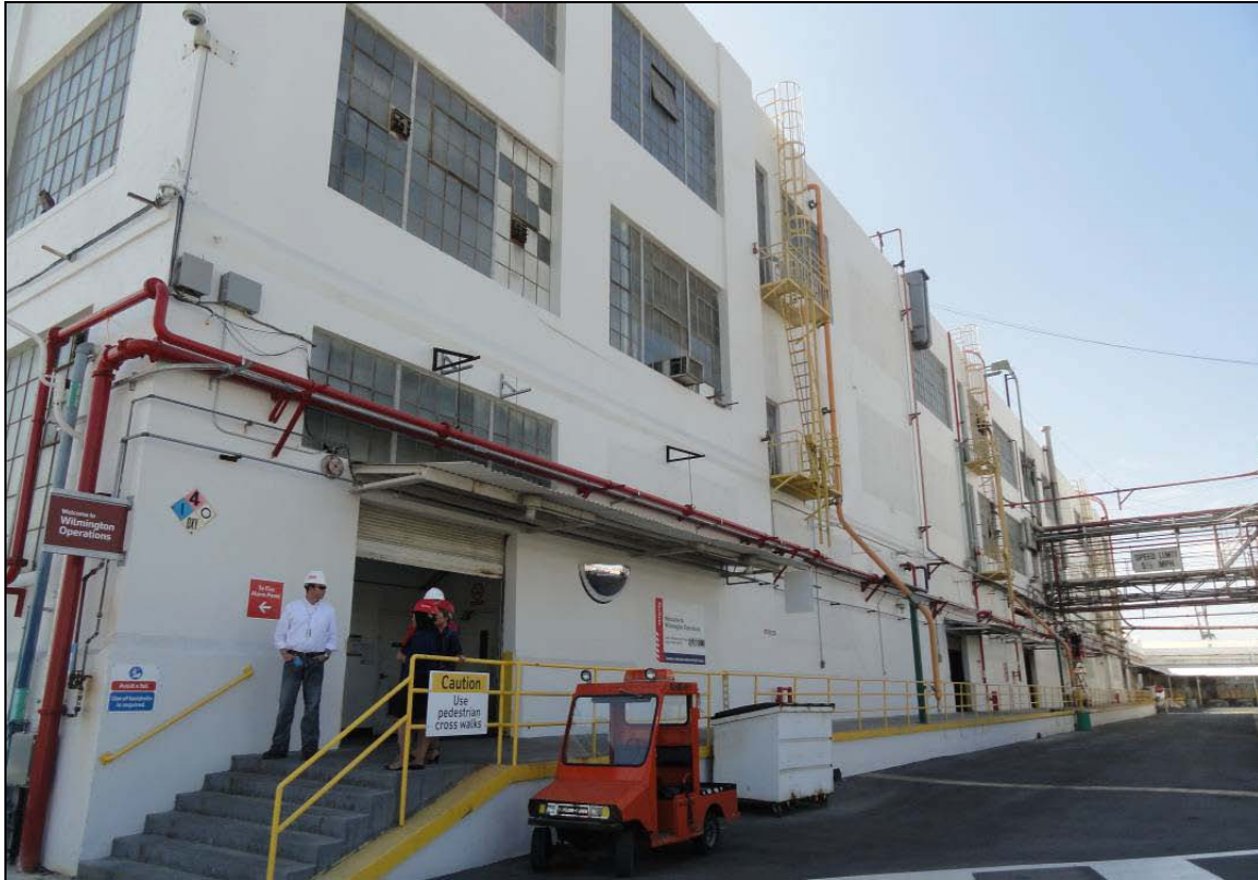
P5. Description of Photo: View looking west at the north façade of the refinery building.
