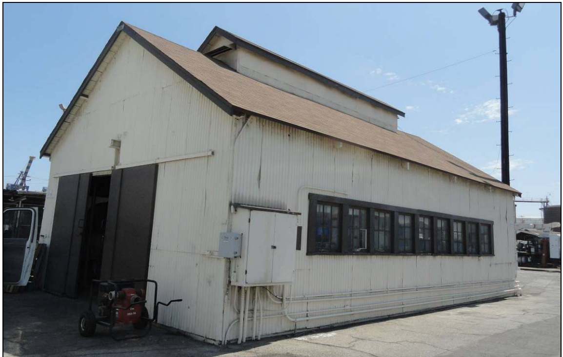
Figure 38 North and east facades of the paint shop, looking south (Applied EarthWorks, August 21, 2012).
