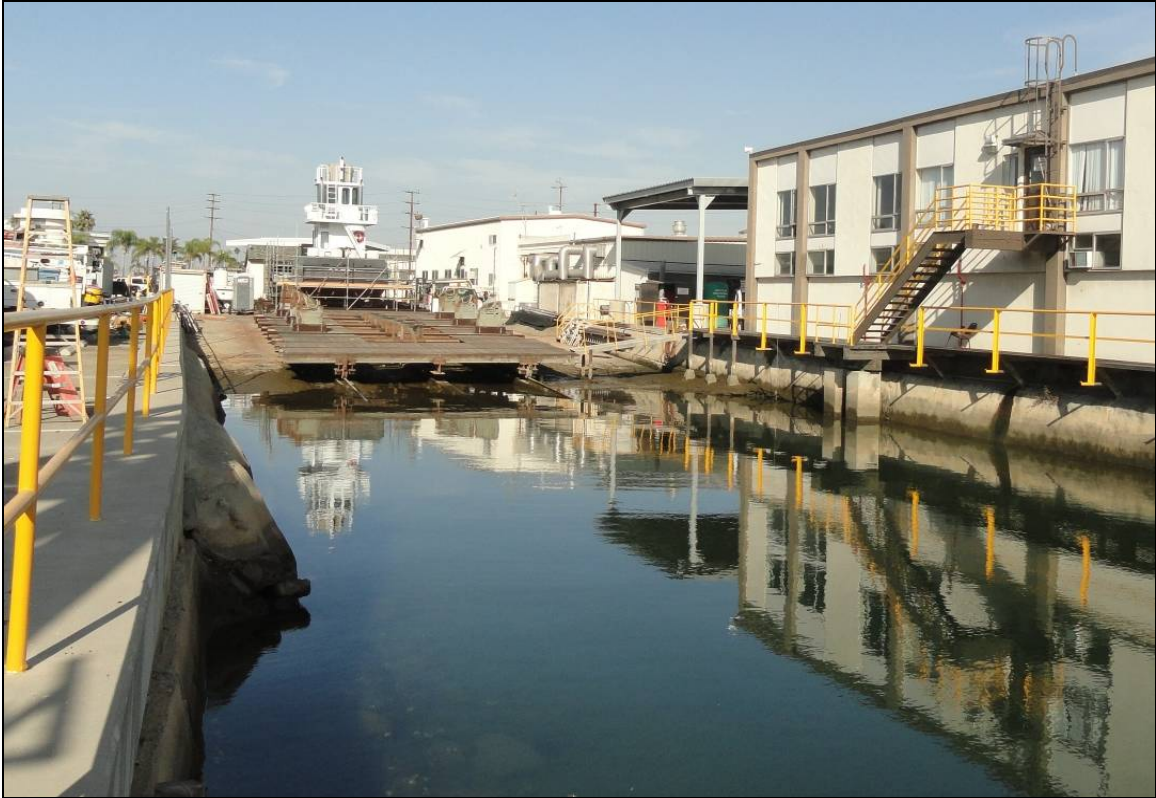
Figure 53 Marine ways and rail car, looking east (Applied EarthWorks, October 5, 2012).
