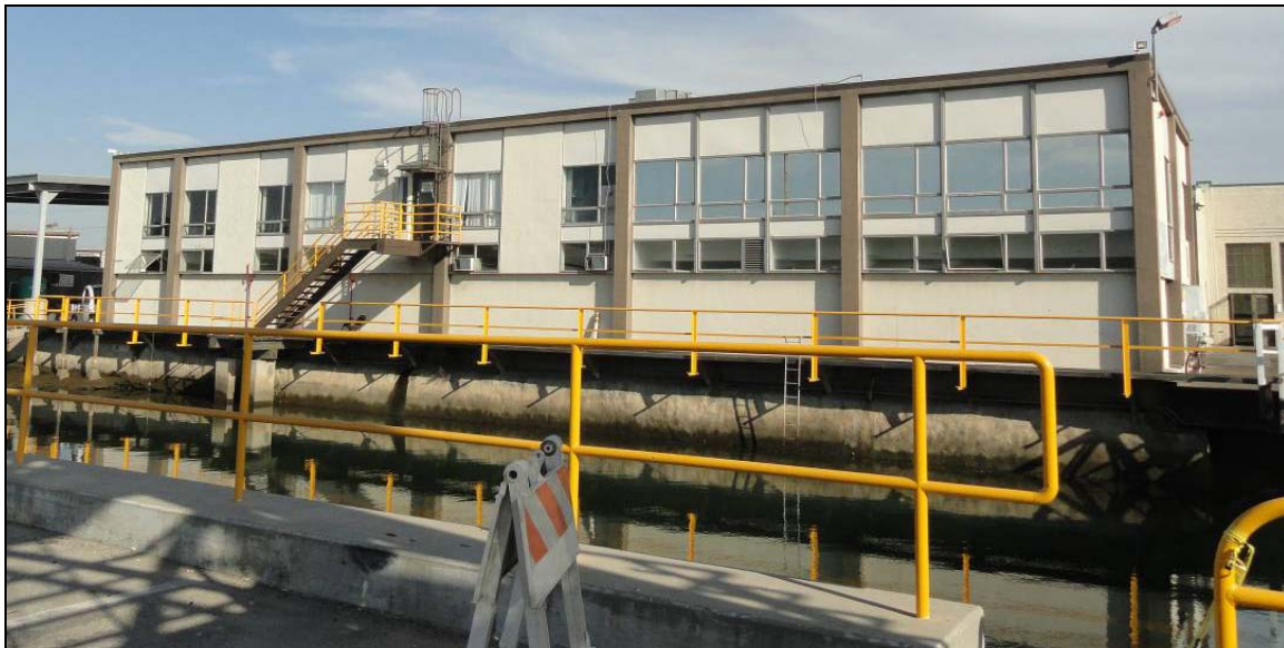
Figure 44 North facade of the service building, looking south (Applied EarthWorks, October 5, 2012).
