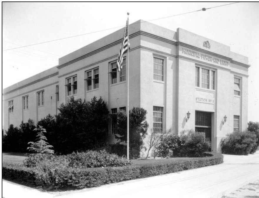
Figure 6 North and west facades of Distribution Station No. 3, looking east (courtesy, Historical Photo Collection of the Department of Water and Power, City of Los Angeles).
