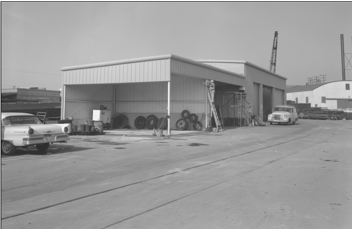
Figure 52 West and south facades of the auto repair garage, looking northeast (LAHD Archives, January 26, 1962).
