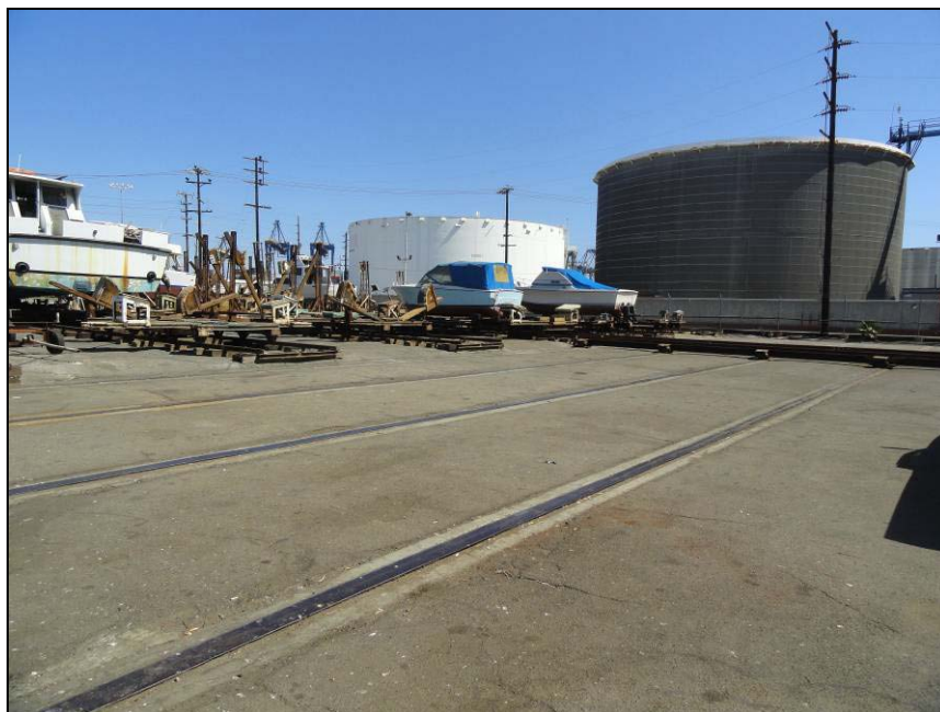
P5d. Description of Photo: View looking southeast at the marine rail lines and sliding connector.
