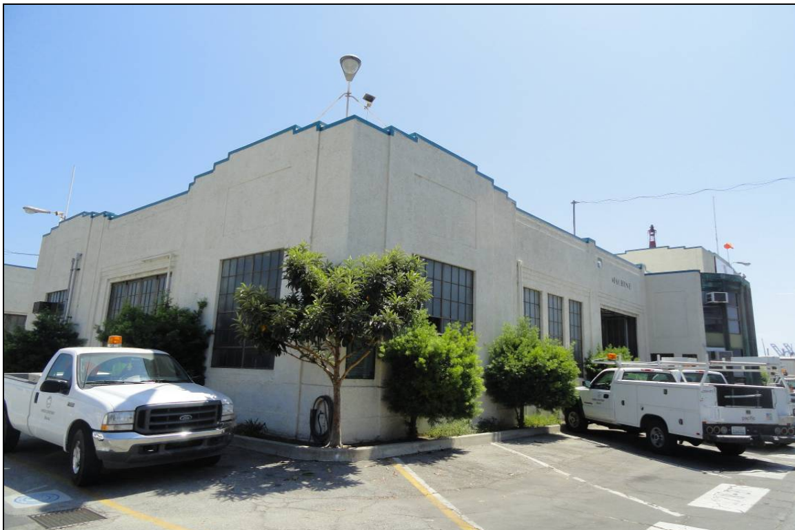
Figure 41 North and east facades of the consolidated shops, looking southwest (Applied EarthWorks, August 21, 2012).
