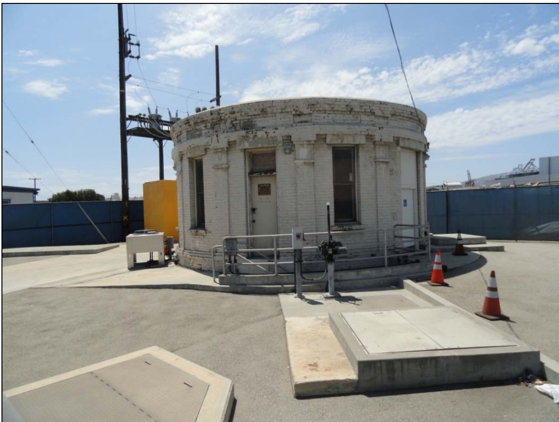
Figure 59 Mormon Island Sewage Plant, looking southwest. The entrance in the center of the photo is original, while the entrance to the right (with the handicap sign) was cut into the building sometime before 1988. An underground passage was added sometime after 1988. In the past the plant grounds were landscaped but are now covered by asphalt and concrete (Applied EarthWorks, August 21, 2012).
