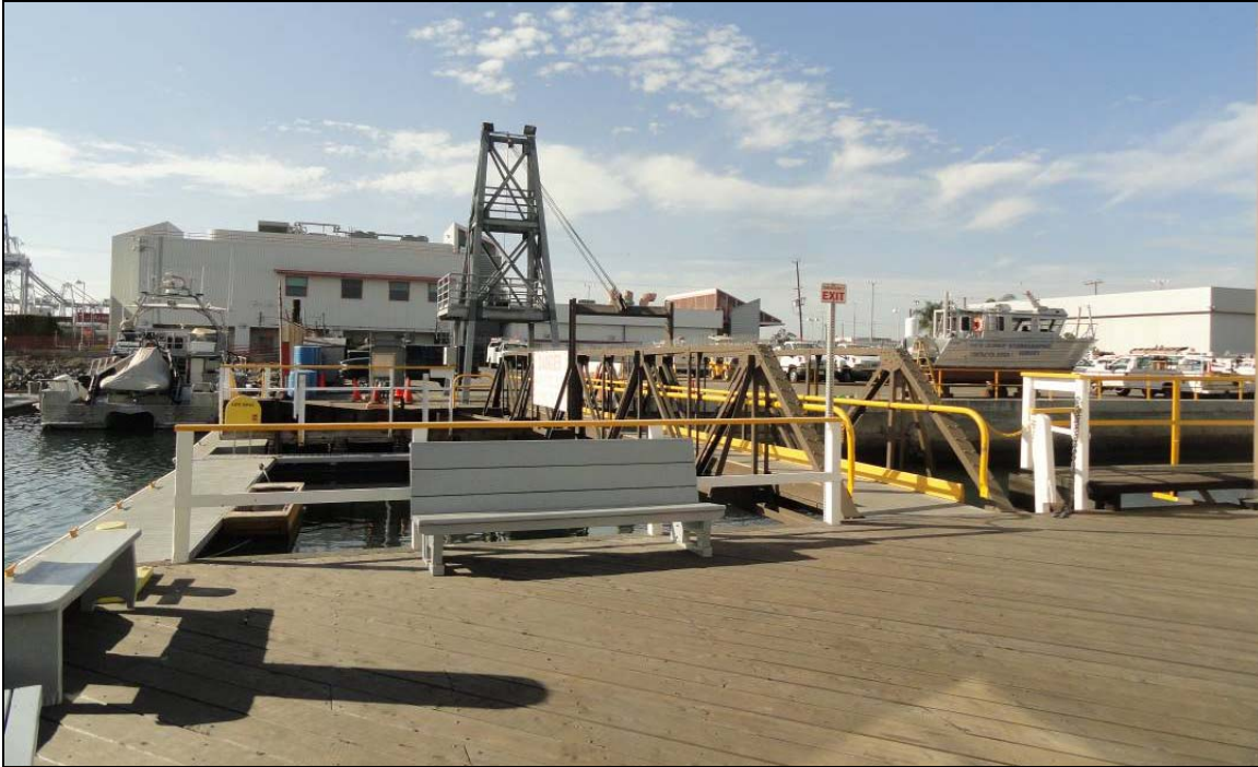
Figure 56 Drawbridge and tower, looking north (Applied EarthWorks, October 5, 2012).
