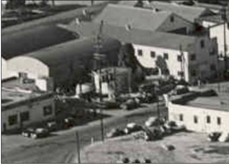
Figure 57 Detail view looking northwest at the pump house and surroundings (LAHD Archives, Spence Air Photos, December 14, 1948).
