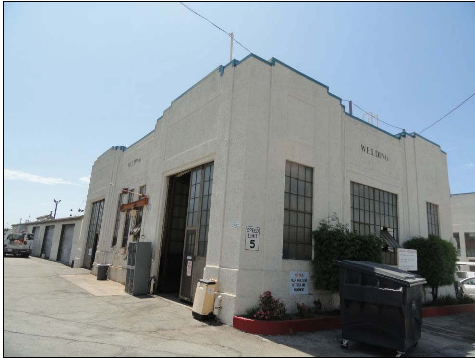
P5. Description of Photo: View looking west at the south and east façades of the Blacksmith and Welding Shop
