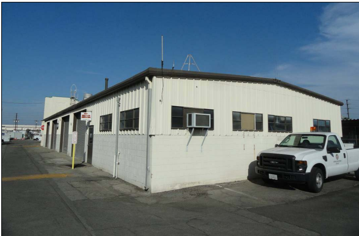
Figure 46 North and west facades of the electric shop, looking east (Applied EarthWorks, October 5, 2012).
