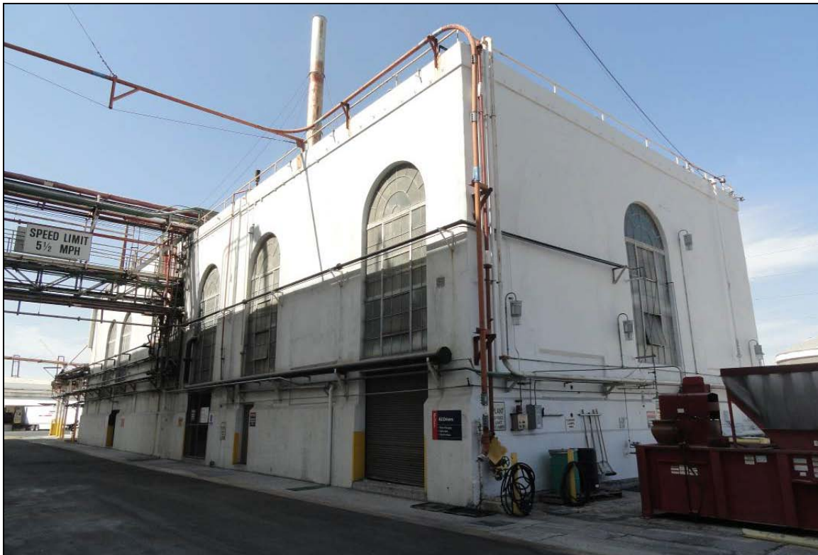
P5. Description of Photo: View looking northwest at the south and east façades of the steam plant and air compressor room.
