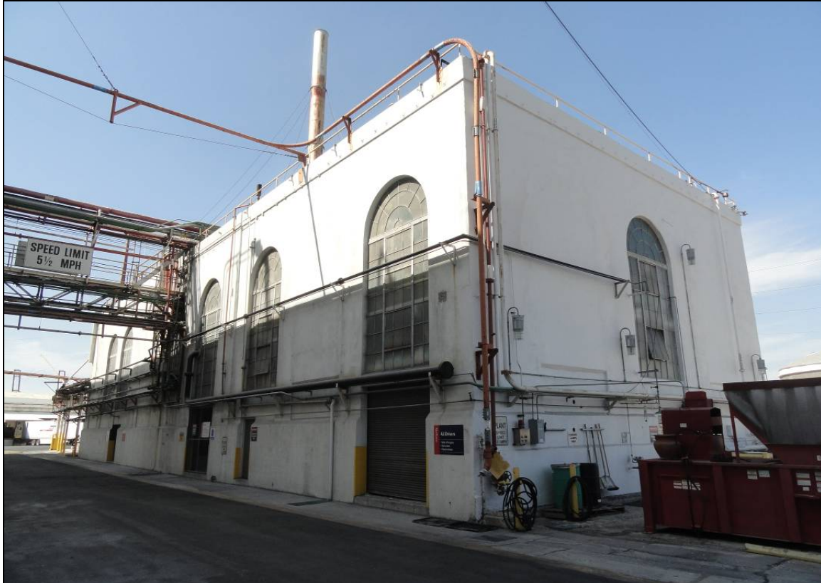
Figure 15 South and east facades of the steam plant and air compressor room, looking northwest (Applied EarthWorks, October 5, 2012).
