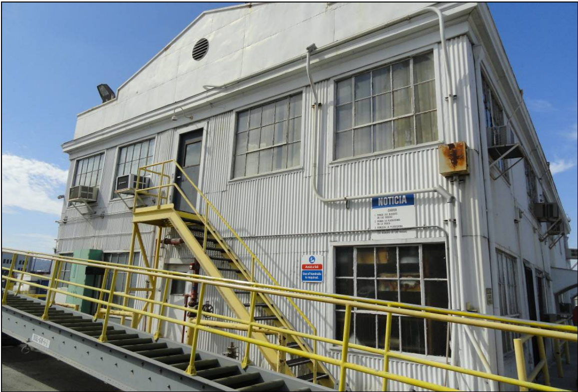
Figure 17 South facade of the wharf office, looking north (Applied EarthWorks, October 5, 2012).
