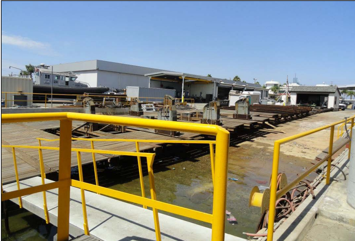
P5. Description of Photo: View looking northeast at the Winch house and rail car.
