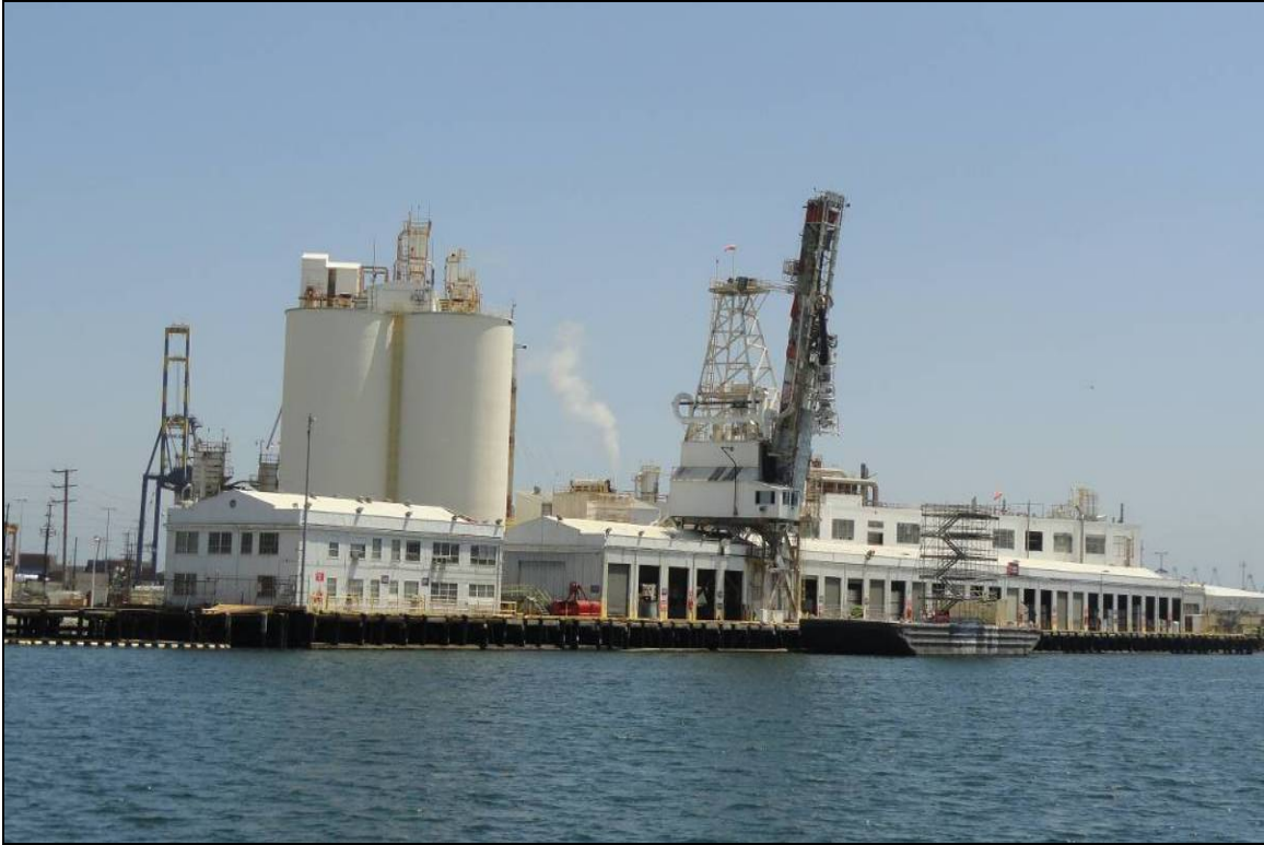
Figure 23 Wharf office, bulk storage bins/silos, warehouse, bulk ship loading conveyor, and the wharf at Berths 165–166, looking southeast (Applied EarthWorks, August 21, 2012).
