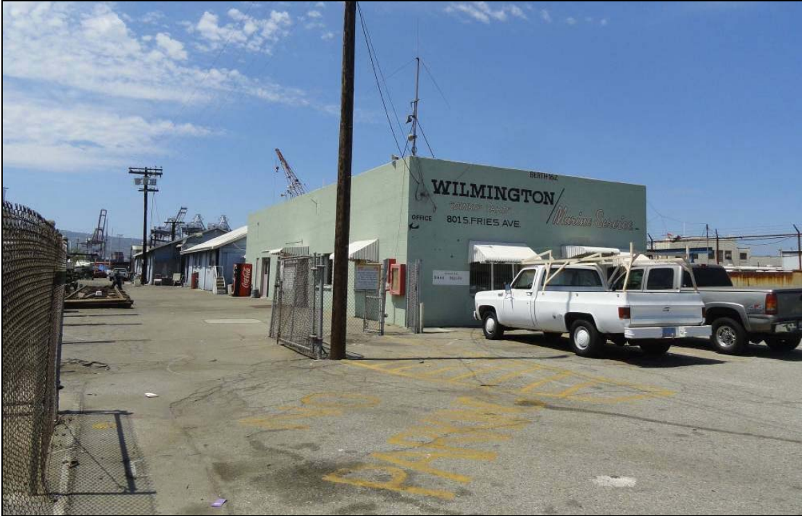
Figure 27 Wilmington Marine Service office and shops, looking west (Applied EarthWorks, August 21, 2012).
