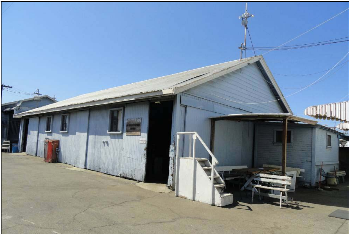
Figure 28 Shop 1, looking northwest (Applied EarthWorks, August 29, 2012).
