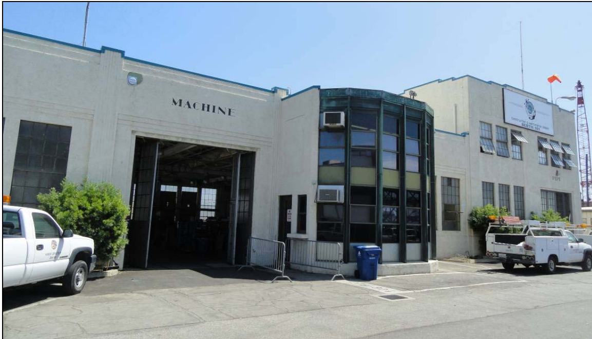
Figure 40 North facade of the consolidated shops, looking southwest (Applied EarthWorks, August 21, 2012).
