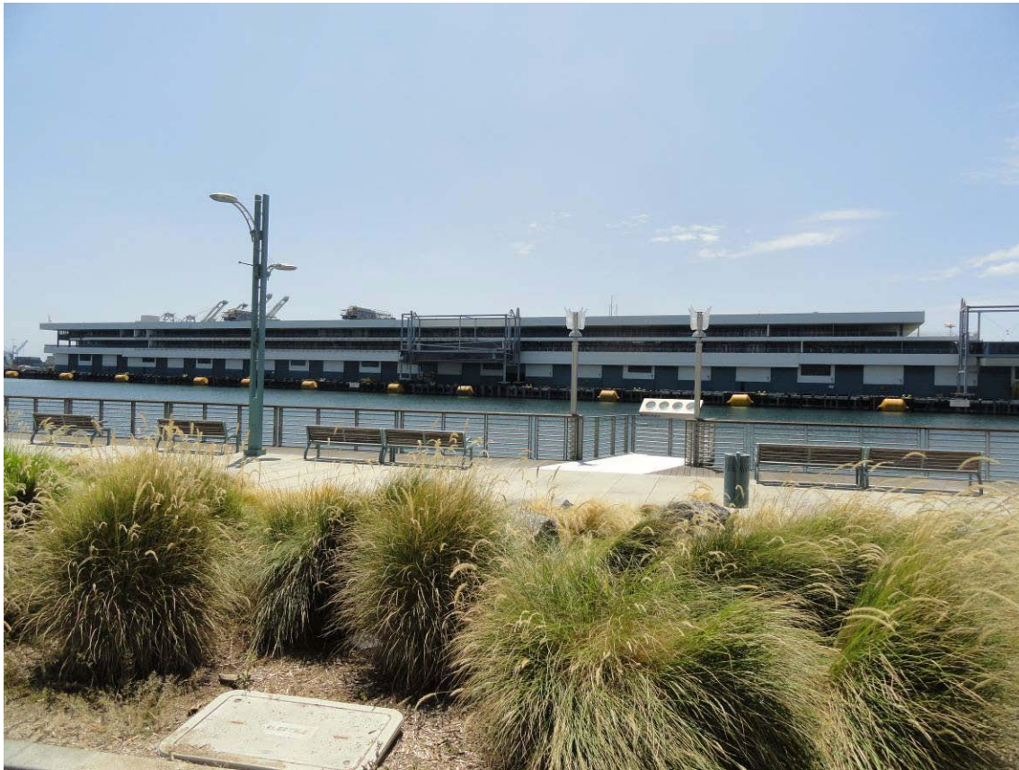
P5c. Description of Photo: View looking west at the northeast facing rear facade.
