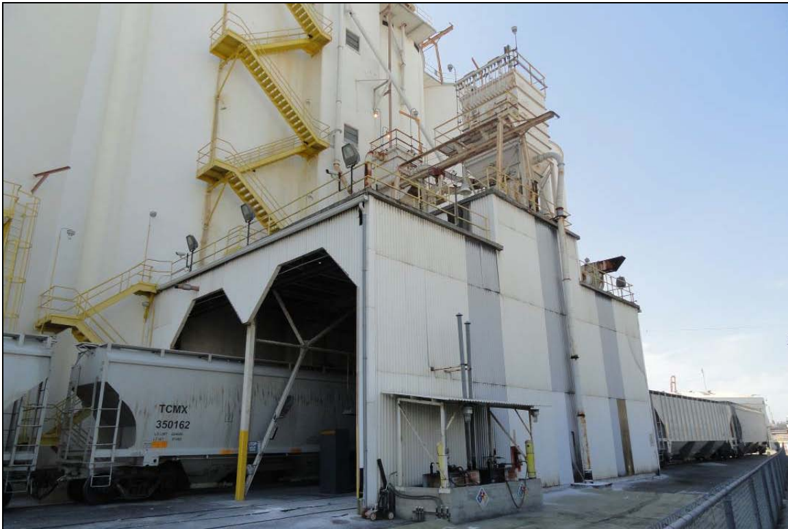
P5. Description of Photo: View looking west at the east side of the unloading shed.
