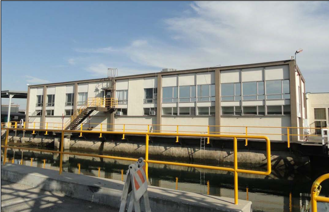
P5. Description of Photo: View looking south at the north facade of the Service Building.
