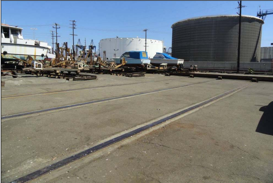
Figure 34 Marine rail lines and sliding connector, looking southeast (Applied EarthWorks, August 29, 2012).
