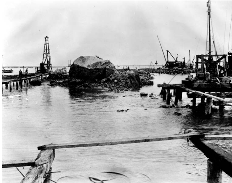
1 2 3 4 5 6 7 8 9 10 11 12 13 14 15 16 17 18 19 20 21 22 23 Photograph 3.4-1: Demolition of Dead Man's Island, dredging and infilling to create Terminal Island ca. 1920 (Los Angeles Water and Power Associates Photo Archive)
