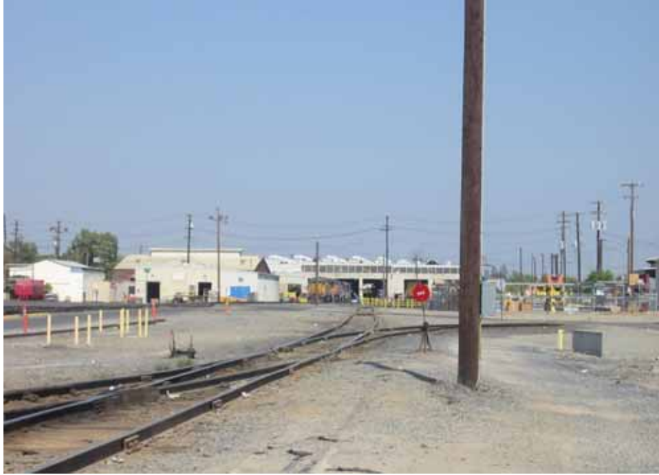
Figure 33. Diagnostics Area of Diesel Shop
