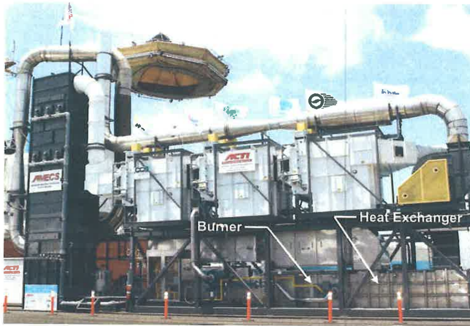
Figure 10. ETS: SCR Heat Management System
