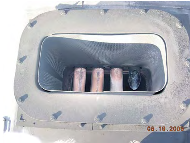
Figure 4: View into the Dash 8 exhaust stack, showing the crankcase vent and air filter suction tubes
