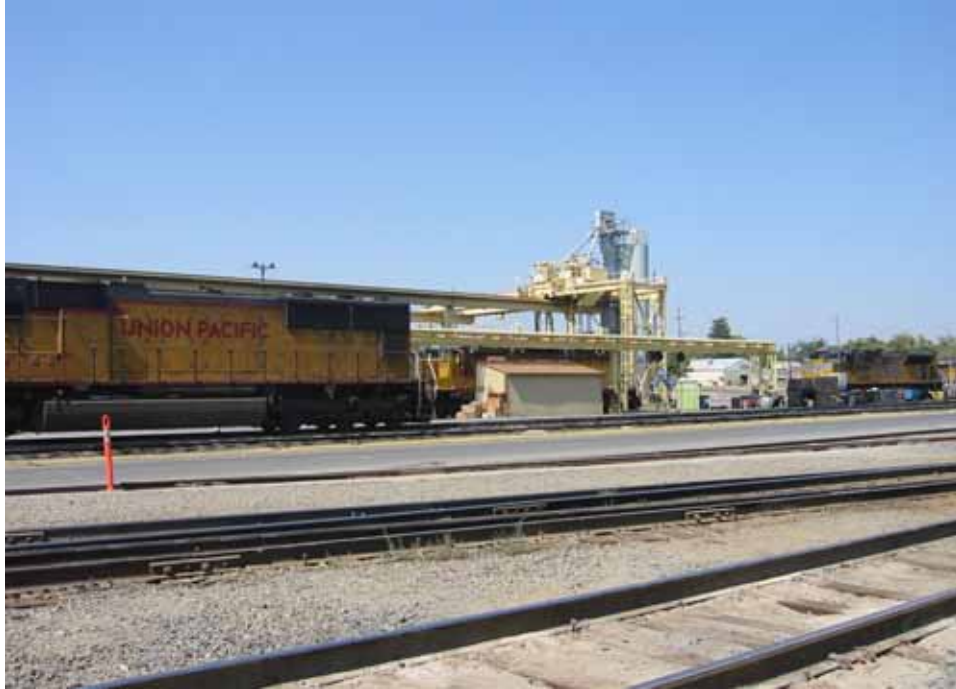
Figure 35. Sanding Stations
