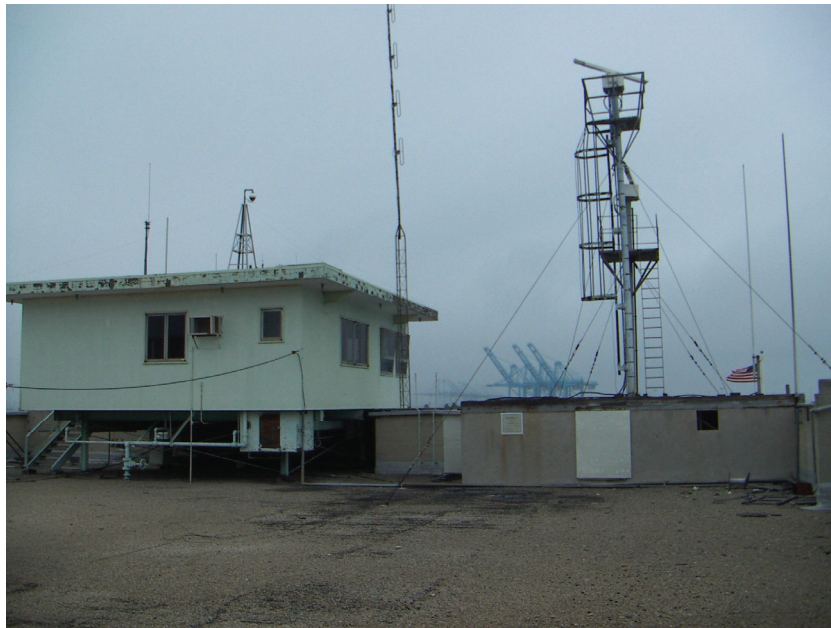
Figure 21 – Harbor Office and Equipment Penthouse on Roof
