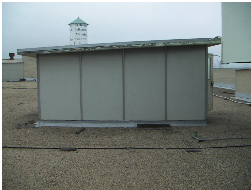
Figure 23 – Stair Penthouse on Roof
