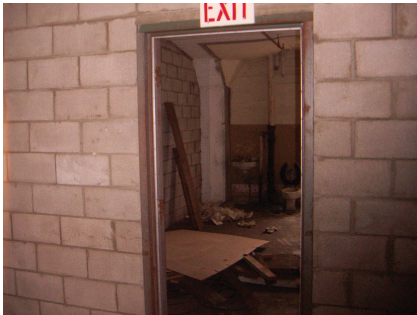
Figure 14 – CMU Infill Wall at Second Floor Restroom
