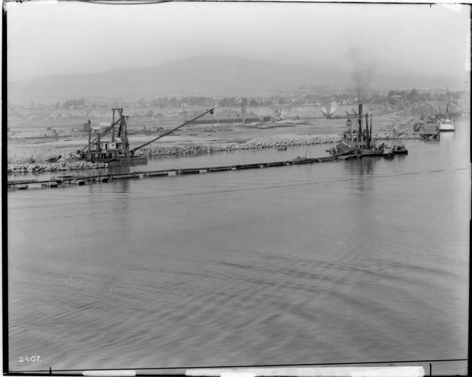
Figure 5 Dredgers at Work on the “Huntington Fill,” circa 1913
