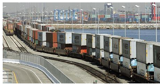
Photograph 4. The Port's rail infrastructure consists of more than 65 miles of on-dock track for building and sorting double-stack trains. The average train is made up of 30 double-stack cars, eliminating approximately 400 truck trips and related air pollution while optimizing the movement of cargo.
