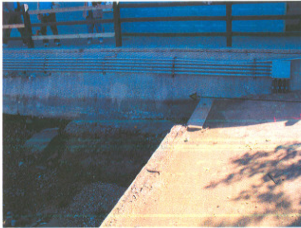
Adjacent Concrete Bulkhead
