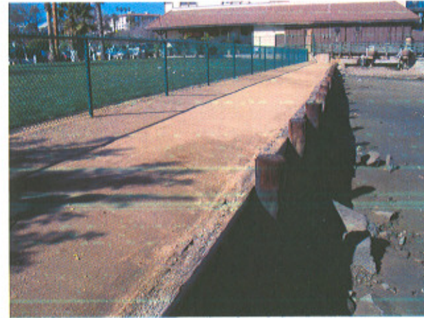
Existing Wooden Bulkhead
