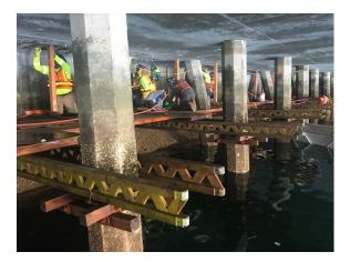
Berths 226-236, Everport Container Terminal Improvements Construction continues at this terminal to deepen berths and improve terminal facilities to accommodate larger next-generation vessels. The project involves improvements at Berths 226-229, increasing berth depth from -45 to -53 feet, and improving Berths 230-232 to a -47 feet berth depth. The project also involves constructing an additional 1.5 acres of backland and electrical
