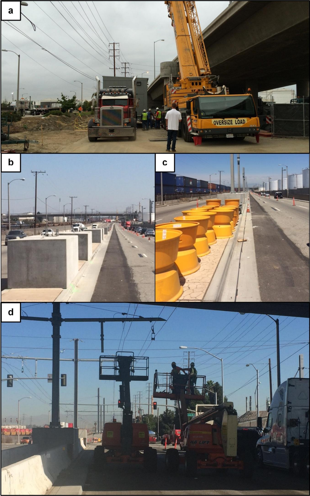
Figure 18 Construction phase – setting of foundations and poles
