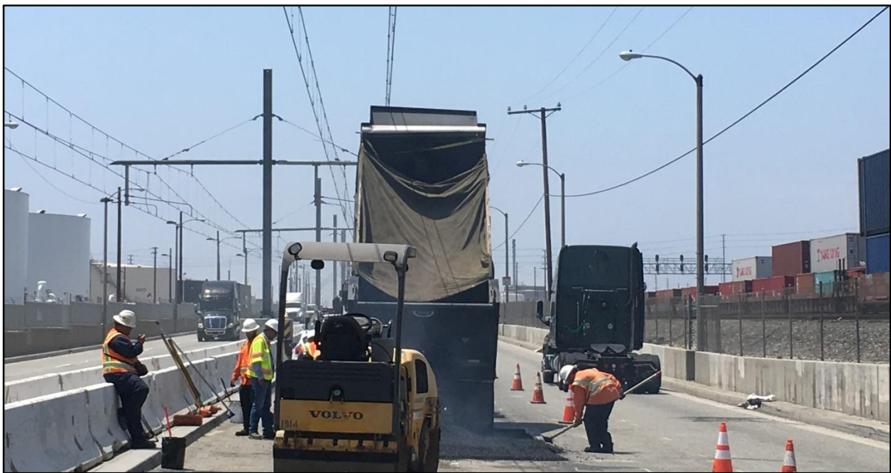
Figure 30 Road works with machinery in the vicinity of the contact line
