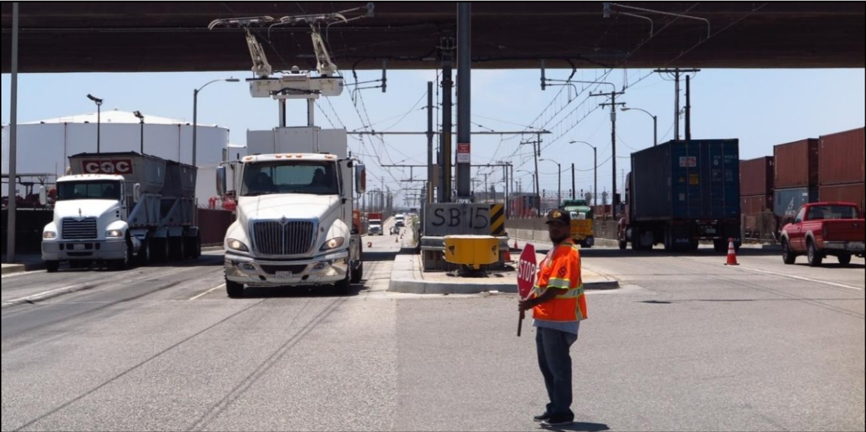
Figure 27 Traffic management in place in both directions
