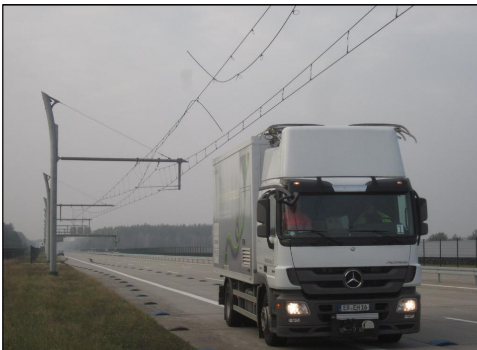
Figure 28 Reduced dropper spacing prevent broken wires from falling to ground
