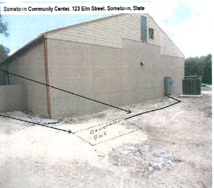
Figure 4. Ground-level photograph showing proposed ground disturbance area.
