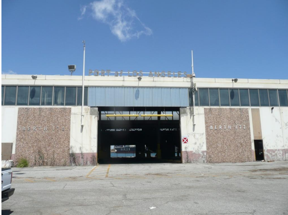
Figure 2-4a. Primary Entrance, West Side of Transit Shed
