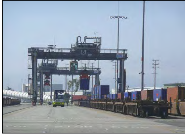
5 6 Photograph 9: Rail-mounted gantry crane at the existing on-dock railyard
