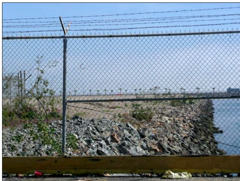
20 21 Photograph 2: Area of new wharf along Berth 306
