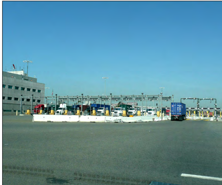
Photograph 7: Existing in-gate and out-gate
