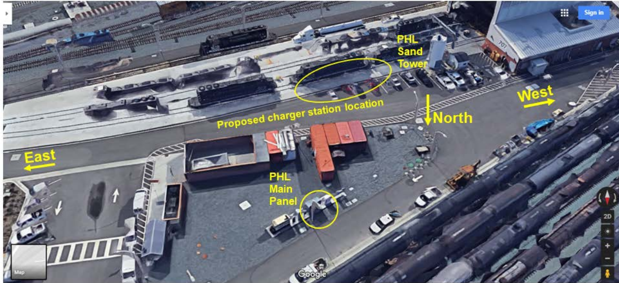
Location of PHL locomotive facility and main power panel
