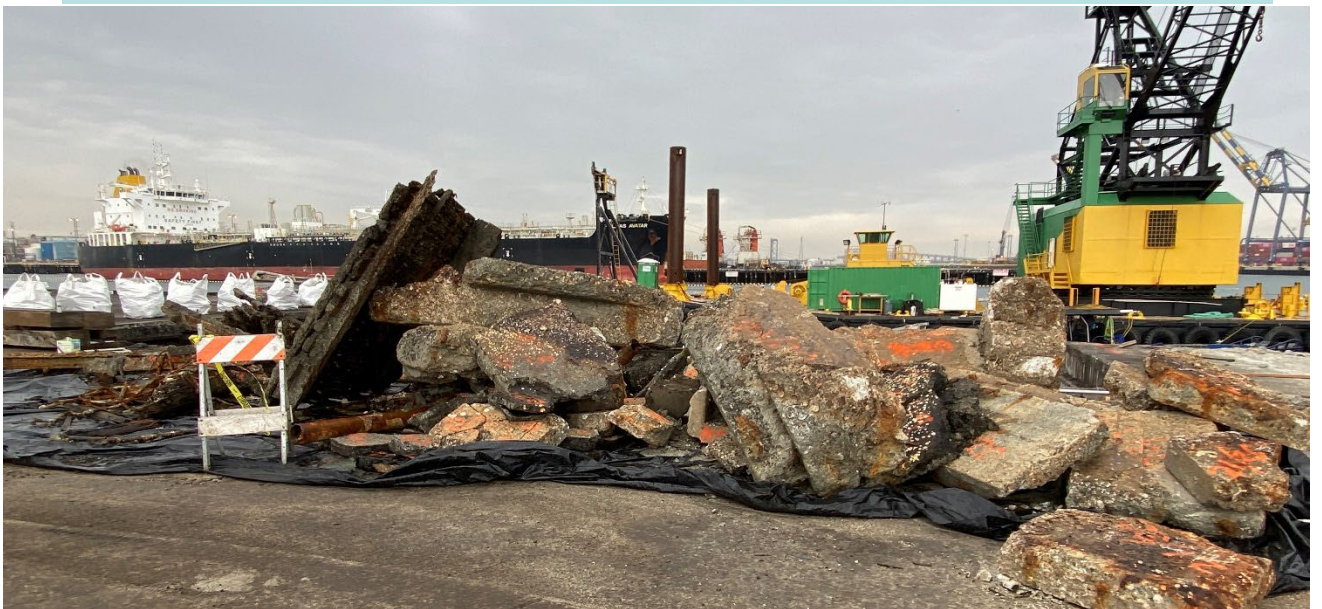
2/26/24 - Total Concrete & AC Debris Removal at Berth 178, Bents 19-23
