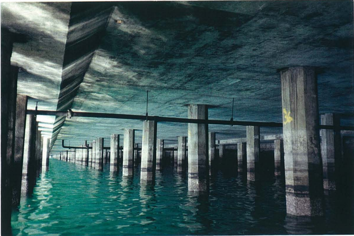
PHOTO 11-3. General view of 24 in. octagonal prestressed piles supporting concrete wharf.
