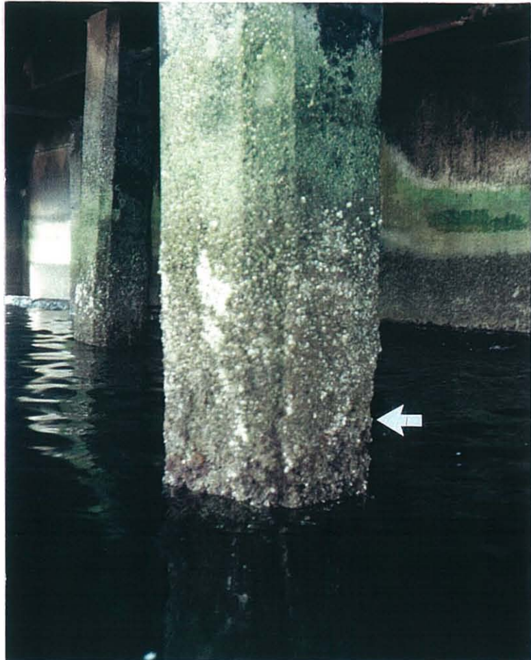
PHOTO 11-14. Built-up cast-in-place (CIP) section on concrete pile. Red arrow indicates typical crack location, while white arrow points to corrosion spall at CIP section.
