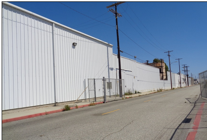
Figure 7: Cannery Block, west elevation, view from Cannery Street looking south down Ways Street, camera facing south. ICF, 2019
