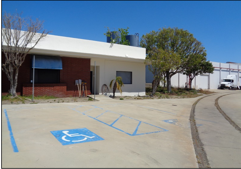
Figure 3: Cannery Block, open courtyard, and a railroad track spur line (foreground) with warehouse buildings (background), detail showing west elevation of office at the northeast portion of the Cannery Block, camera facing south. ICF, 2019.
