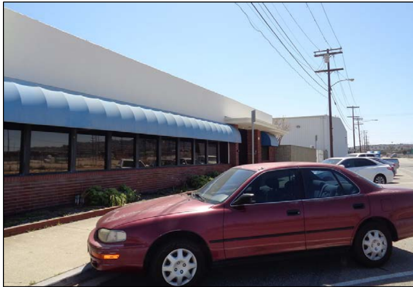
Figure 14: Cannery Block, north elevation, detail showing office building in foreground and warehouse in the background, camera facing west. ICF, 2019.
