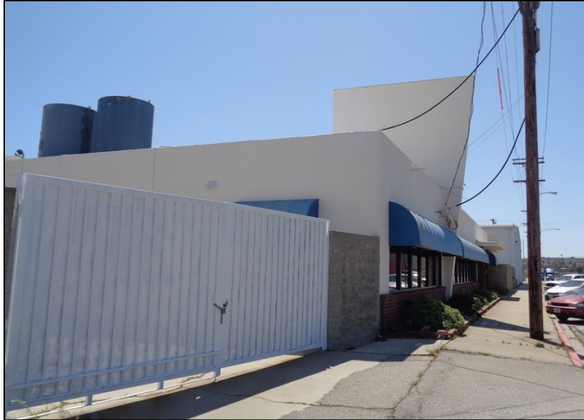
Figure 13: Cannery Block, north elevation, detail showing gate and office building in foreground and warehouse in background, camera facing west. ICF, 2019.
