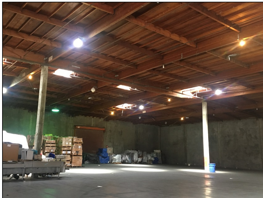
Figure 29: Cannery Block, c. 1960 warehouse interior, northeast portion of Cannery Block, camera facing north. ICF, 2019.
