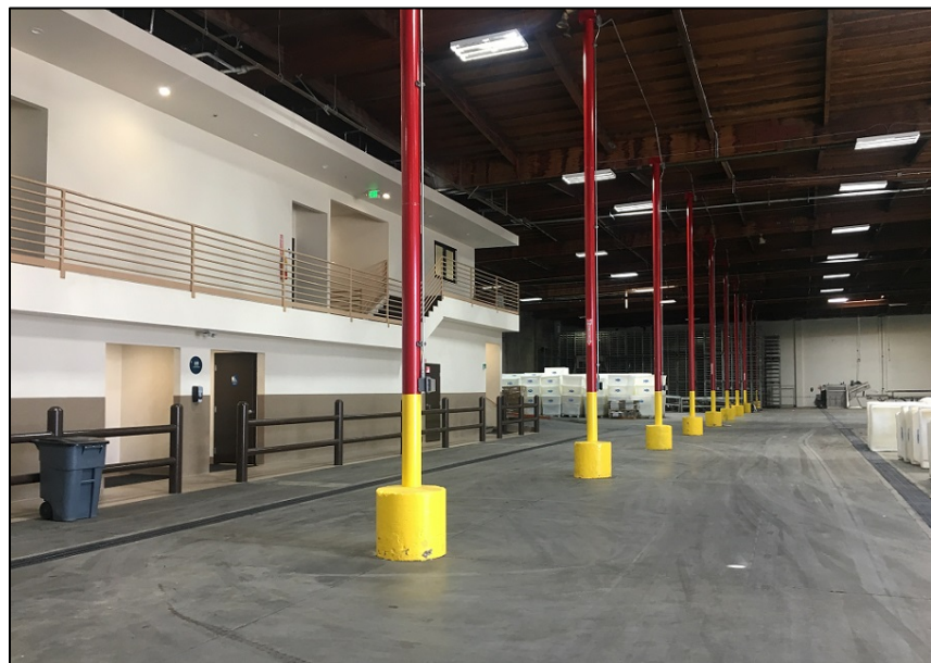
Figure 31: Cannery Block, 1972 warehouse interior, southeast portion of Cannery Block, camera facing south, detail showing interior office construction (left). ICF, 2019.
