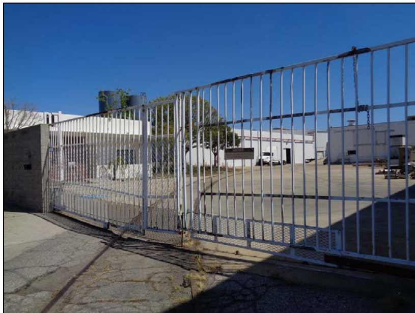
Figure 17: Cannery Block, north elevation, detail showing gate between office building to the east and warehouse to the west, camera facing southeast. ICF, 2019.
