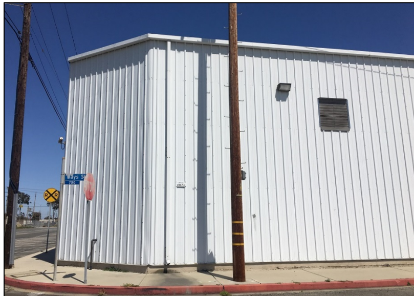
Figure 12: Cannery Block, west elevation, warehouse located at northern corner of west elevation, camera facing east. ICF, 2019
