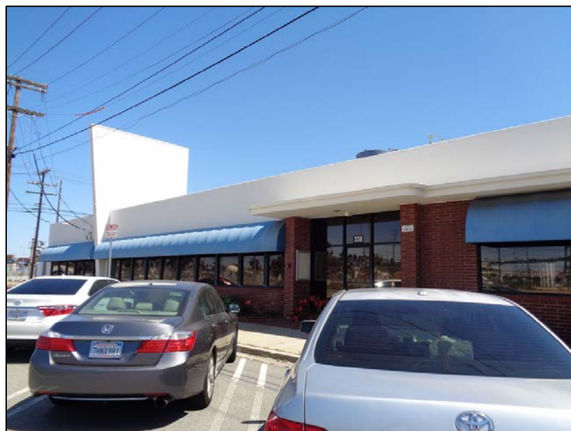
Figure 15: Cannery Block, north elevation, detail showing office building with signage pylon, camera facing southeast. ICF, 2019.
