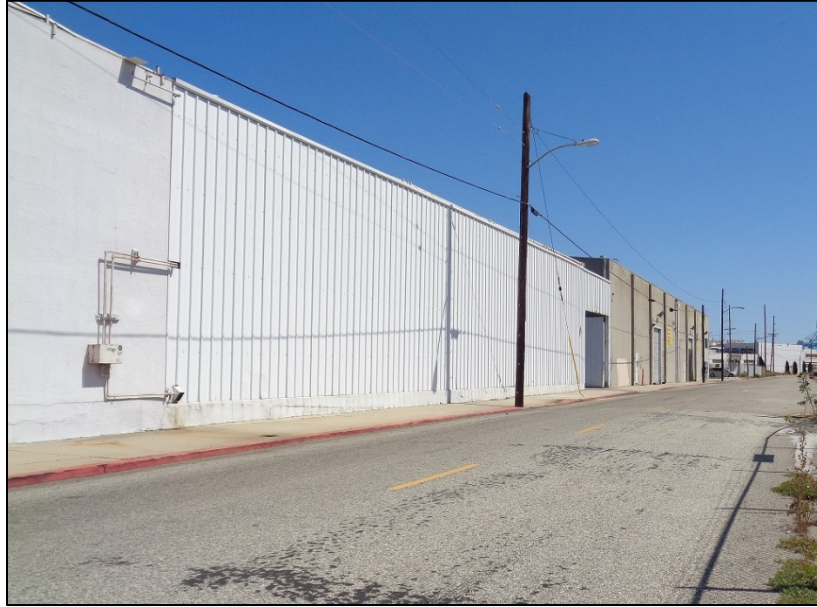
Figure 11: Cannery Block, west elevation, showing southern portion of elevation, camera facing south. ICF, 2019.
