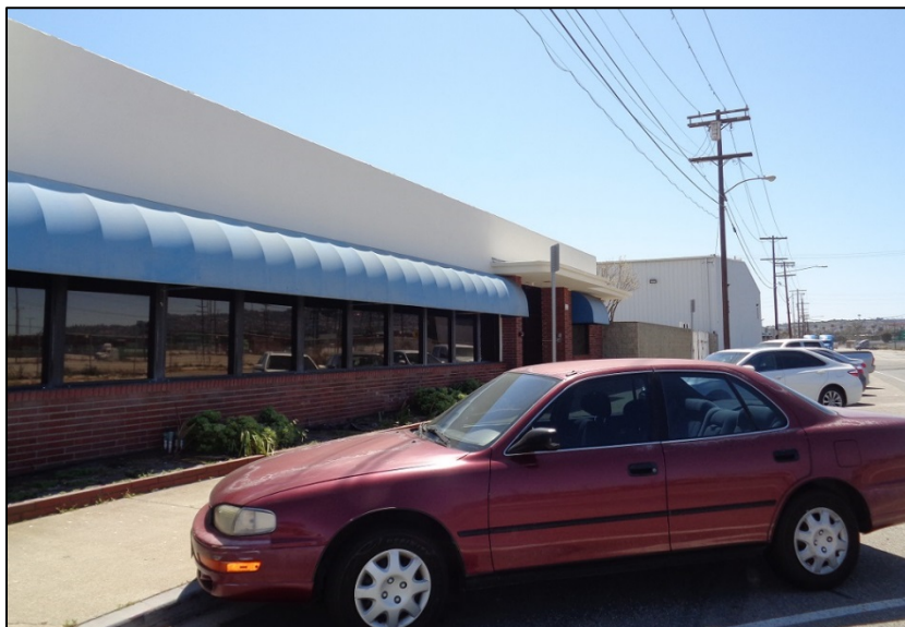
Figure 14: Cannery Block, north elevation, detail showing office building in foreground and warehouse in the background, camera facing west. ICF, 2019.
