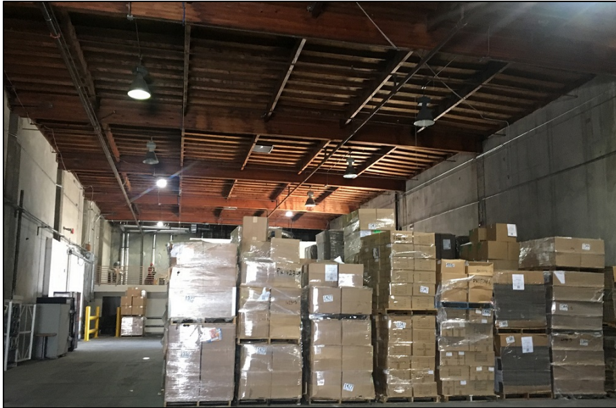
Figure 32: Cannery Block, 1972 warehouse interior, southwest portion of Cannery Block, camera facing south. ICF, 2019.
