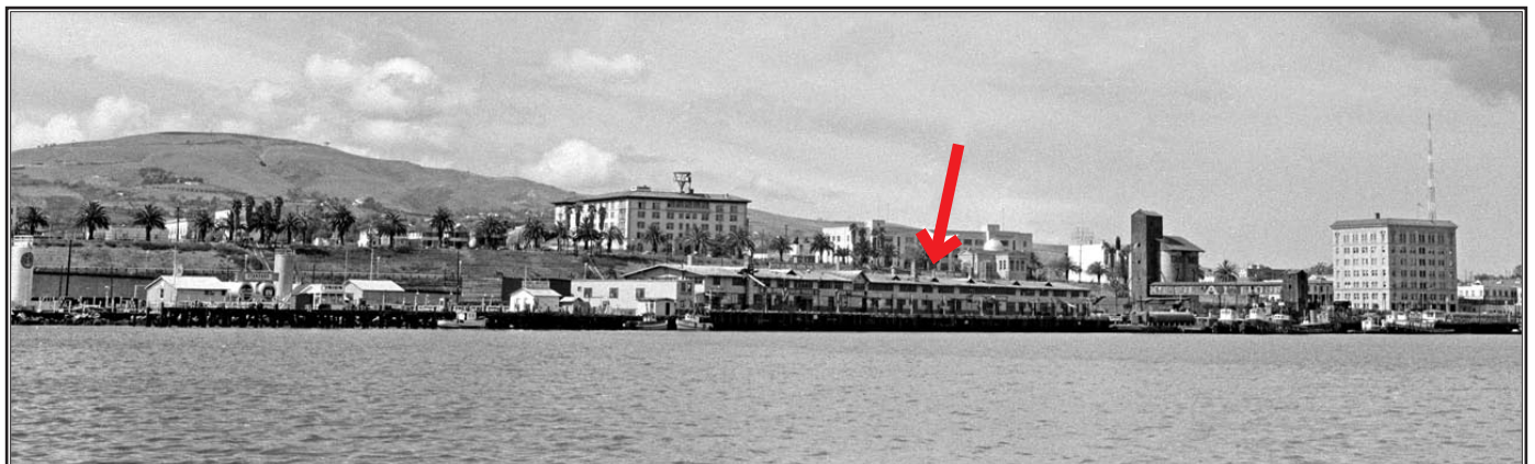
Main Channel and Municipal Fish Market, circa 1940 (Port of Los Angeles).
