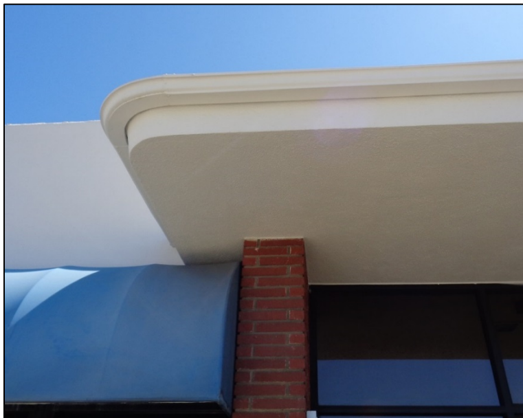
Figure 16: Cannery Block, north elevation, detail showing office building with curved cantilevered porch hood, camera facing west. ICF, 2019.
