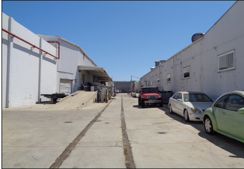
Figure 5: Cannery Block, driveway at a north-south axis, running south from open courtyard between two sets of warehouse buildings, camera facing south. ICF, 2019.
