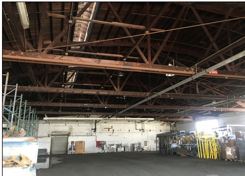
Figure 28: Cannery Block, 1950 warehouse interior, northwest portion of Cannery Block, camera facing southwest. ICF, 2019.
