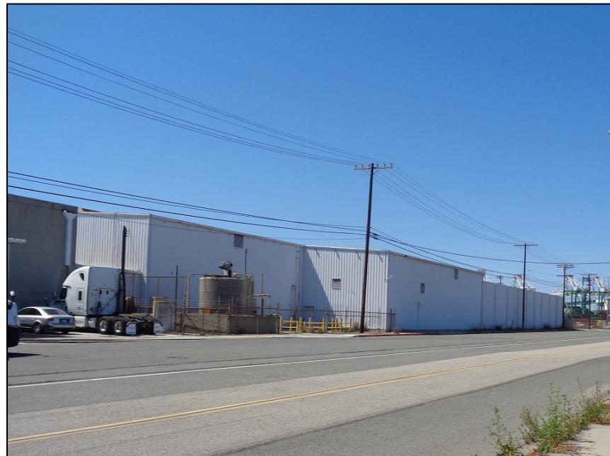
Figure 20: Cannery Block, east elevation with warehouses, showing northern portion of elevation, camera facing northwest. ICF, 2019.
