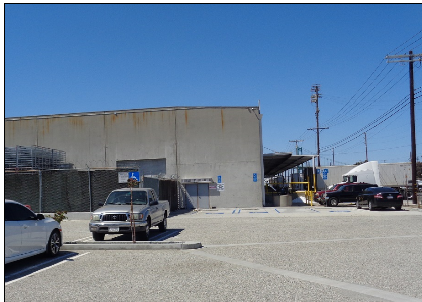
Figure 24: Cannery Block, south elevation, showing eastern corner of elevation, camera facing north. ICF, 2019.
